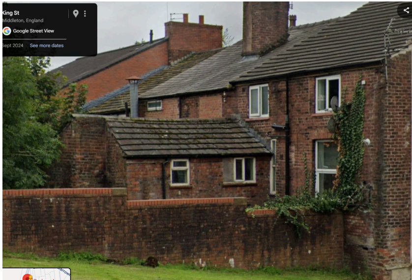
Google street view image showing the rear of no.76 Long Street and the brick wall on the shared site boundary.
