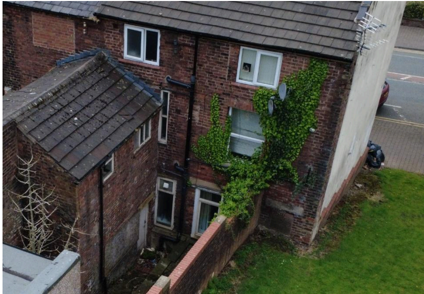
Drone image showing the lower ground floor window and the adjacent brick wall along the site boundary.
