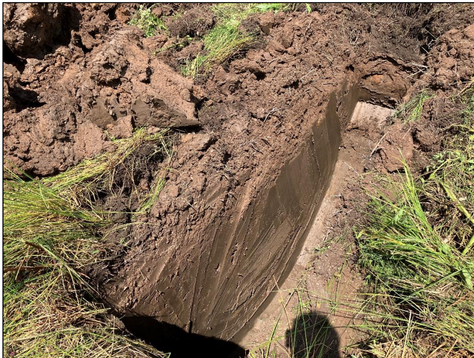
Photograph 37 – Photograph of TP13.
