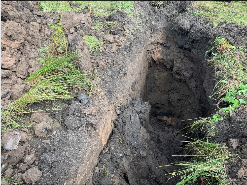
Photograph 27 – Photograph of TP10
