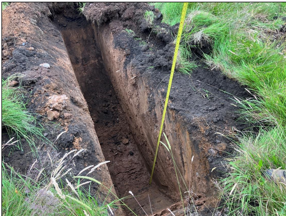
Photograph 4 – Photograph of TP02.
