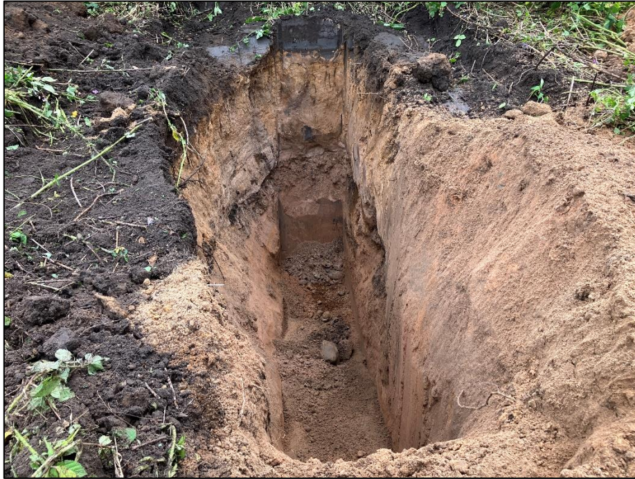
Photograph 44 – Photograph of TP15.
