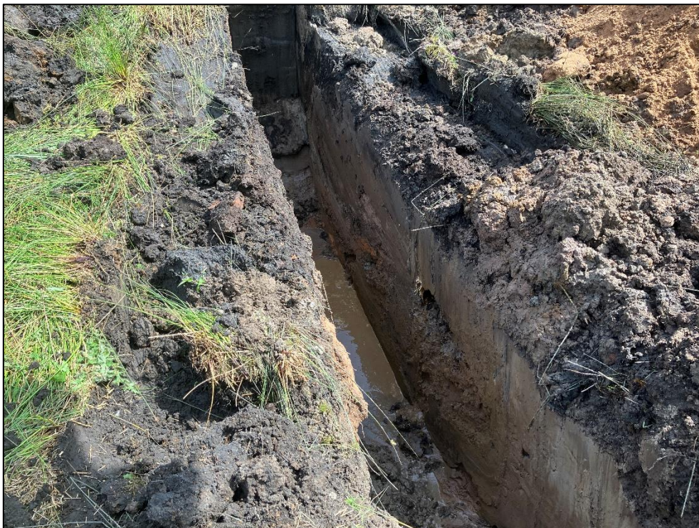
Photograph 49 – Photograph of TP17.
