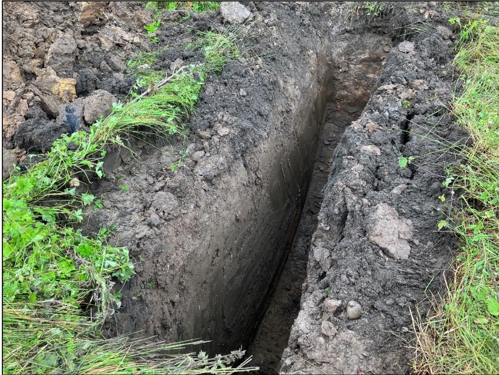
Photograph 19 – Photograph of TP07.
