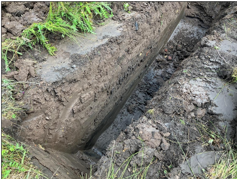
Photograph 41 – Photograph of TP14.
