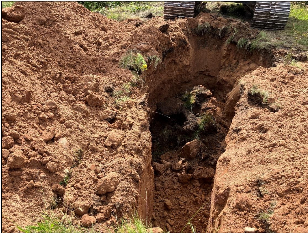
Photograph 46 – Photograph of TP16.
