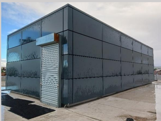
Photograph 23: Metal clad buildings on top of flat roofs.
