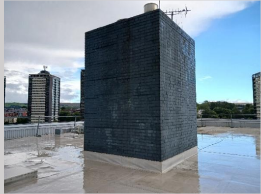
Photograph 20: Brick structure on roof of block B. Only accessible externally.
