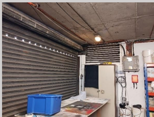
Photograph 26: Garages, potential access for bats.
