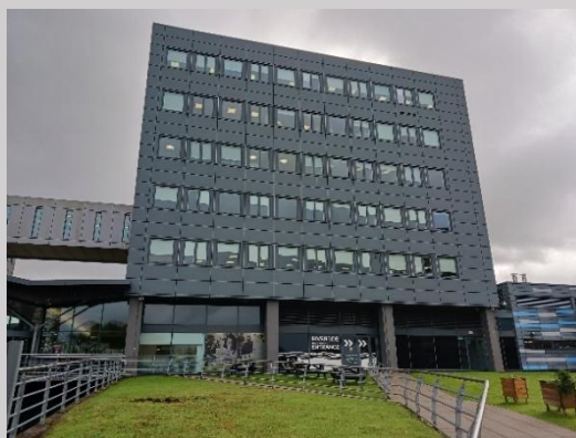
Photograph 4: Block A connected to block B.
