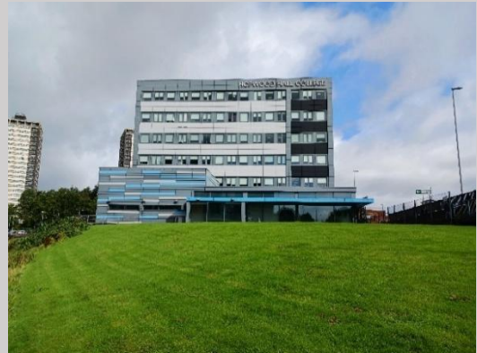
Photograph 14: Block A outside site boundary.
