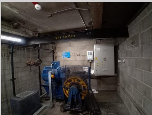
Photograph 17: Winch lift room on the roof of Block A.
