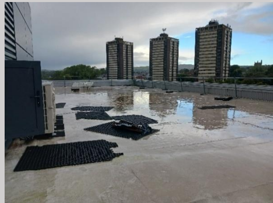
Photograph 10: Example of flat roof on site.
