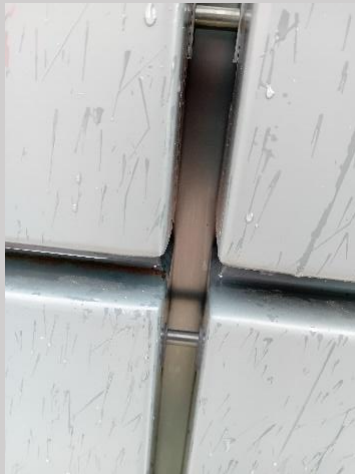
Photograph 15: External metal cladding, block A and block B.
