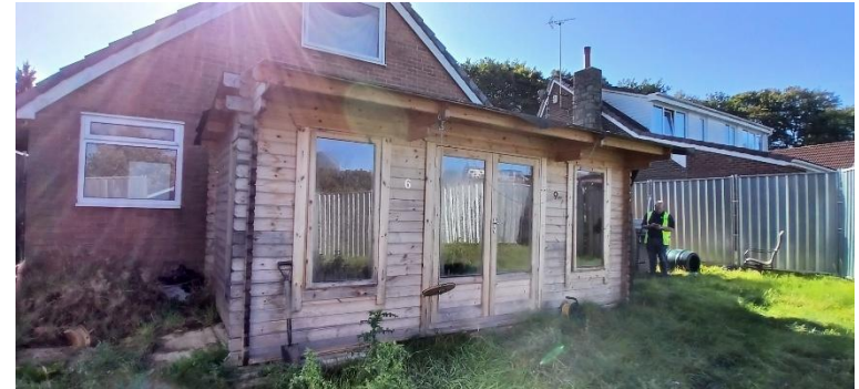
Adjoining wooden panel structure to rear of B1
