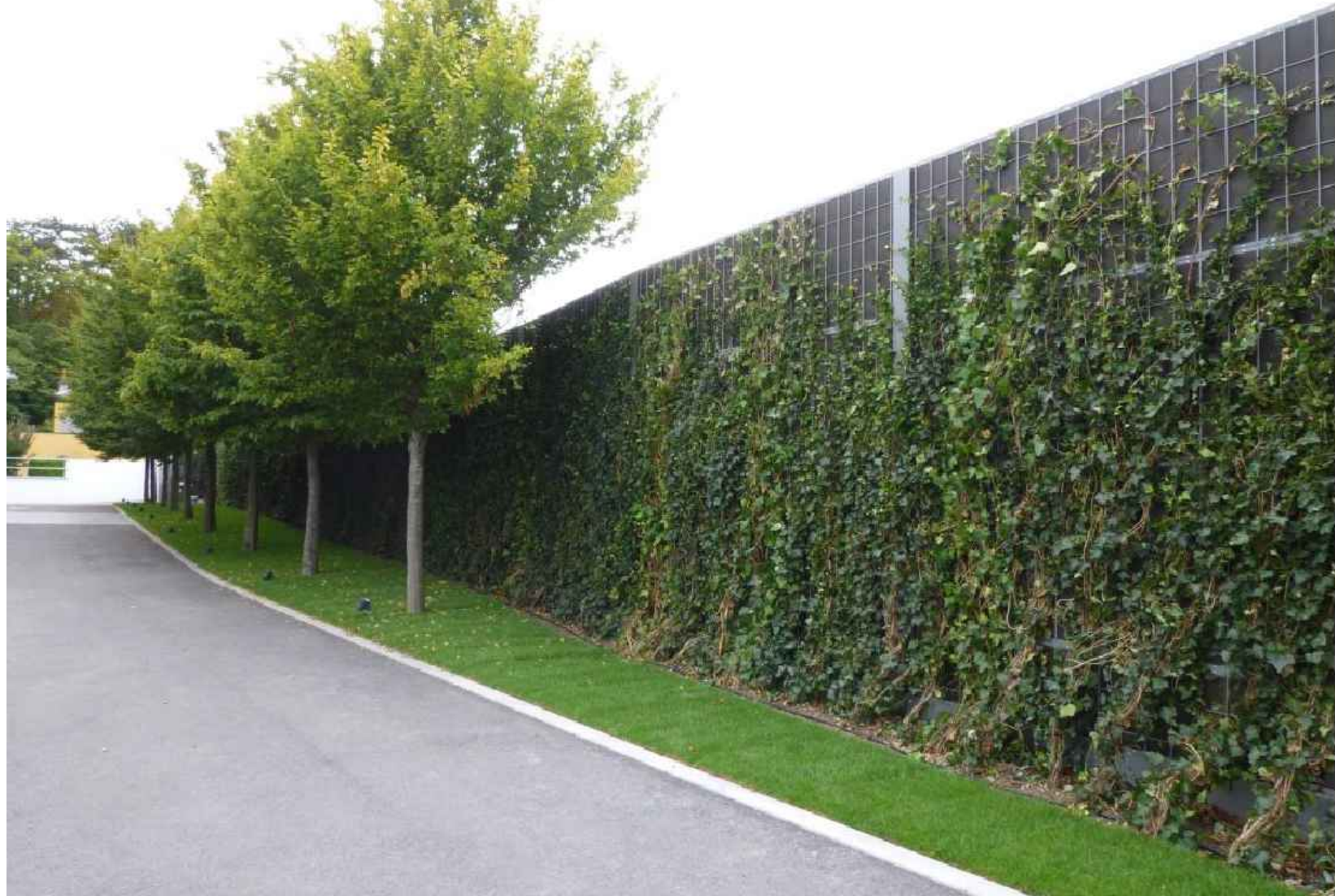
Proposed Acoustic Fence Type 3 & 4 Sample picture of Gramm Barrier System GREENSoundBlok (www.grammbarriers.com)
