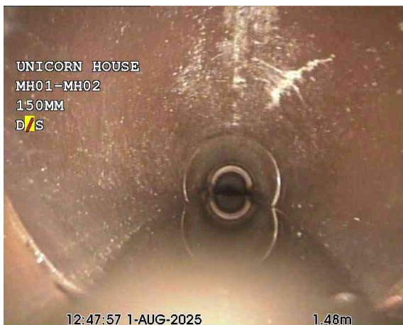
MH01_4f80a8fa-e08b-4d76-933b-8cce79fe3443_20250807_1 10951_577.jpg, 00:00:22, 1.48 m Water level, 20% of the vertical dimension
