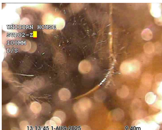
SVP02_34a6ac0c-34bb-4ce6-a6cf-01257af3c8d2_20250811_101025_819.jpg, 00:01:43, 9.40 m Roots, fine at joint
