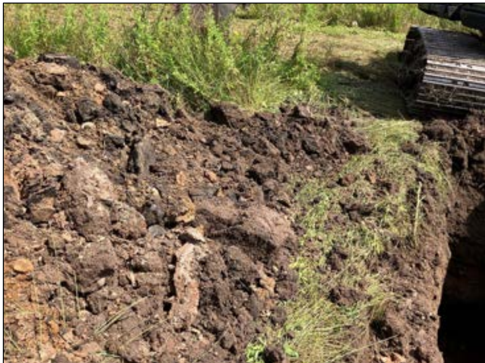
Photograph 47 – Photograph of Topsoil encountered in TP16..
