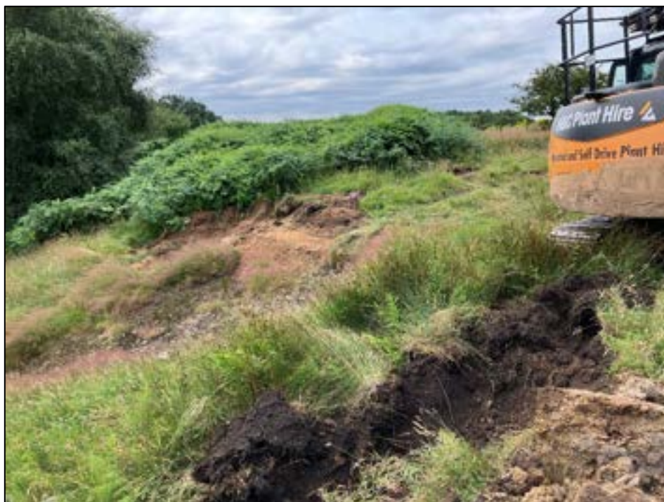
Photograph 67 – Photograph of TP24, with TP23 in the background.
