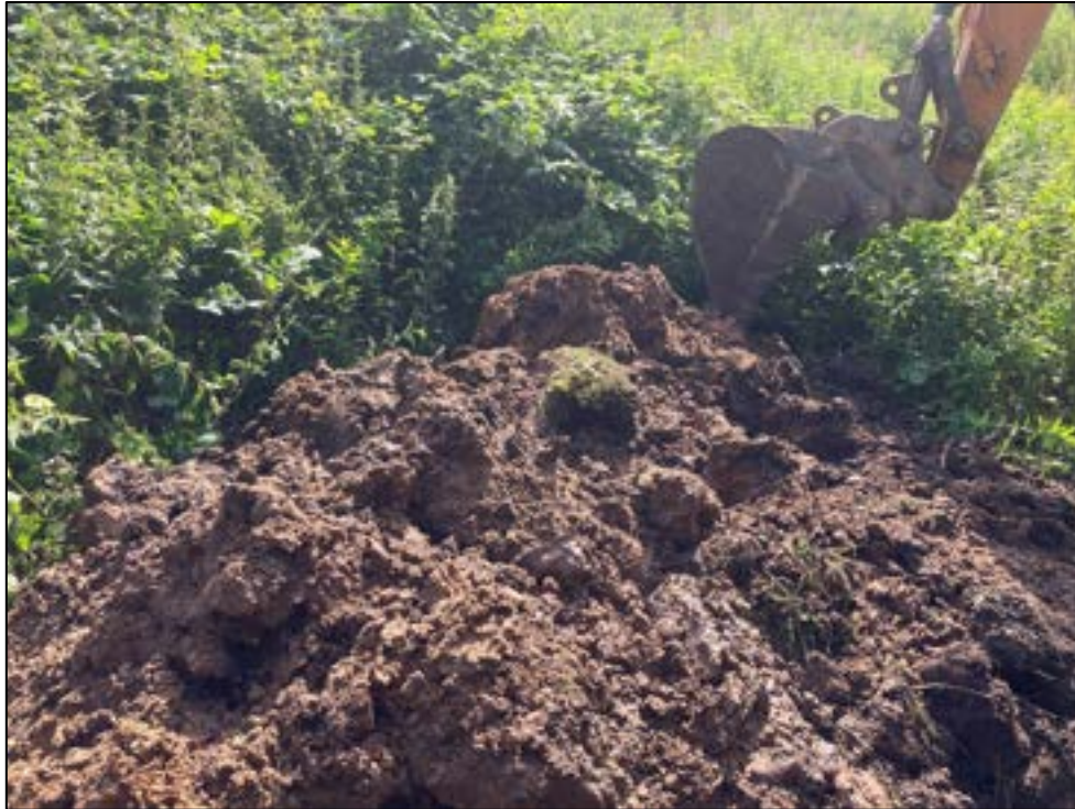
Photograph 58 – Photograph of Made Ground encountered in TP20.
