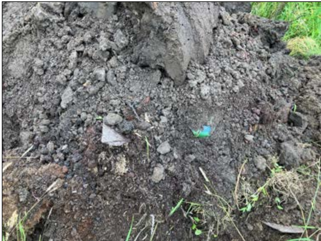
Photograph 8 – Photograph of the Made Ground encountered in TP03.
