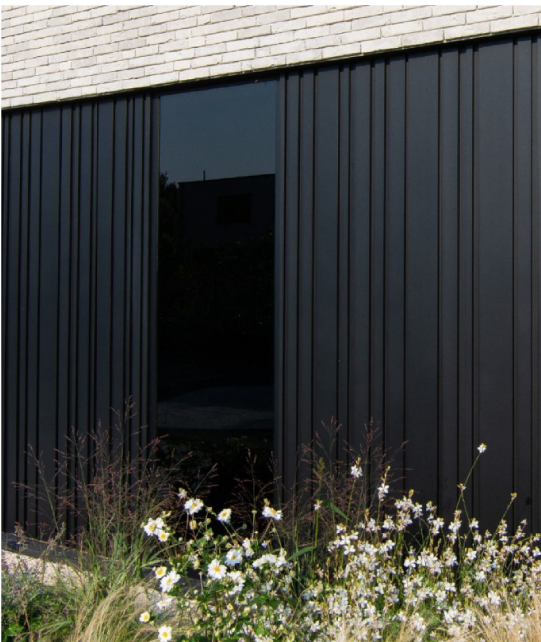
Example of stained larch timber cladding
