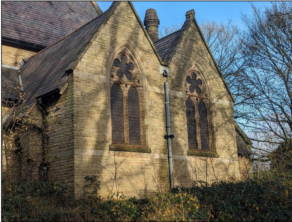
Plate 5: East end of south elevation
