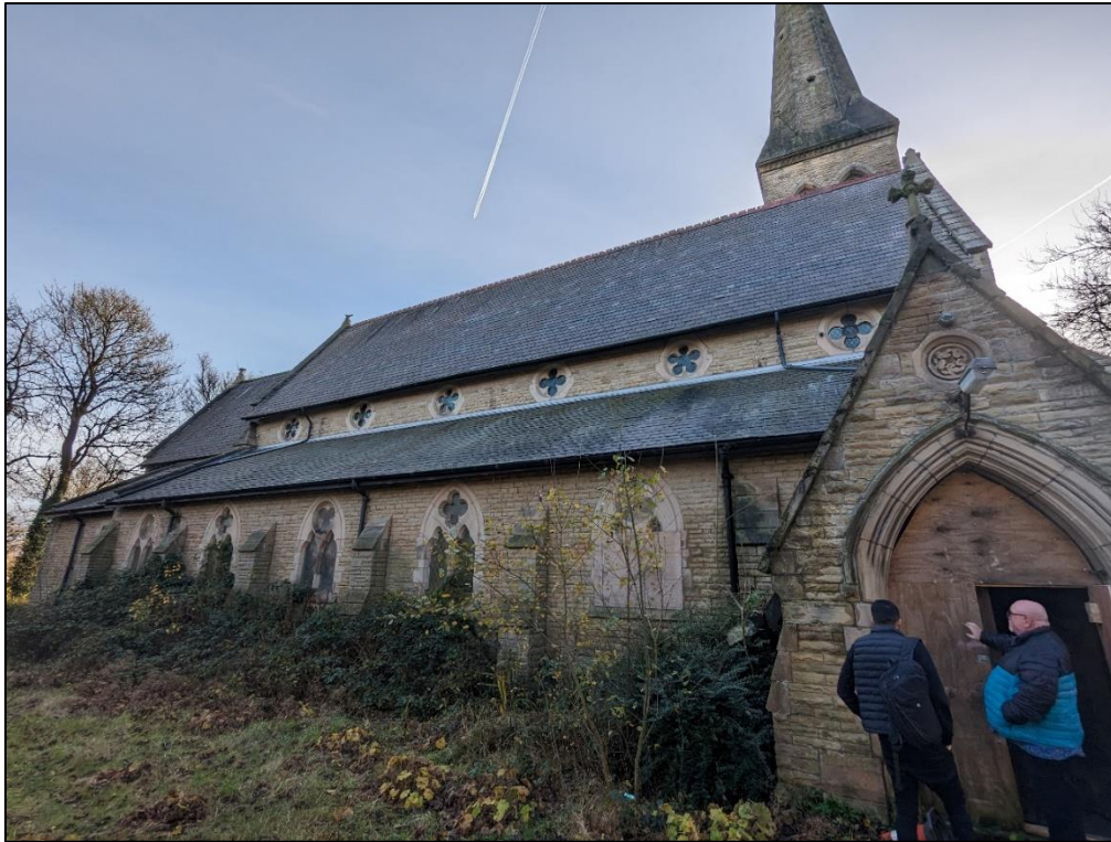
Plate 1: North elevation of church
