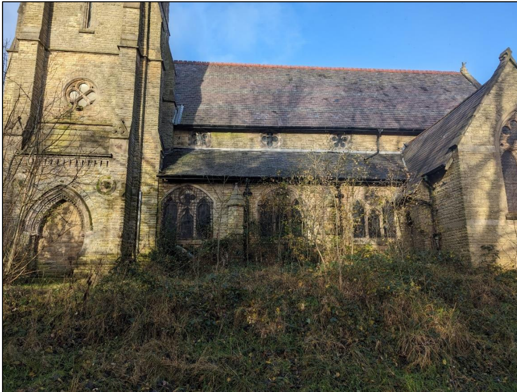
Plate 3: South elevation of church
