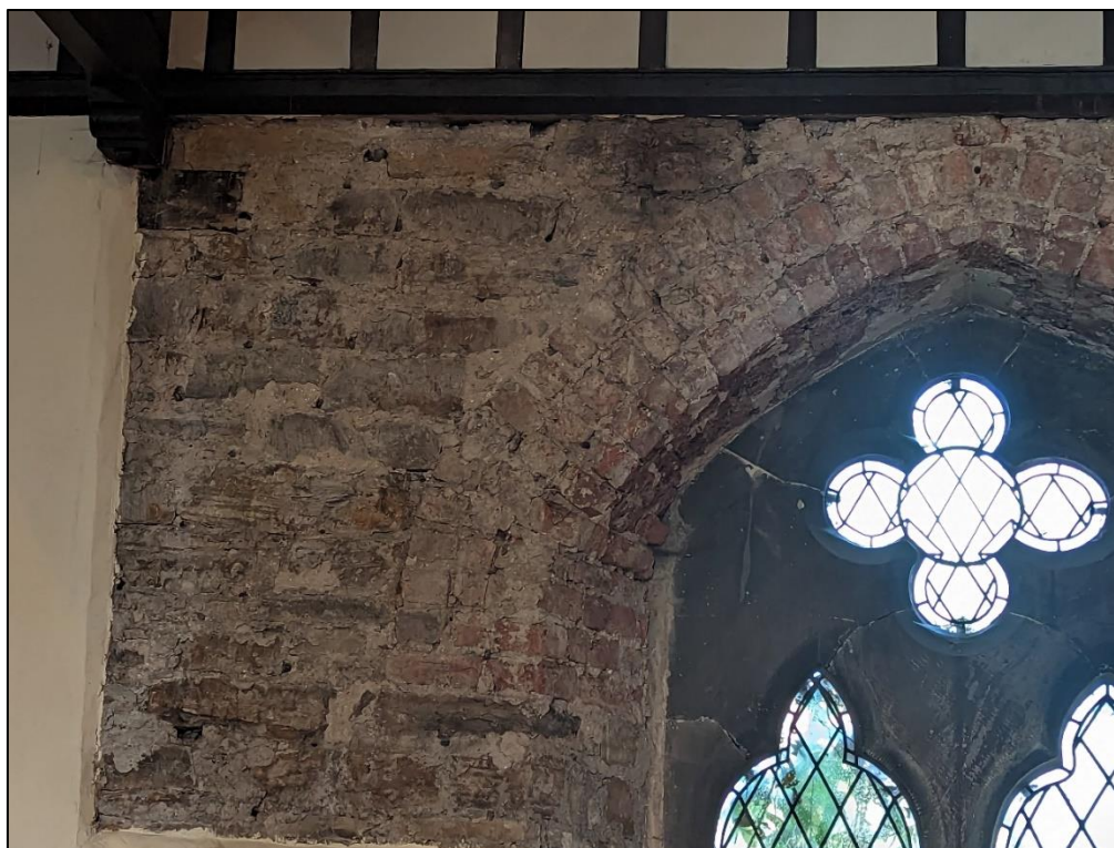
Plate 28: Detail of sandstone walling with brick built lintel
