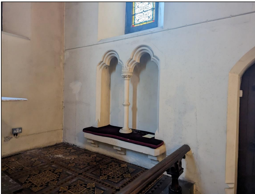
Plate 24: Arched recess for Sedilia in south chancel wall
