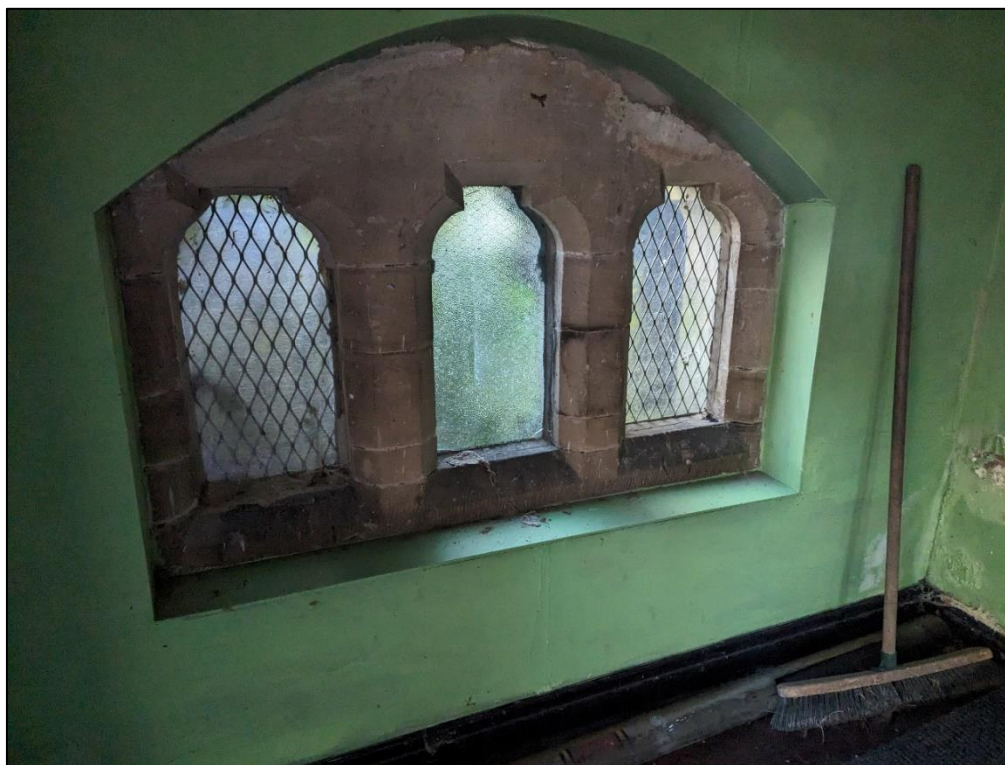
Plate 12: Porch window detail
