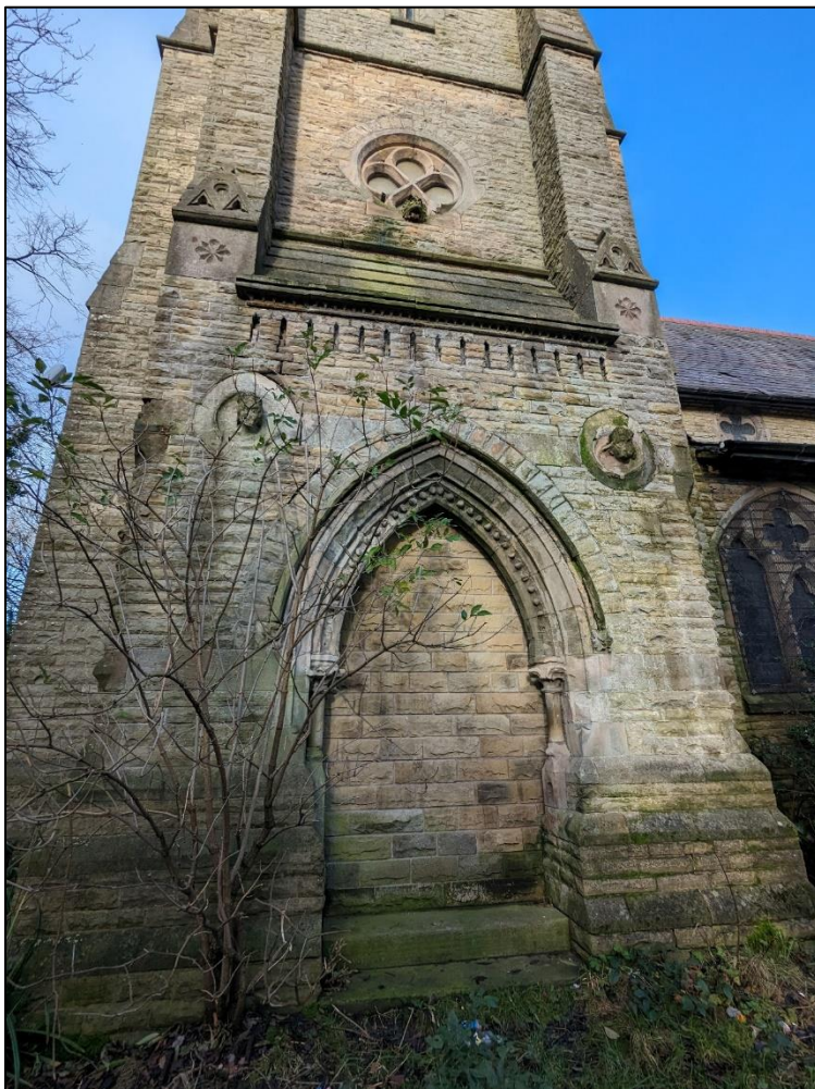
Plate 2: Blocked doorway in south elevation of church
