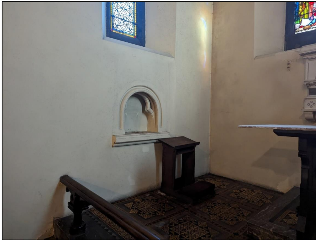
Plate 25: Credence niche to north chancel wall
