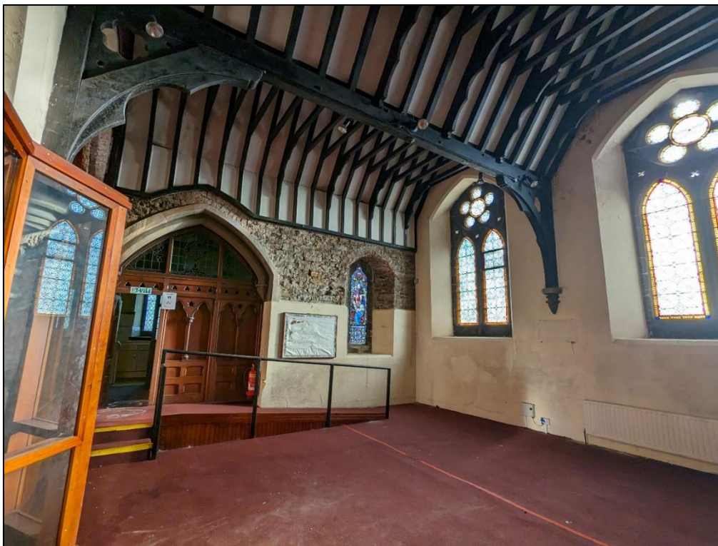
Plate 32: Timber panelling to opening to south transept
