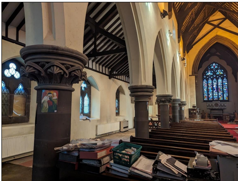
Plate 30: Columns to northern aisle
