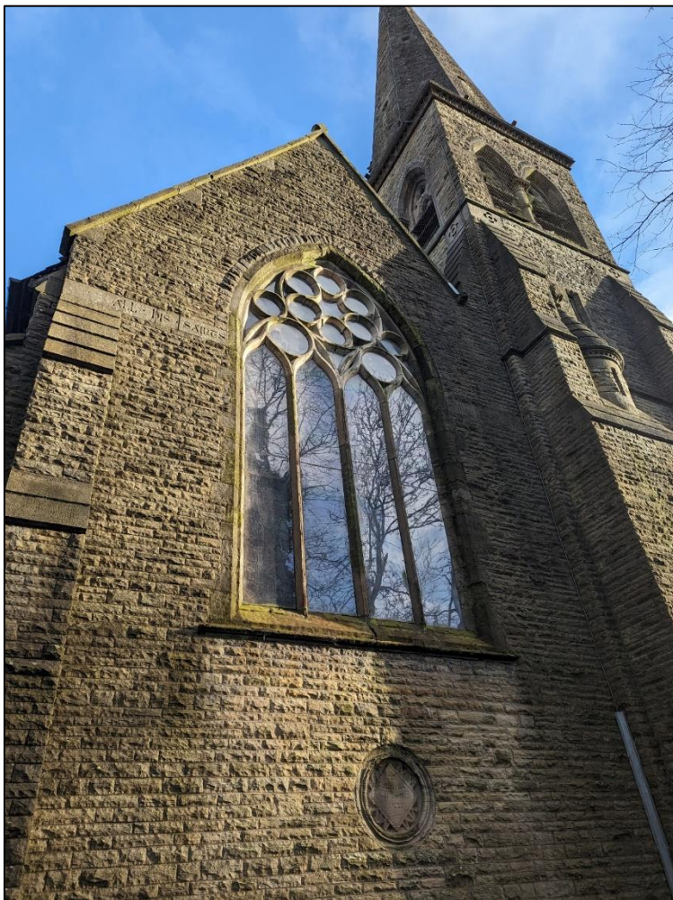
Plate 6: Large stained glass window in west elevation, covered with perspex
