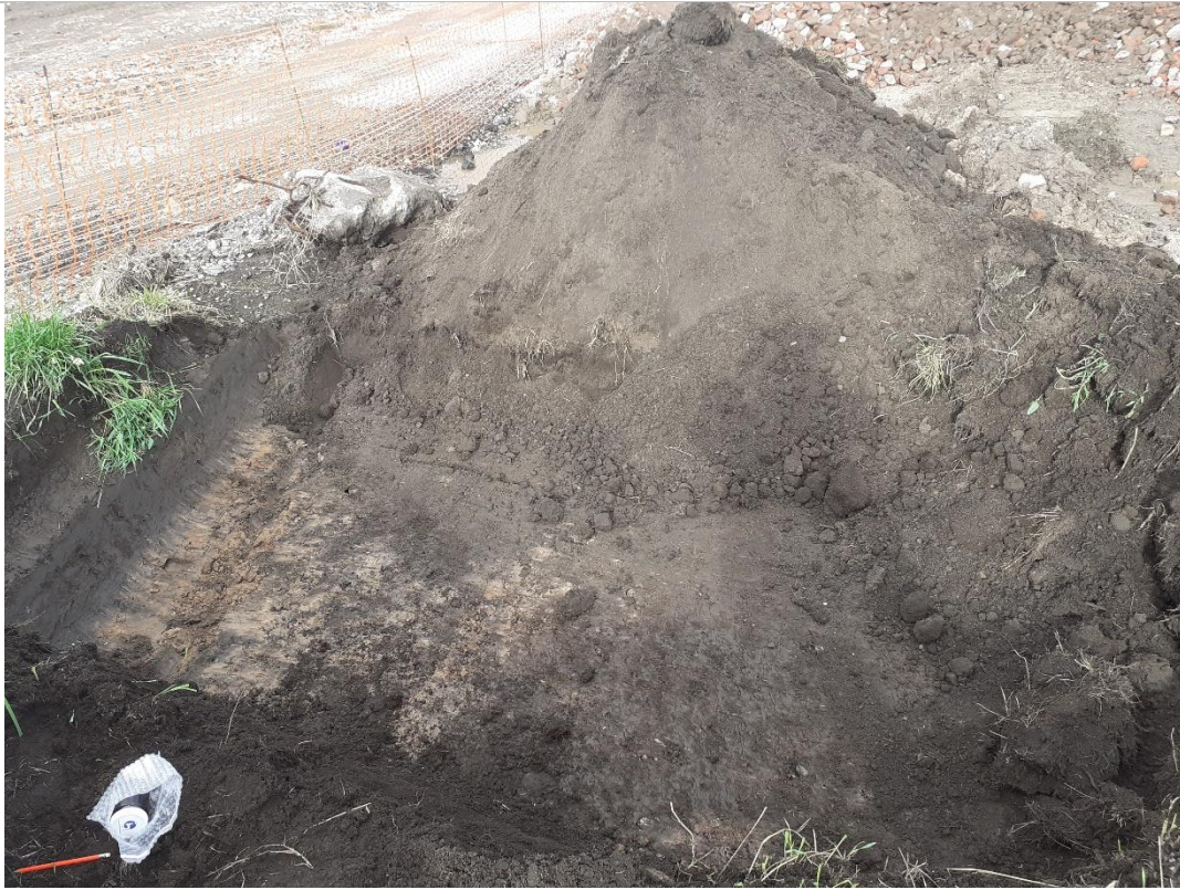
PLATE 1 TP126 HOTSPOT EXCAVATION
