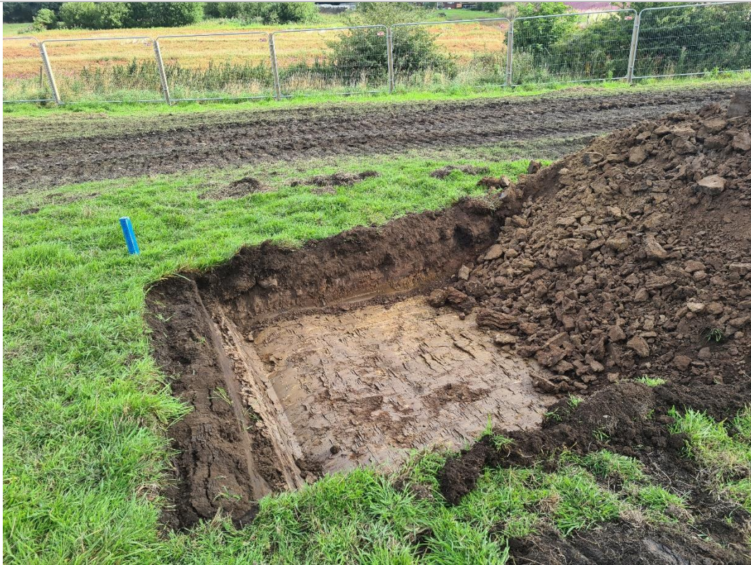
PLATE 2 TP120 HOTSPOT EXCAVATION
