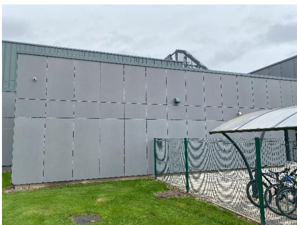
Photo 7: Existing school building
