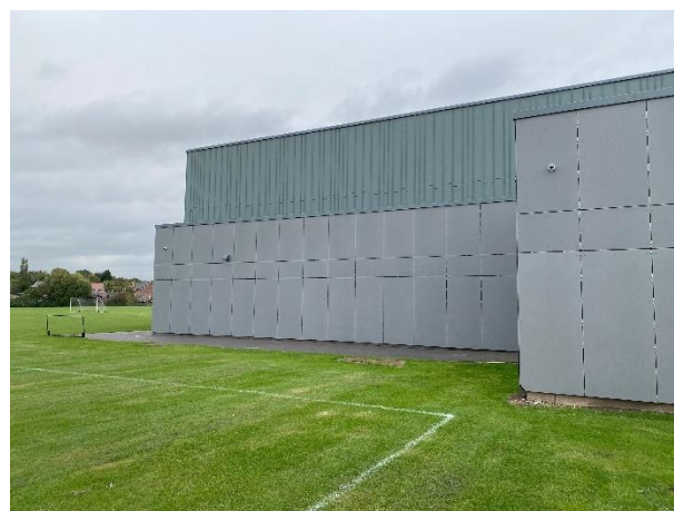
Photo 8: Existing school building
