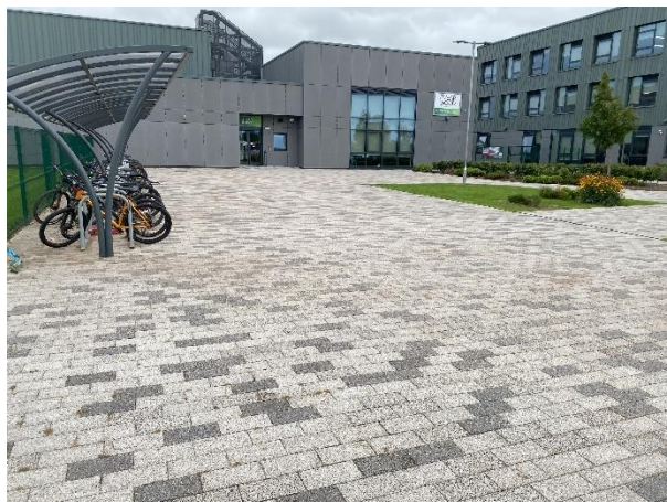
Photo 1: Hardstanding with modified grassland and existing school building
