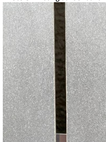
Photo 10: Gap between panels at existing school building with dense insulation behind
