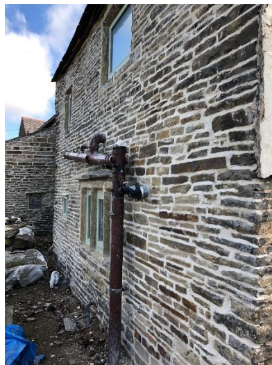
Picture 5. Image of the completed restoration work.
