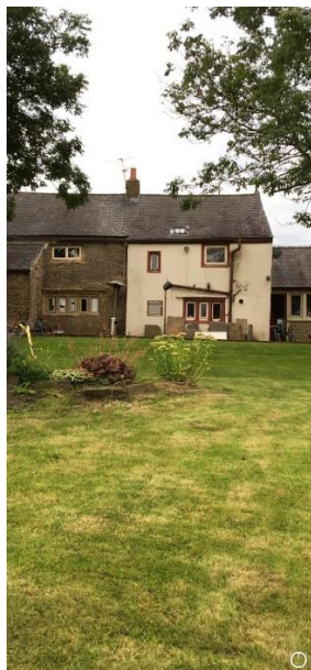
Picture 1. Image of part of the rear elevation with render applied
