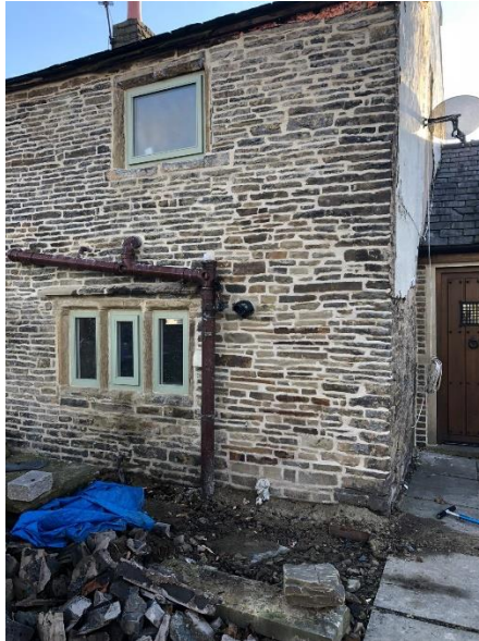
Picture 7. Image of the completed restoration work.
