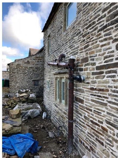
Picture 6. Image of the completed restoration work.
