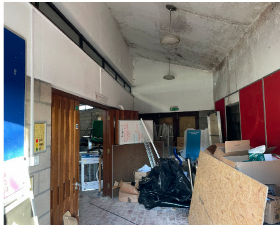
5 View into the entrance lobby.
