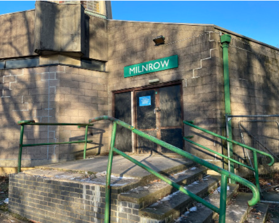
6 Steps into one of two mirroring main entrances.
