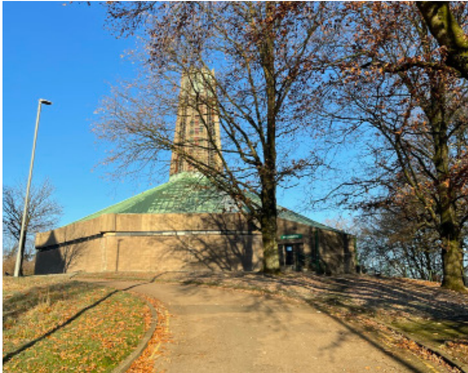
7 View from approach via existing road to the South.
