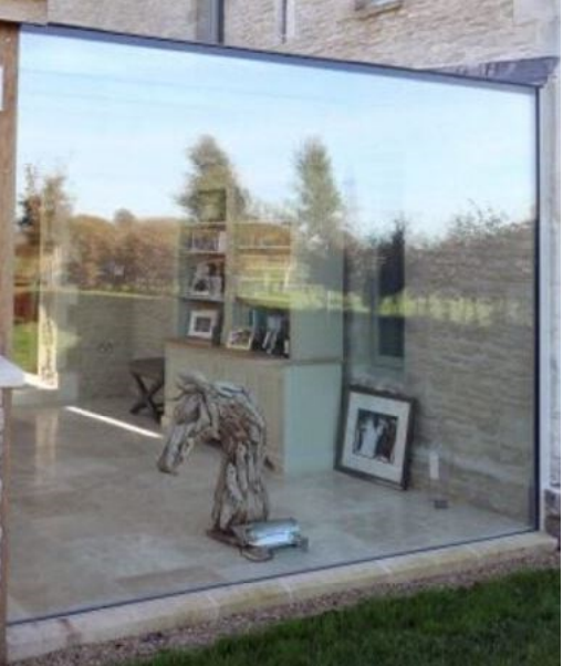
Condition 7 - Glass link image
