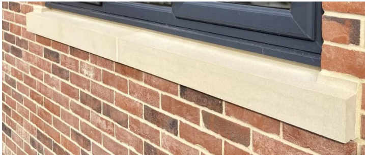
Cast Stone window heads and cills.
