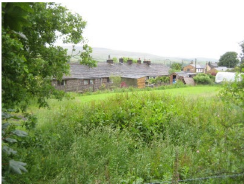
Figure 14: View of the rear of 9-19 Salley Street
