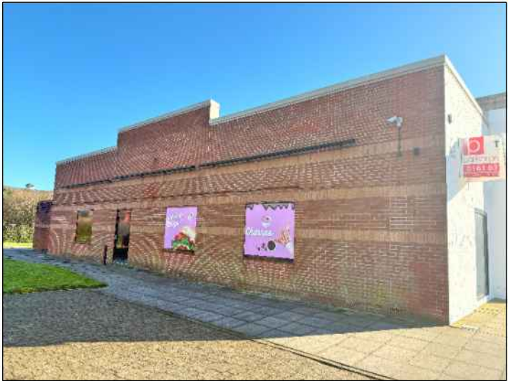
03 View from the side elavtion - North-west
