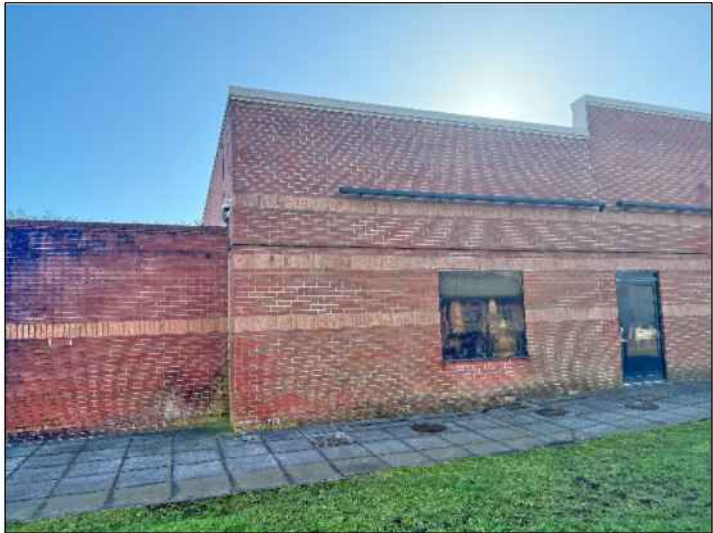
04 View from the side elavtion - North-west
