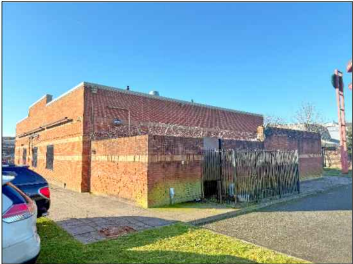
05 View from the side elavtion - North-east
