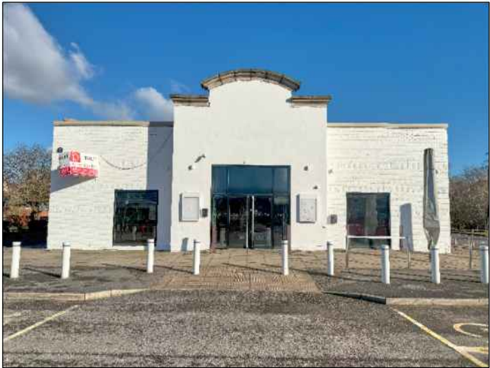
02 View of the front elevation - South-west
