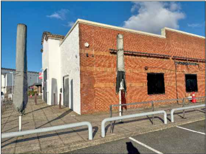
01 View from the side elevation - South-east
