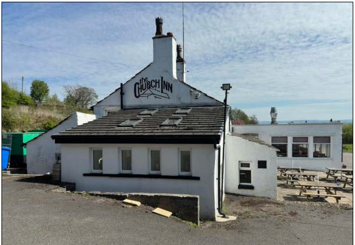
Outshuts to front side and rear of the first bay are early 19 th century and early-mid 20 th century
