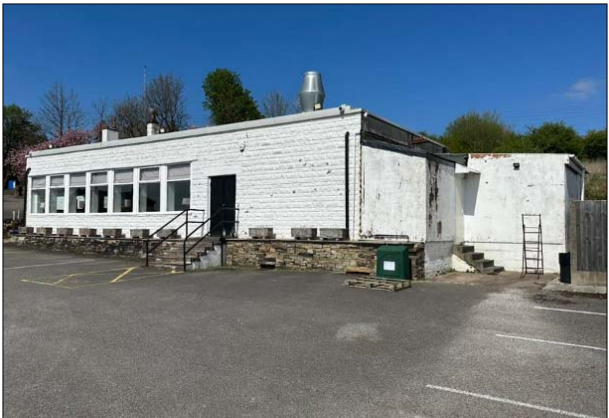
The large probably 1970s dining room extension that masks much of the original building
