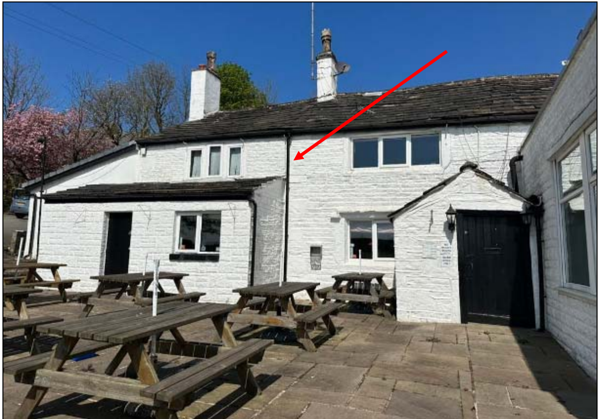
Front elevation showing quoins marking end of the earliest phase of the 17 th century house, the two-storey bay to its left is an addition also of the 17 th century
