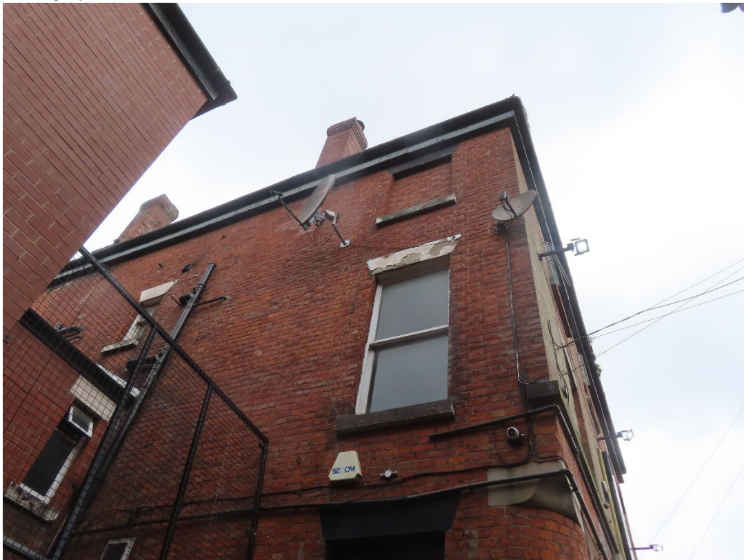
Open up built up window opening at the first floor and second floor level.
