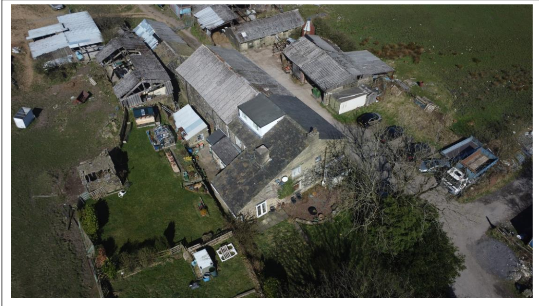
Lower Cleggswood Farm (houses and stone barn), Littleborough
