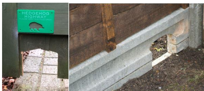
Insert 4: Showing wildlife access gap within fencing
