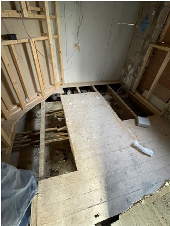
Photo showing Suspended Timber Floor
