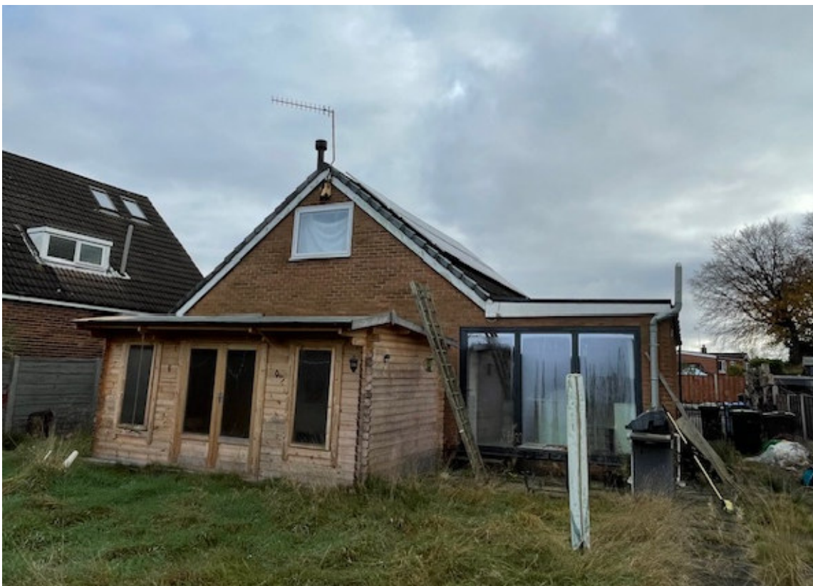
The rear elevation of the property.
