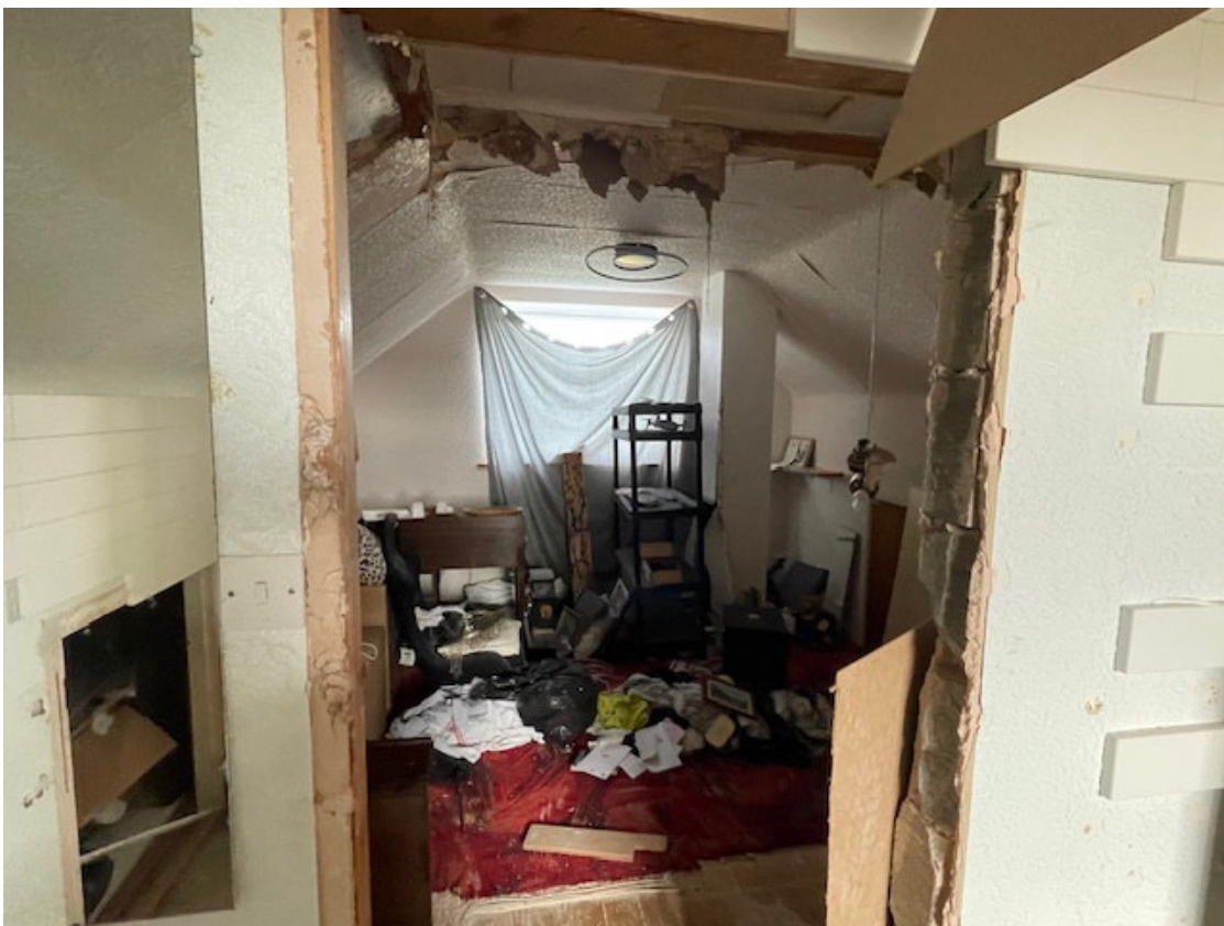
Existing Loft Floor
