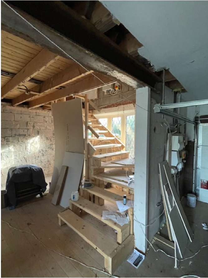
Timber Staircase to Loft Floor.
