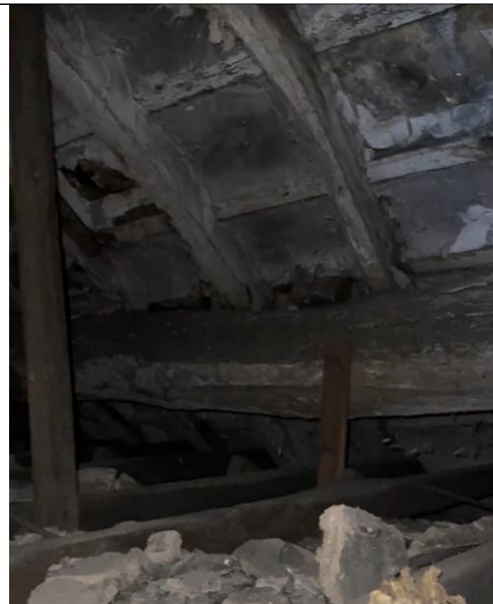
B1 Loft: Loft void – unlined roof with timber rafters and ridge beam.
