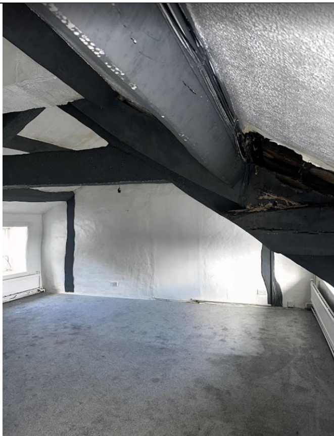
B1 Loft: Vaulted ceiling – internal view showing exposed beams.
