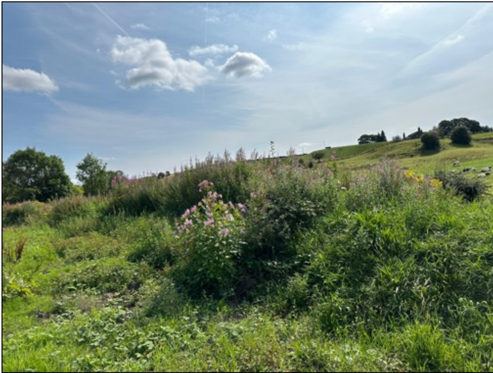
Photograph 4; A view of the rear of the eastern bund.
