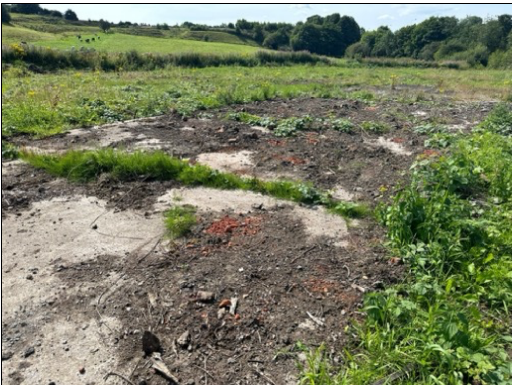
Photograph 12; Some sections of concrete foundations feature across the site.
