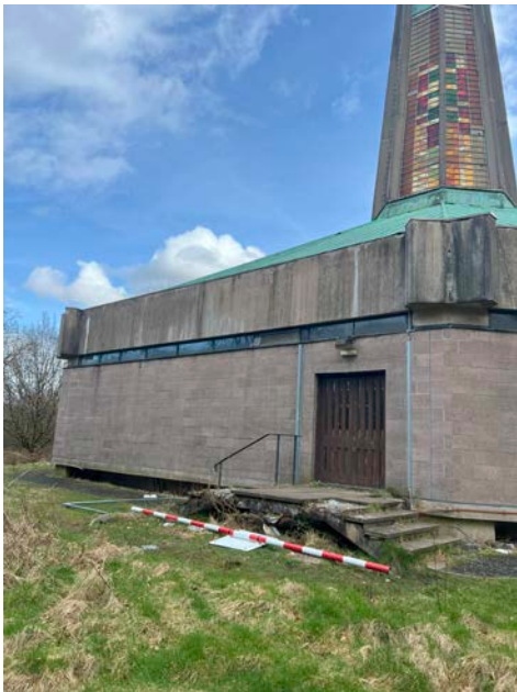
Rear steps to be retained and repaired
