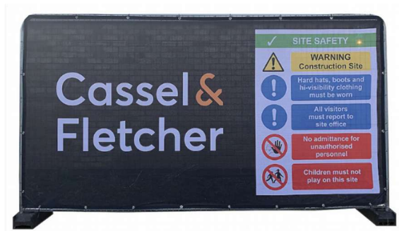
Figure 1 - Heras fencing with mesh protection
