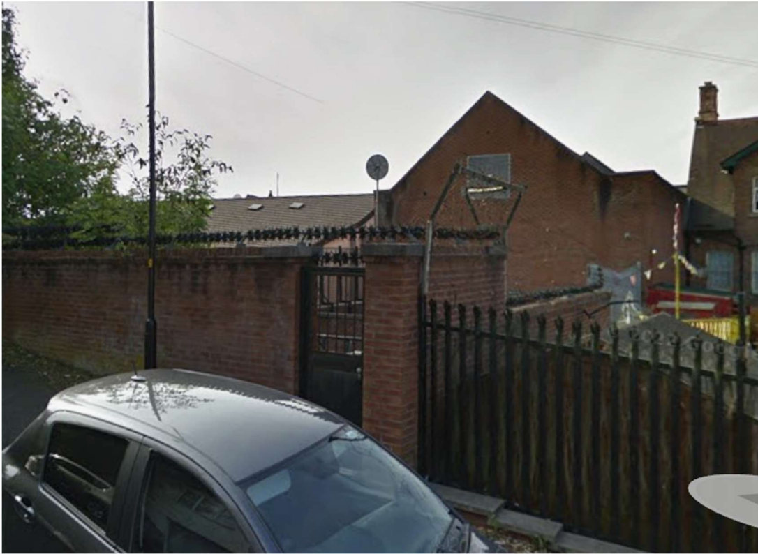
Fig. 2: Rear Elevation of the building and yard area.
