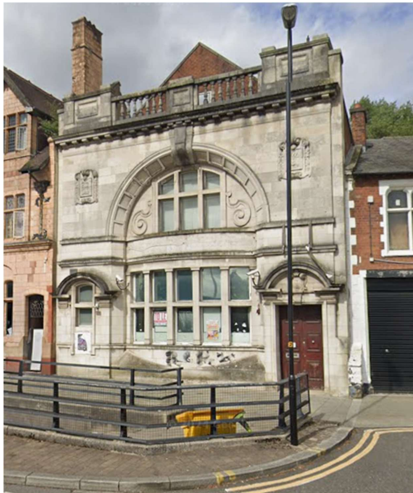
Fig. 1: Front Elevation of the building.
