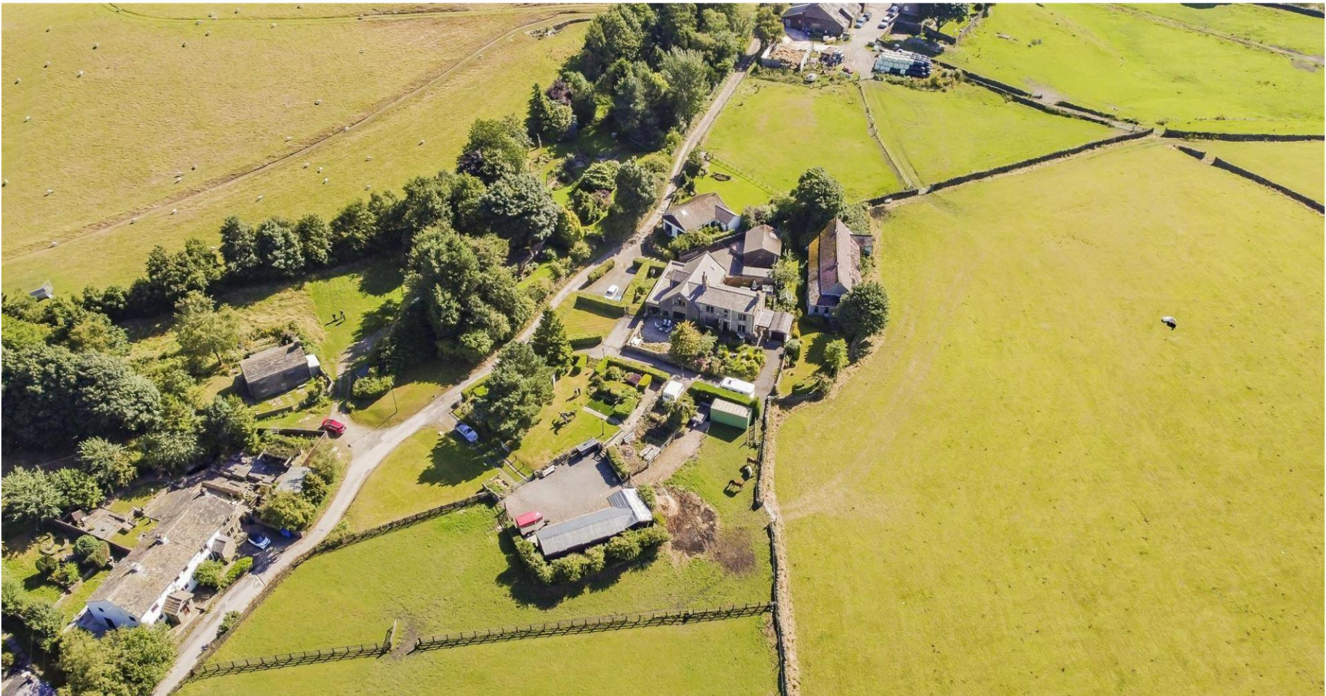
View 7 - Drone view of proposed site facing northeast.
