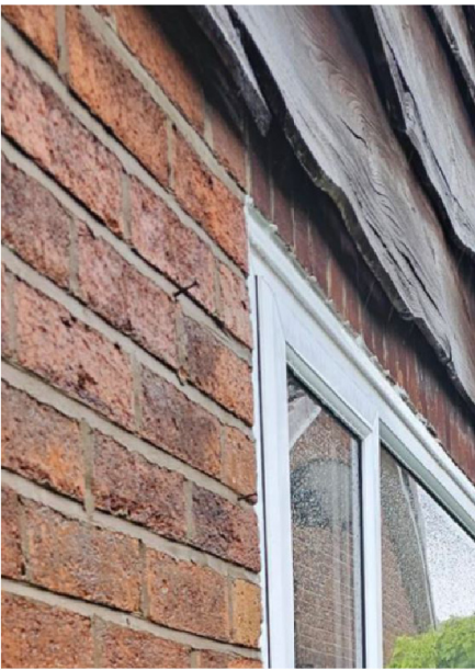
PHOTO OF PROJECTING CLADDING SMM PROPOSED RENDER WILL SIT BACK FROM THIS.
