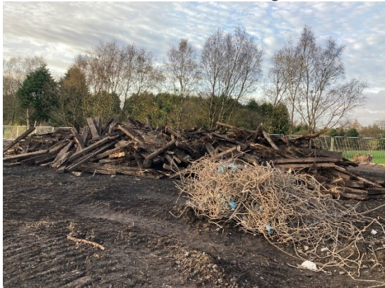
Plate 5 Stockpile Containing Visible ACM Fragments Awaiting Handpicking
