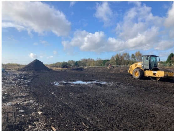
Plate 24 Placement of Made Ground
