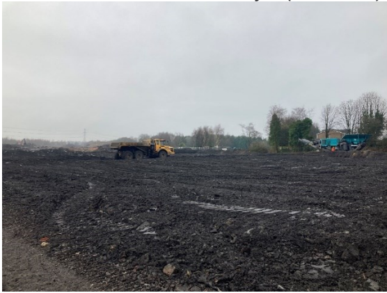
Plate 23 Placement of Pile Mat
