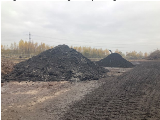
Plate 5 Stockpile Containing Visible ACM Fragments Awaiting Handpicking
