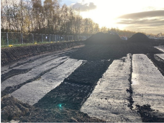
Plate 21 Placement of Final Layer (Formation)
