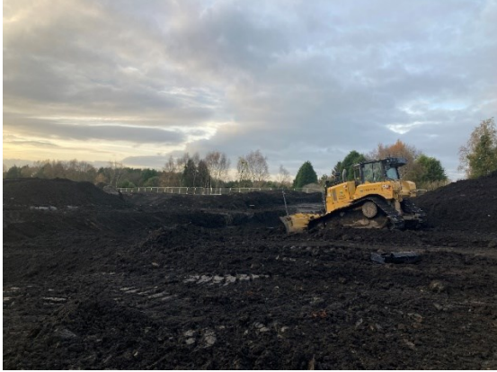
Plate 25 Replacement of Made Ground
