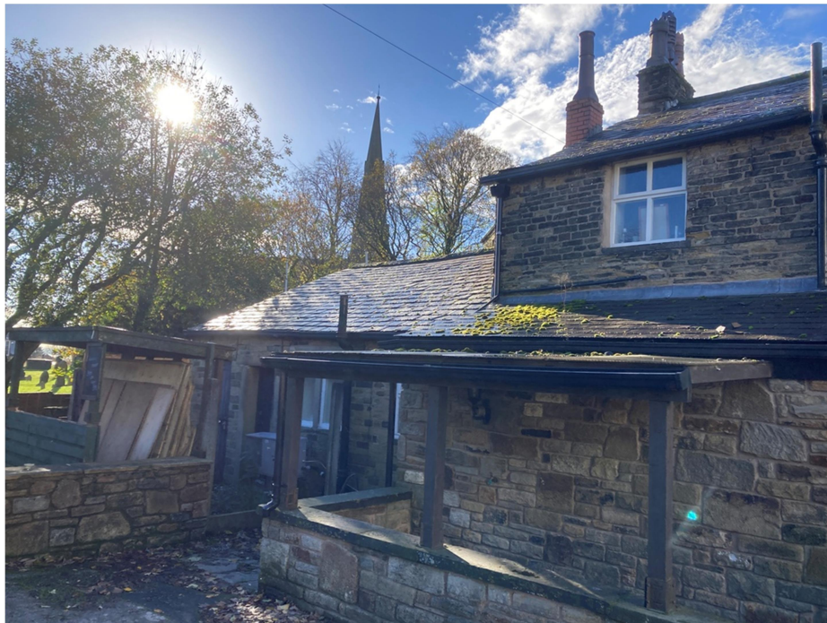
Image 2. Rear View of the property
