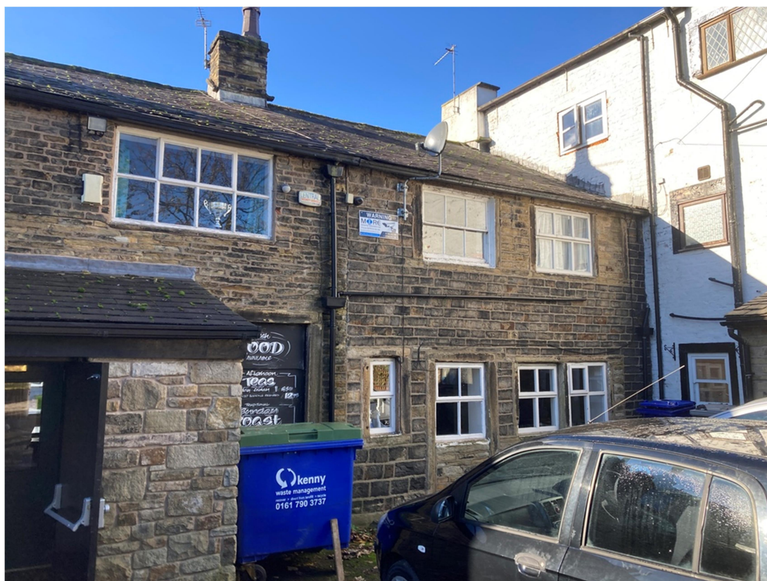
Image 3. Rear Elevation View of the property
