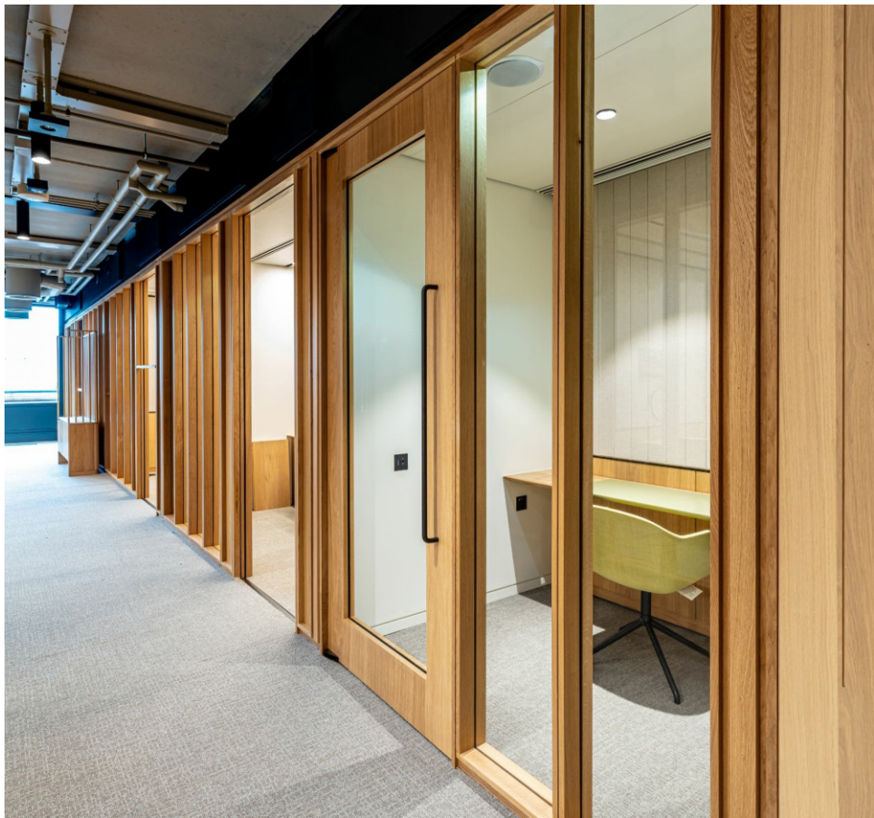
Examples of timber cladding and timber framed glazing
