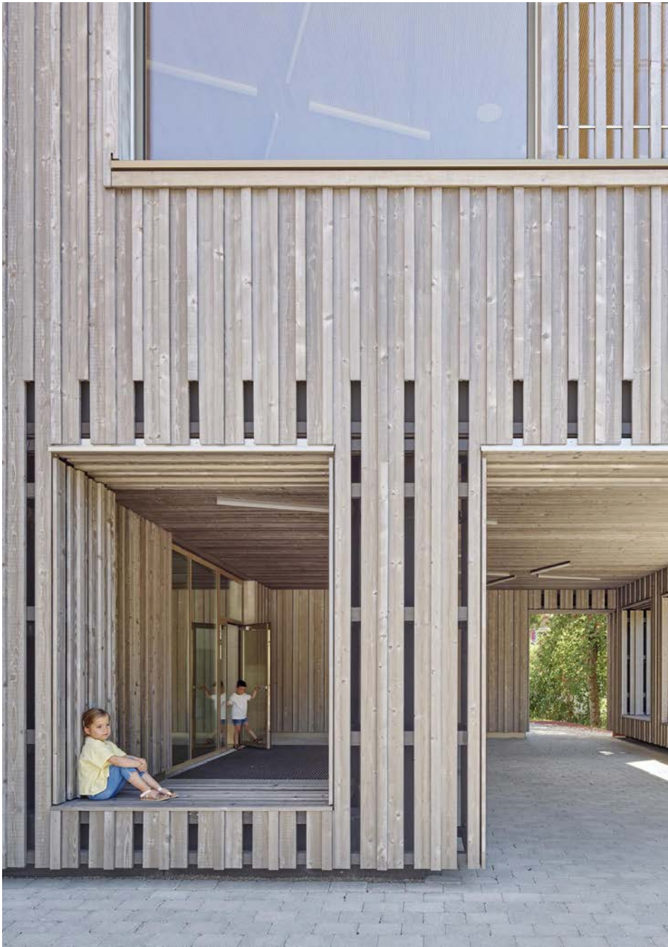
Examples of timber cladding and timber framed glazing
