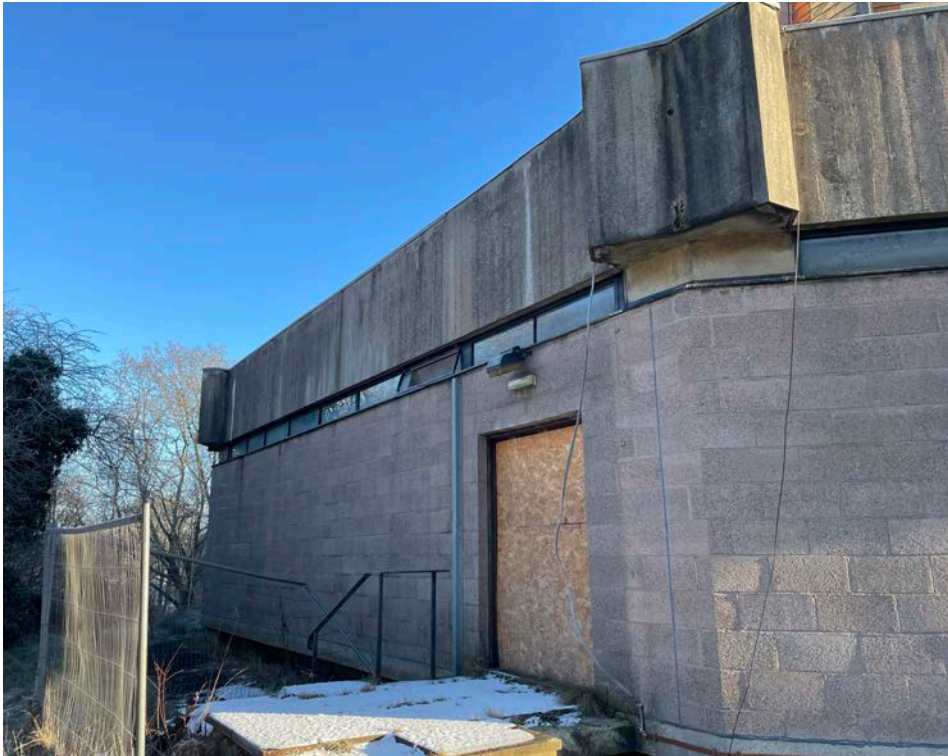
8 View looking at the existing rear access to the building.
