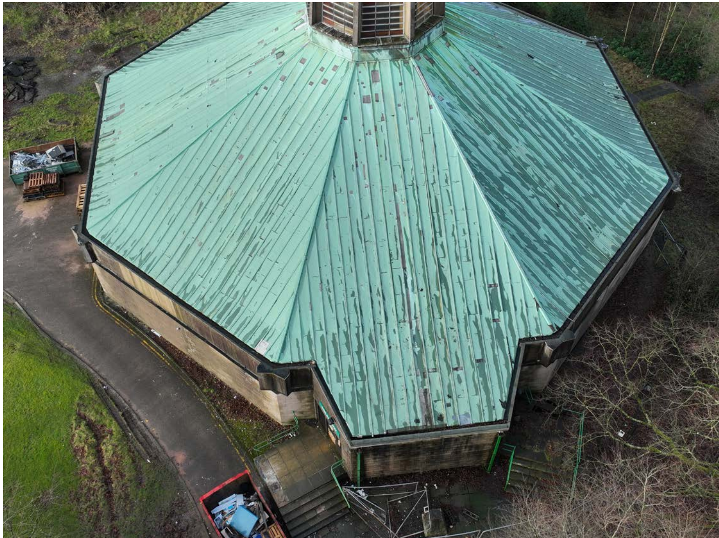
View towards Zone 2 (Image credit: Castle Keep Surveys)
