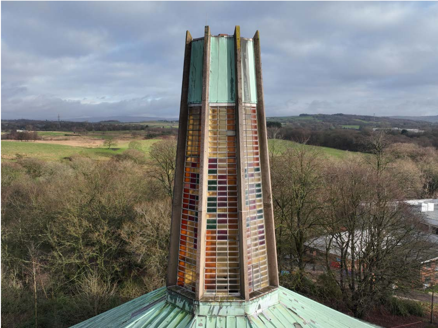
View of Glazed Lantern (Image credit: Castle Keep Surveys)
