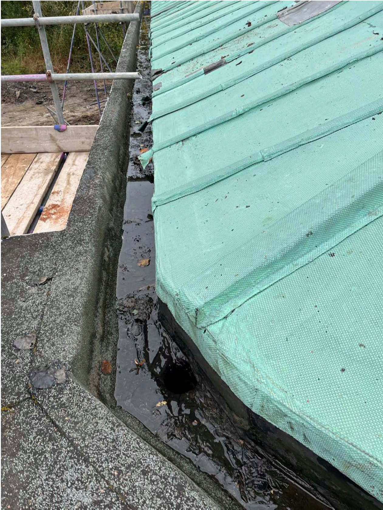
View showing Parapet Gutter Drainage Outlet (Image credit: Seven Architecture)
