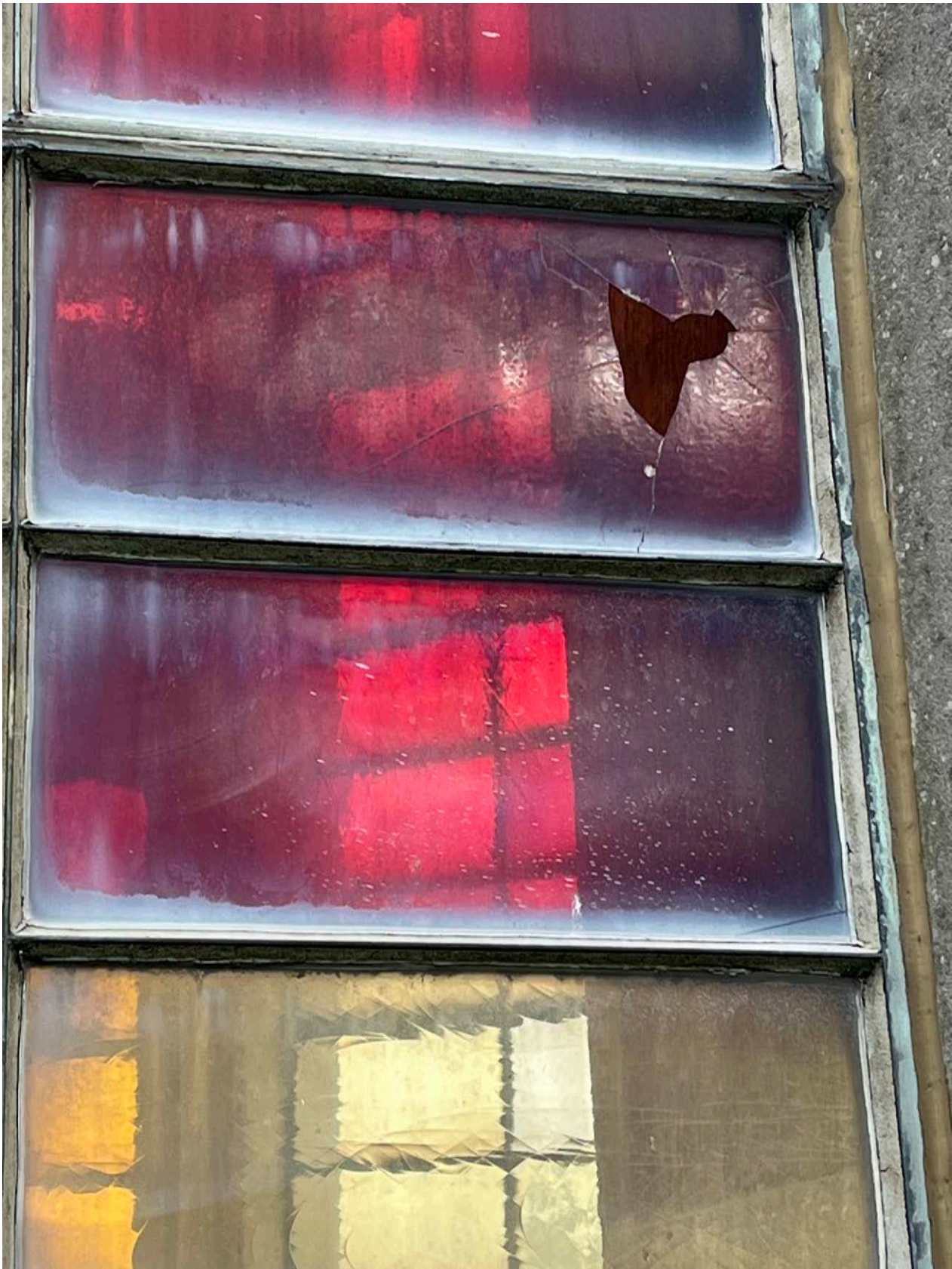
Close Up View showing Glazed Lantern (Image credit: Seven Architecture)
