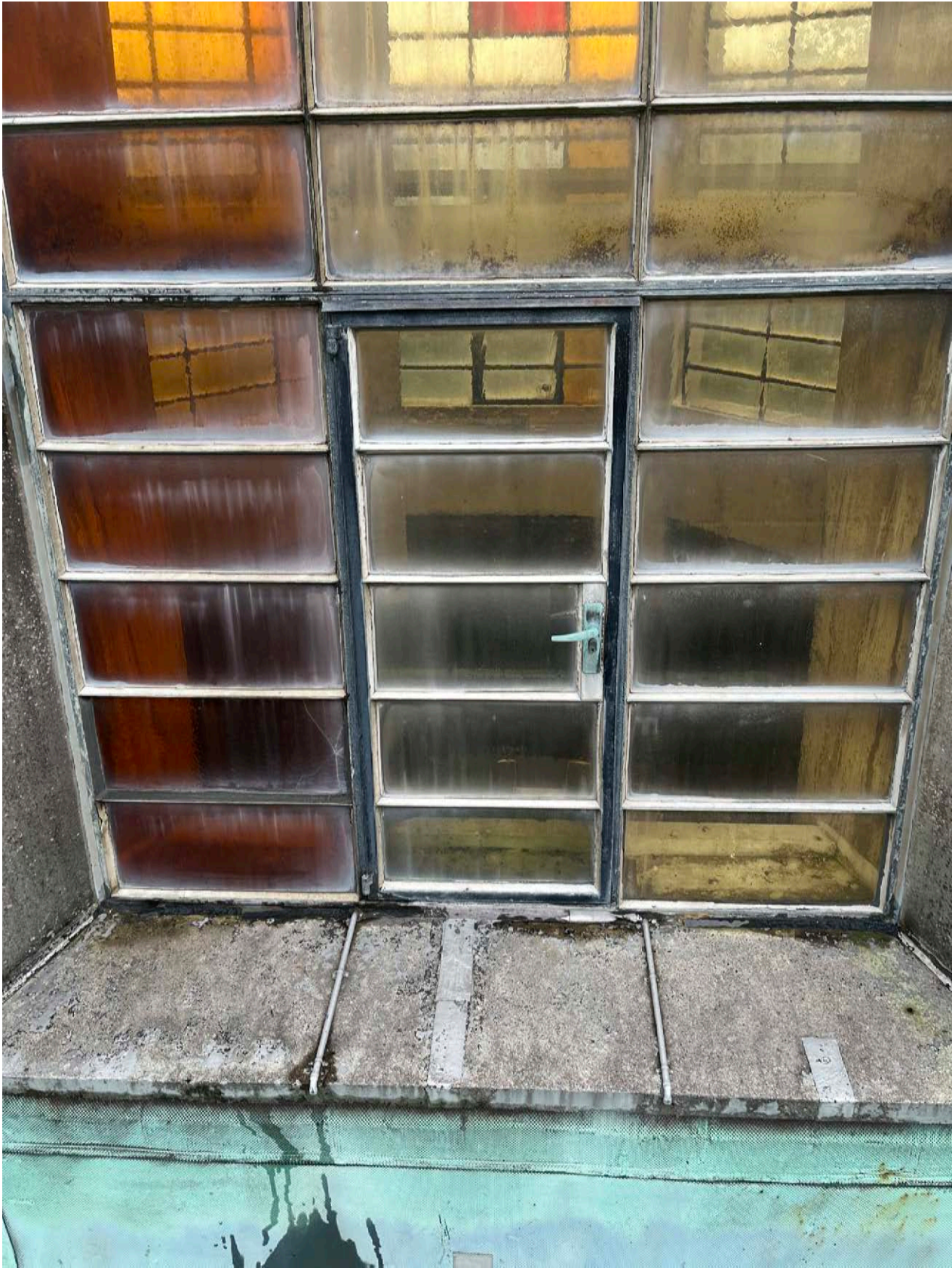
View showing Door within Glazed Lantern (Image credit: Seven Architecture)
