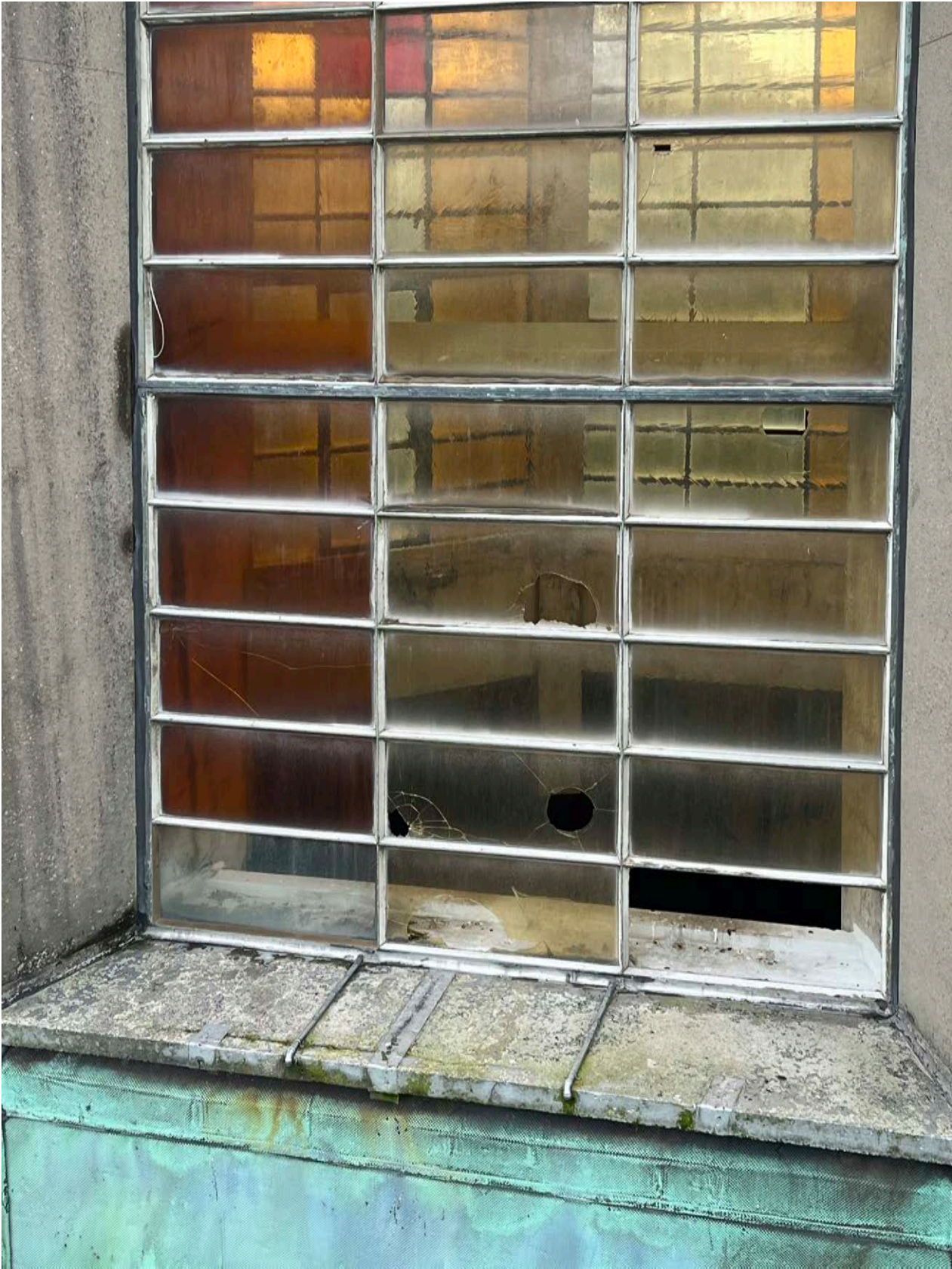
View showing Glazed Lantern (Image credit: Seven Architecture)
