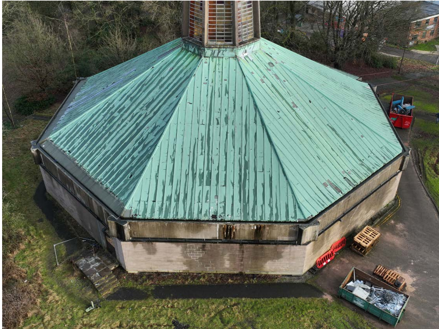
View towards Zone 7 (Image credit: Castle Keep Surveys)
