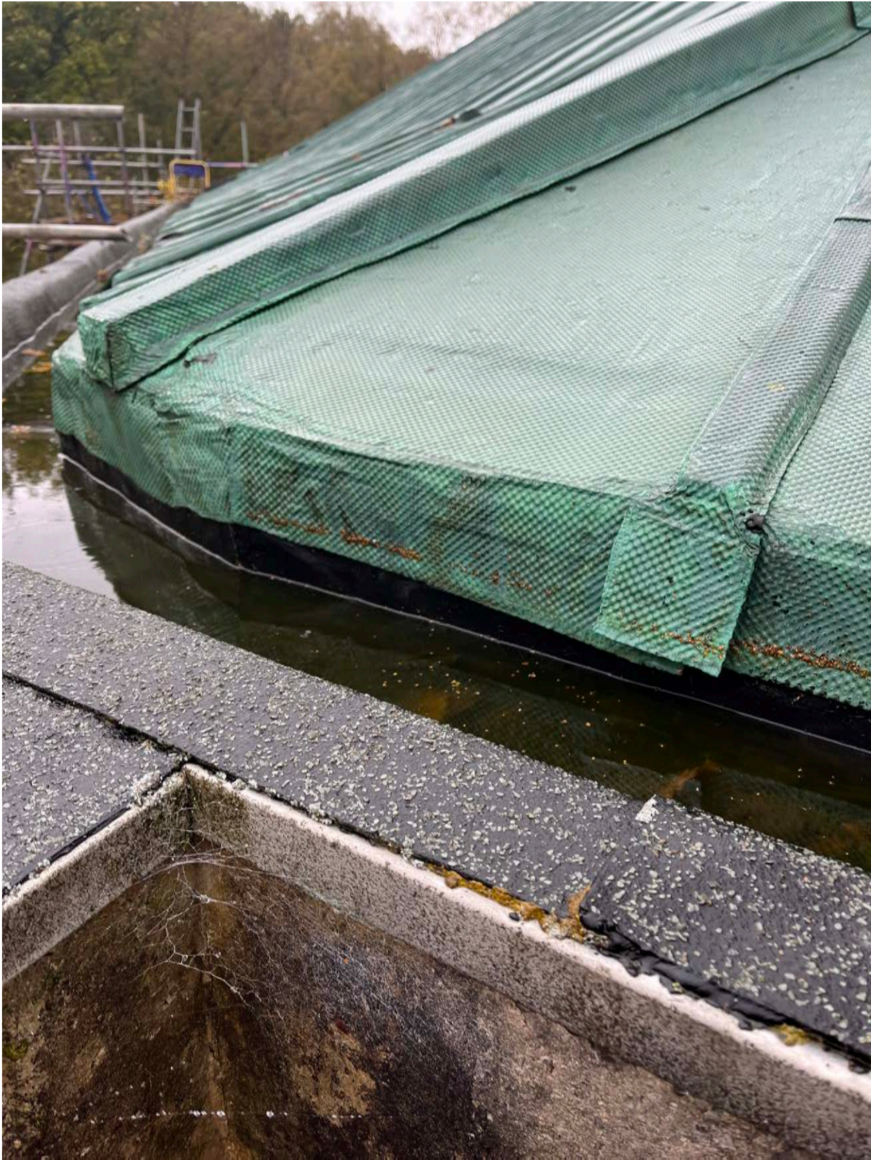
View showing Parapet Gutter (Image credit: Seven Architecture)
