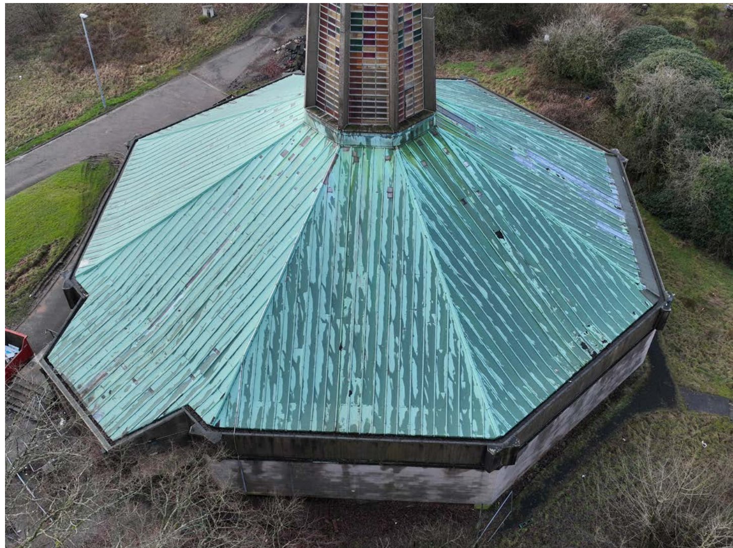
View towards Zone 3 (Image credit: Castle Keep Surveys)
