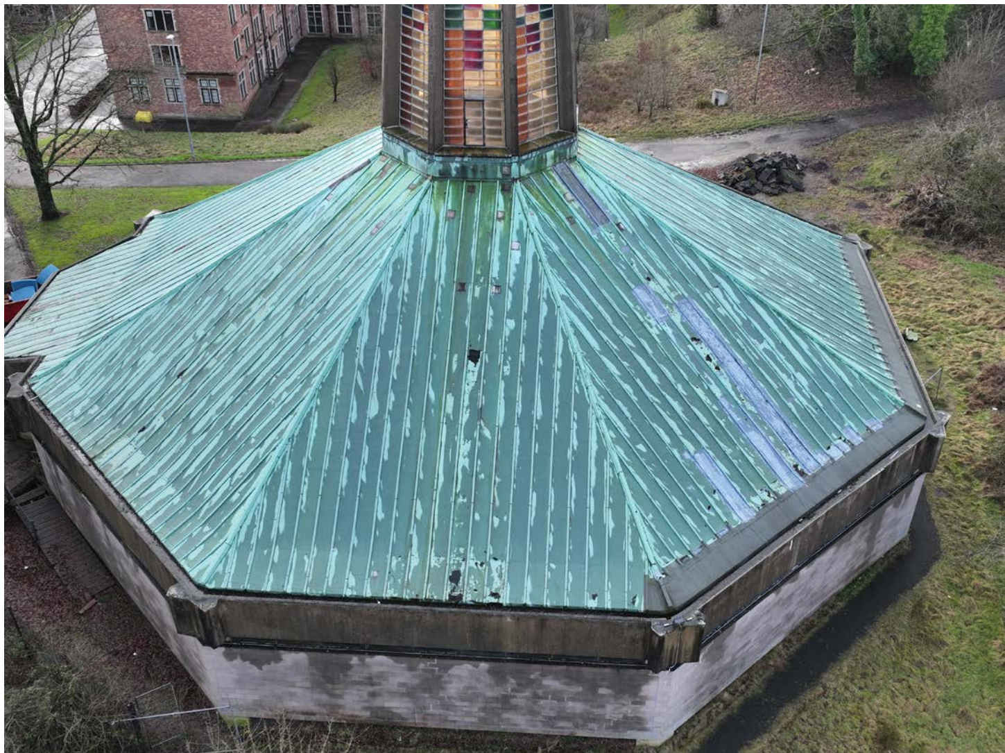
View towards Zone 4 (Image credit: Castle Keep Surveys)
