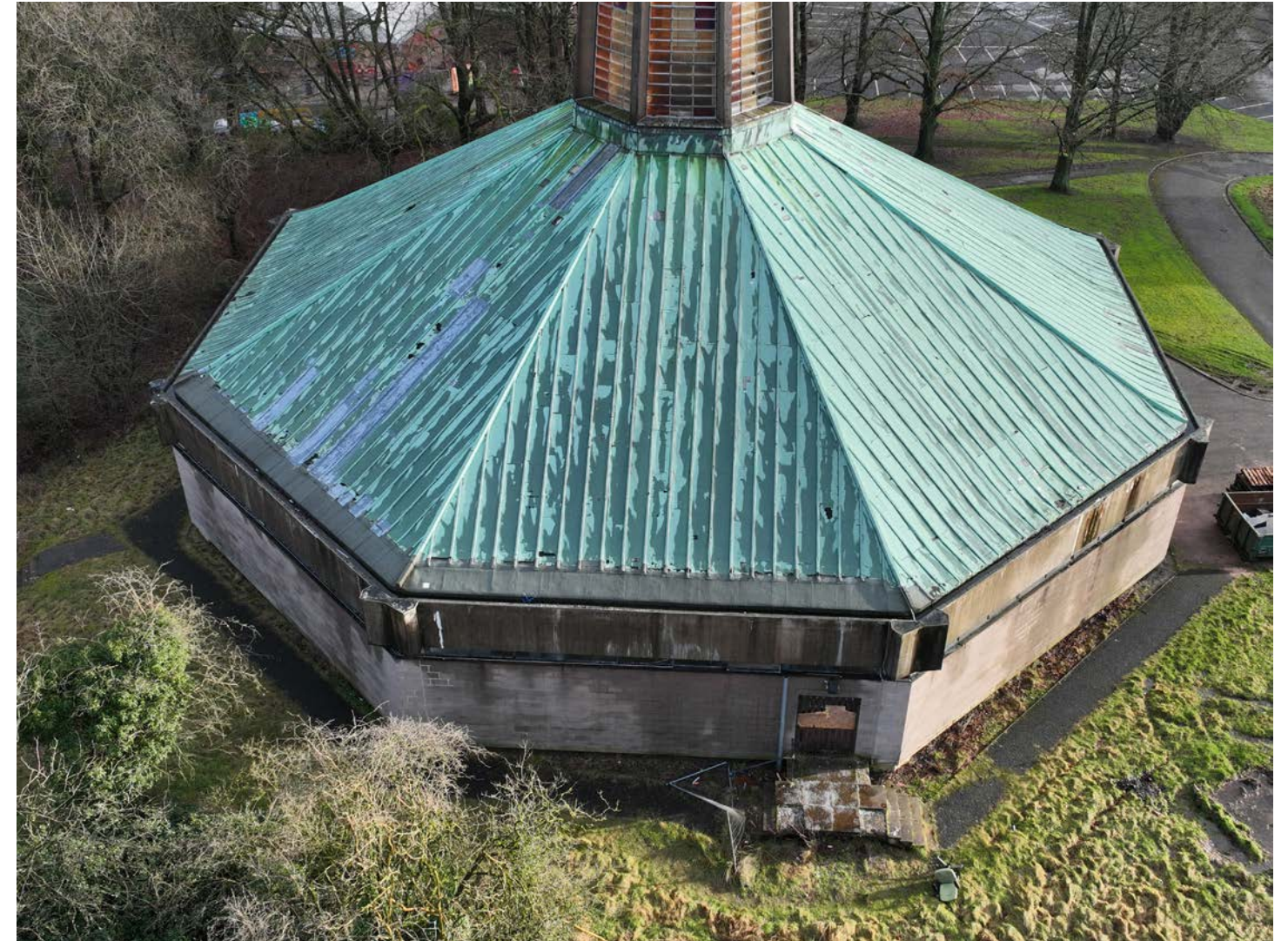
View towards Zone 6 (Image credit: Castle Keep Surveys)
