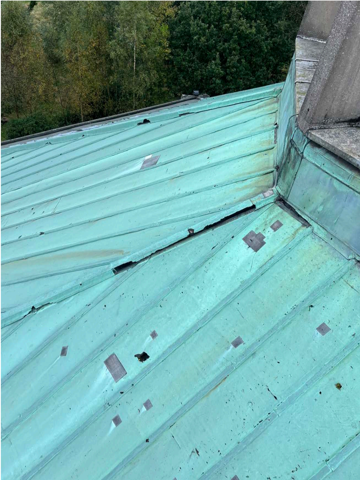
View showing Existing Copper Roof Covering (Image credit: Seven Architecture)
