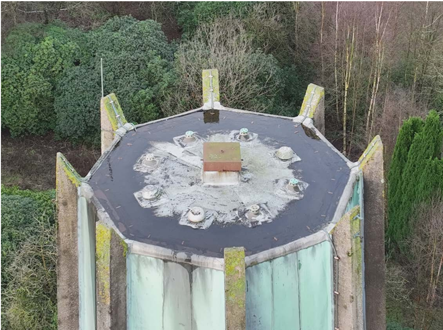
View towards Zone 9 (Image credit: Castle Keep Surveys)
