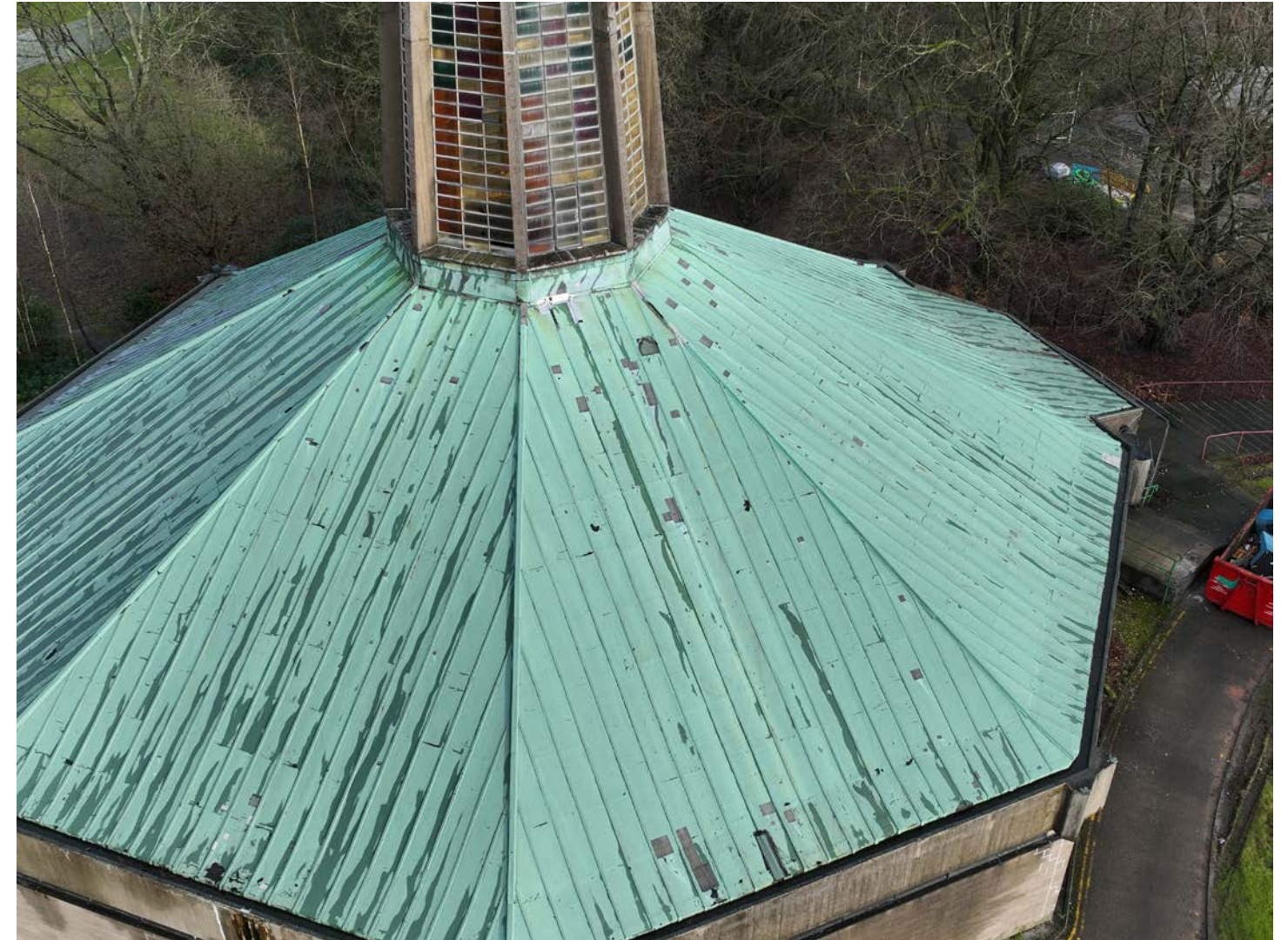
View towards Zone 8 (Image credit: Castle Keep Surveys)
