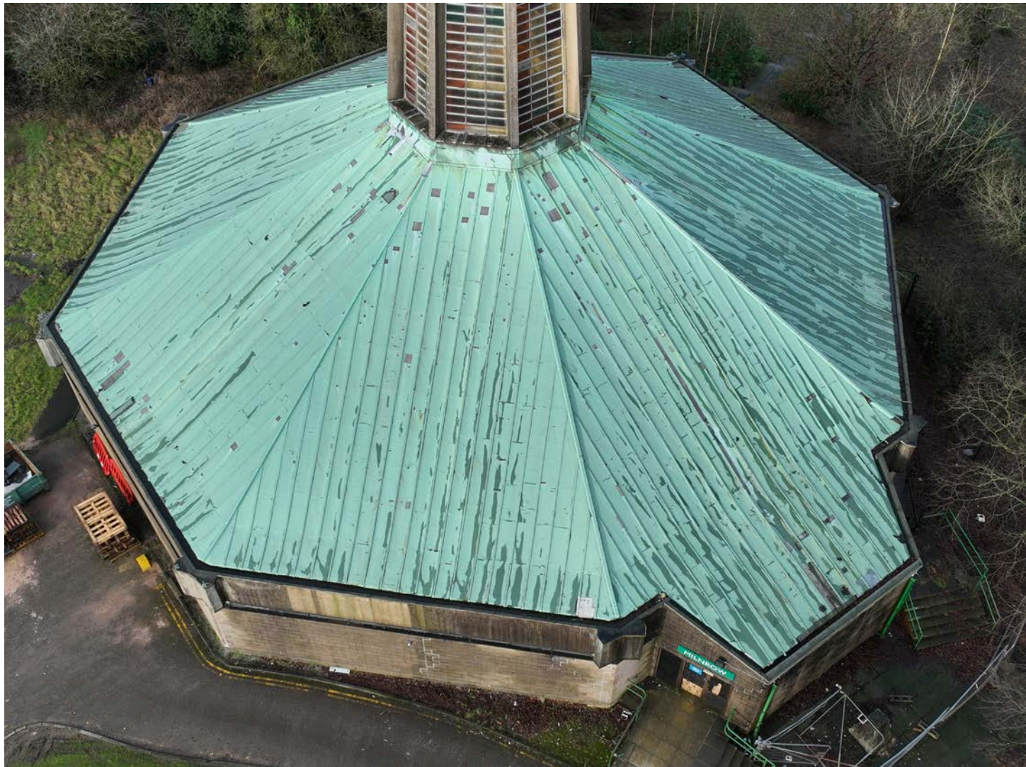
View towards Zone 1 (Image credit: Castle Keep Surveys)
