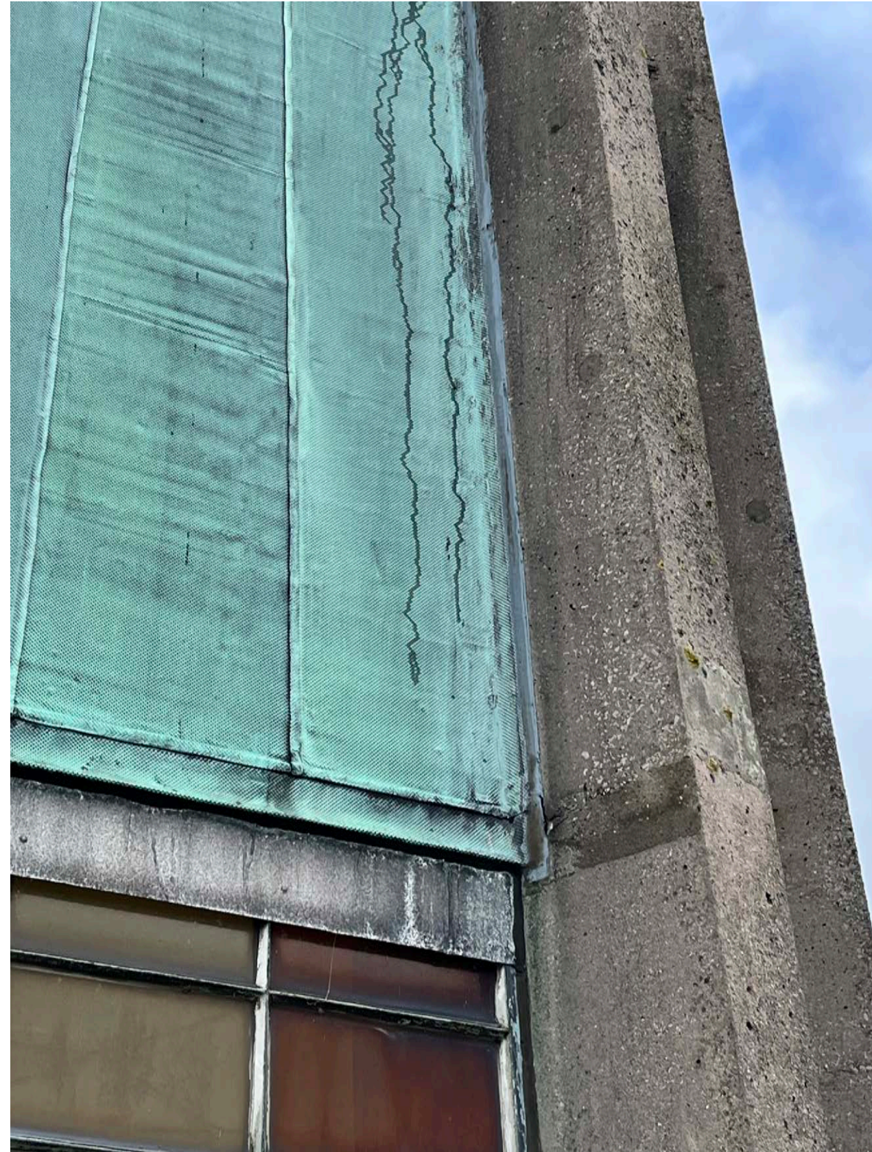
View showing Copper Cladding to Glazed Lantern (Image credit: Seven Architecture)
