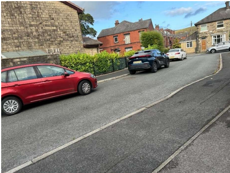
On site photo viewed from Park View towards Town House Road
