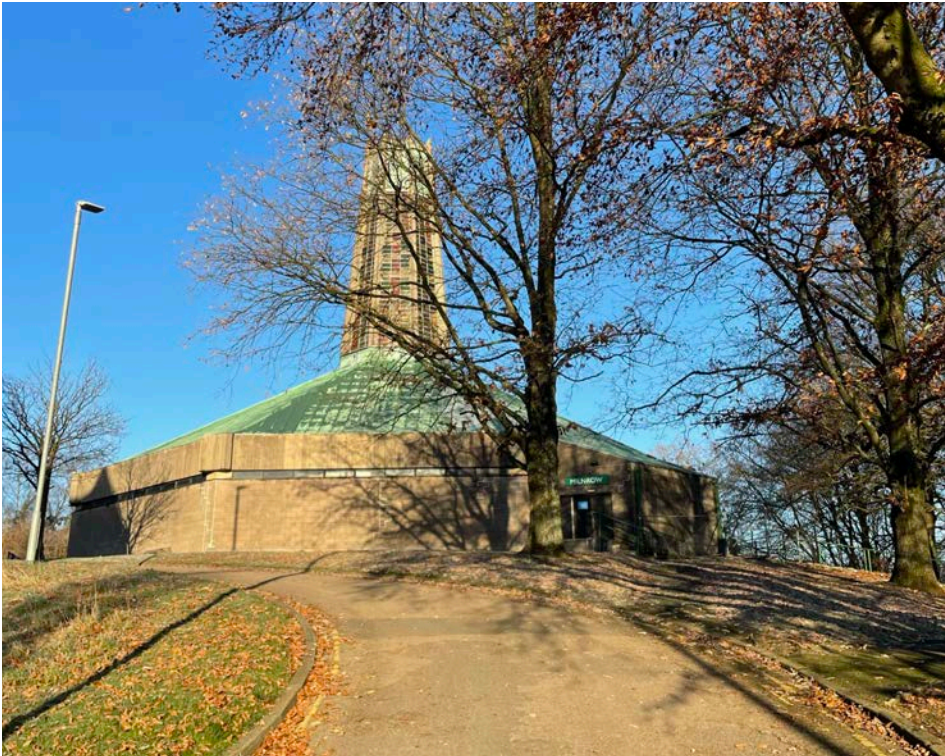
7 View from approach via existing road to the South.
