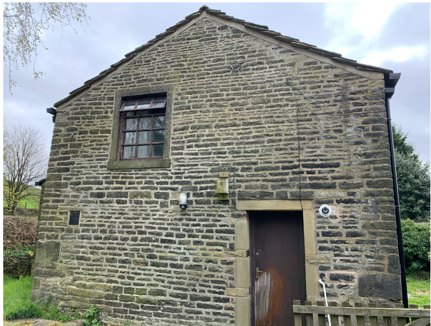
Figure 6 Top: East elevation with C20 lean-to (April 2022 PRIOR TO RENOVATION)
