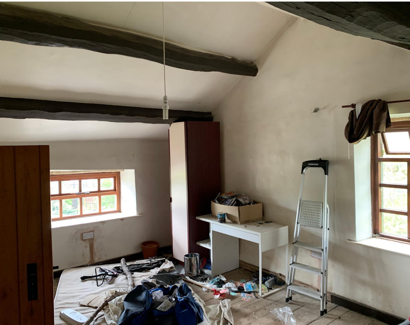
Figure 15 Second floor bedroom (April 2022 PRIOR TO RENOVATION)
