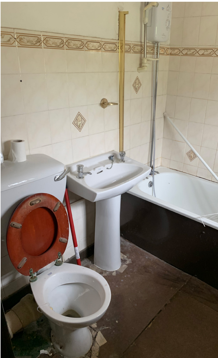
Figure 17 Bathroom located within C20 rear extension (April 2022 PRIOR TO RENOVATION)
