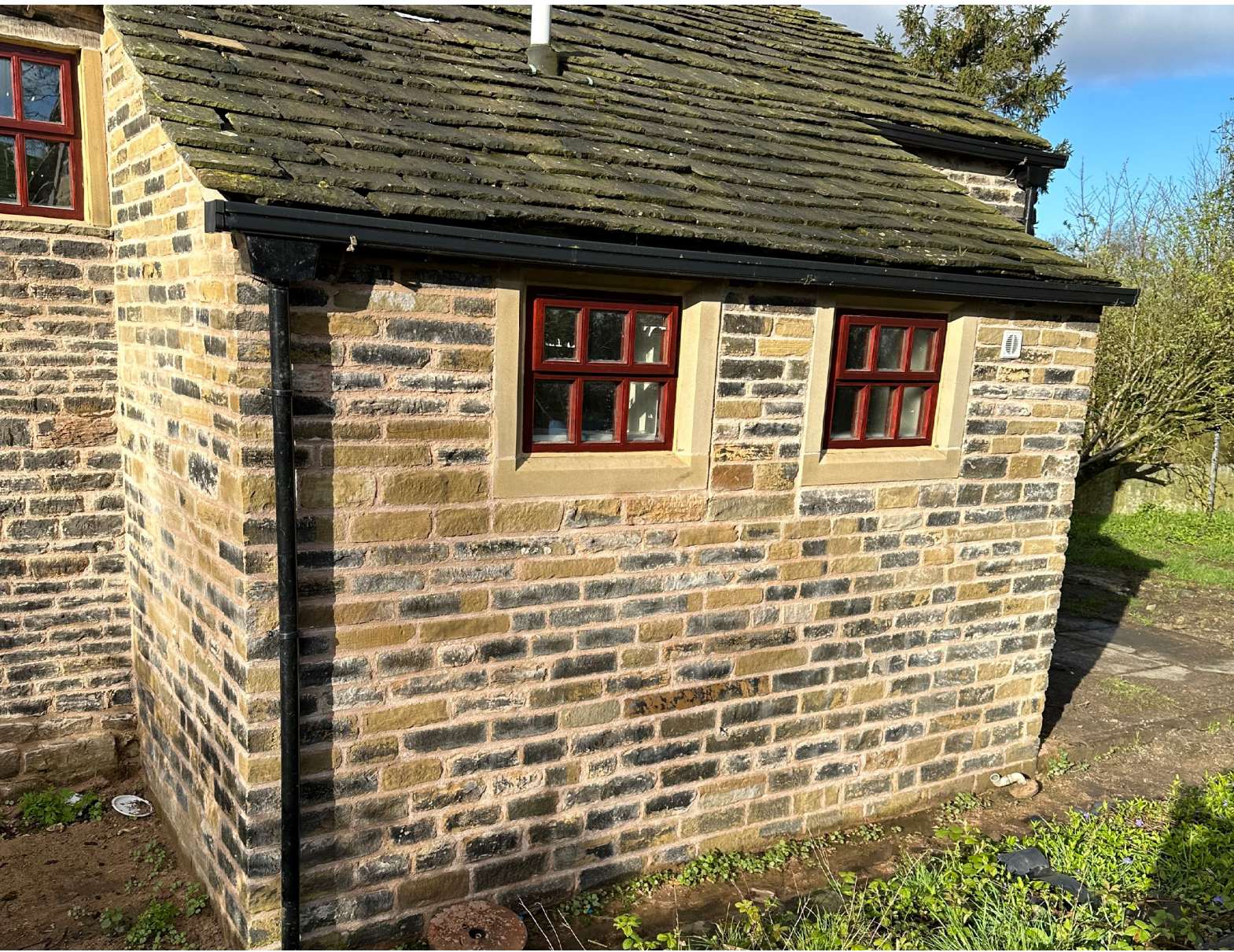
Figure 8 Rear elevation (April 2024 FOLLOWING RENOVATION)
