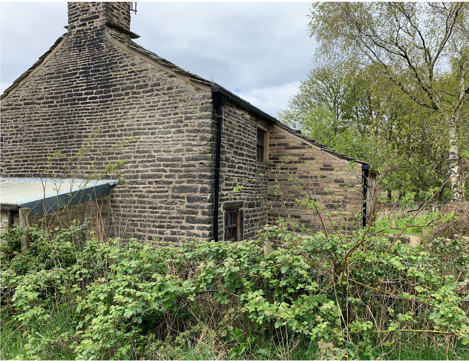
Figure 9 East elevation with view to the rear (April 2022 PRIOR TO RENOVATION)
