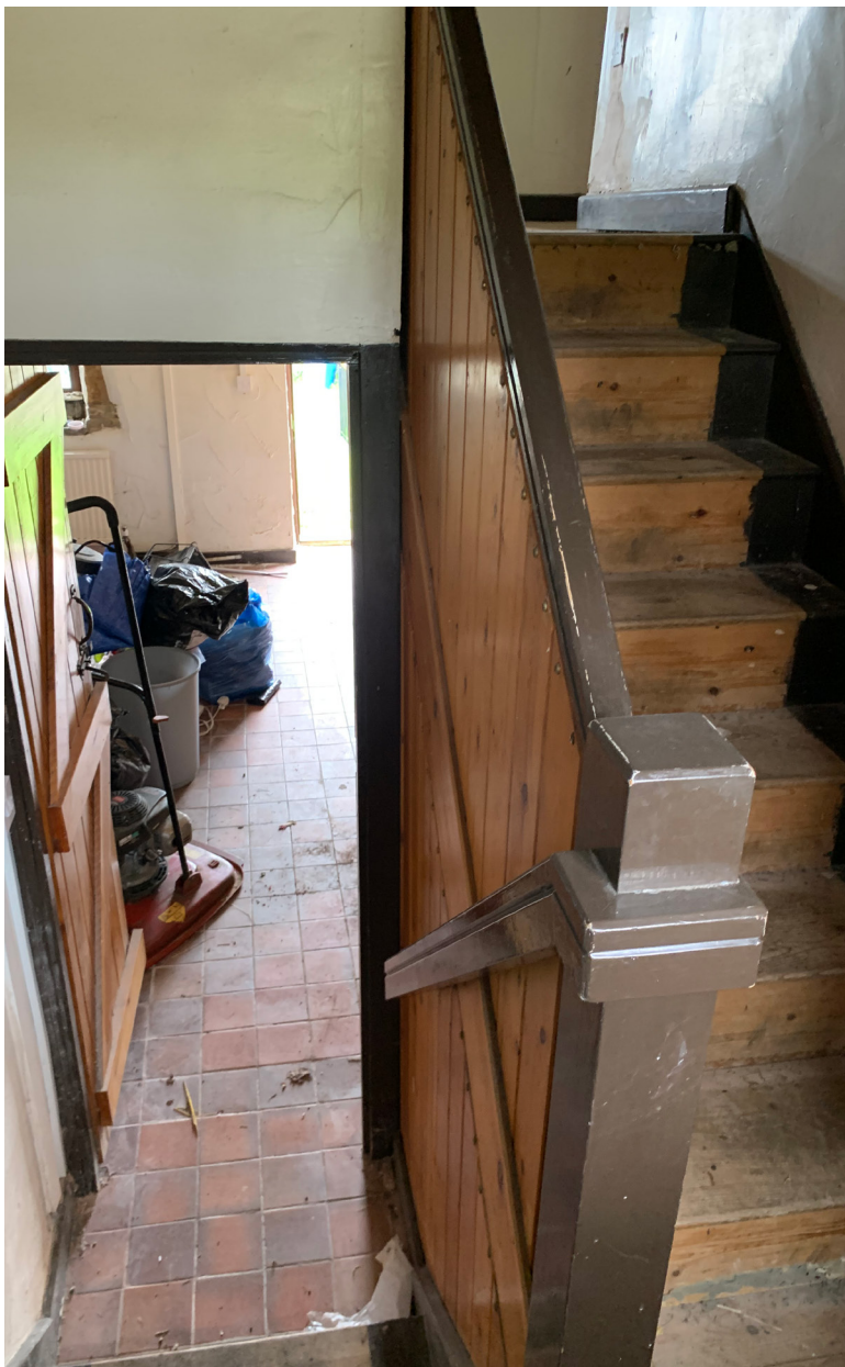
Figure 16 Modern stair in rear extension (April 2022 PRIOR TO RENOVATION)
