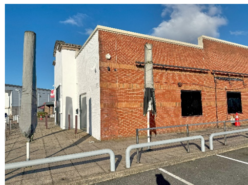
06 View of the side elevation South-east.
