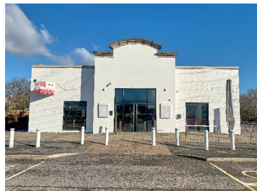
02 View of the front elevation South-west.
