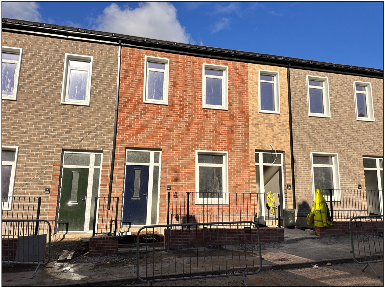
Photograph 1: Front Elevation of the site at Pilsworth Road, Heywood
