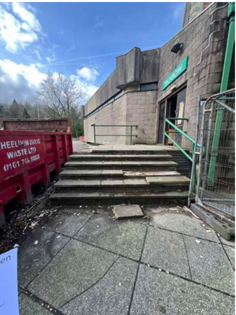
Existing Front Steps to be replaced with new
