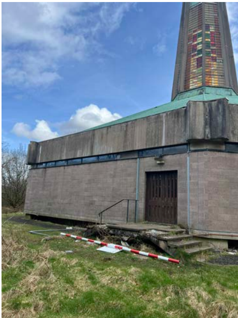
Rear steps to be retained and repaired
