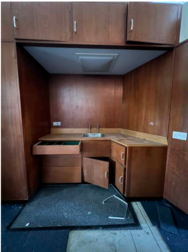
Existing Kitchen Cabinetry and Vestry Cupboards
