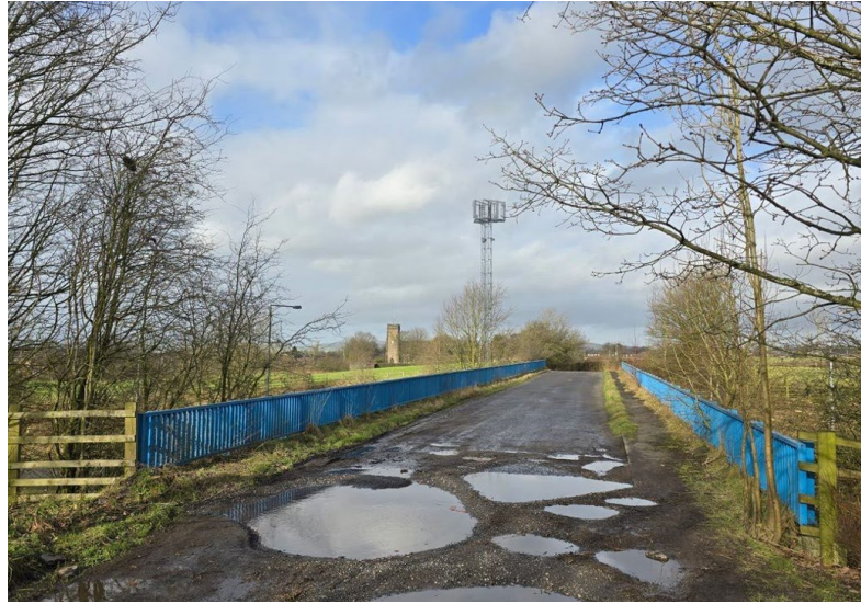
Fig. 23: Viewpoint 1 - View from the footbridge over the A627(M), (as per LPA Delegated Report Fig. 1)
