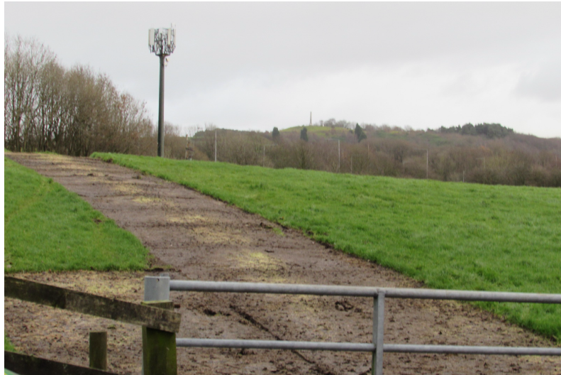
Fig. 4: Existing Cornerstone base station site (the NTQ site)
