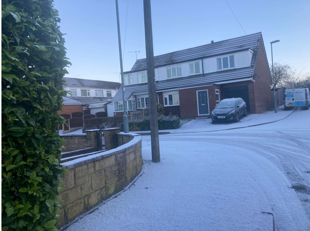
Figure 16; Photograph of no.3 Johnston Avenue showing the two storey side extension.
