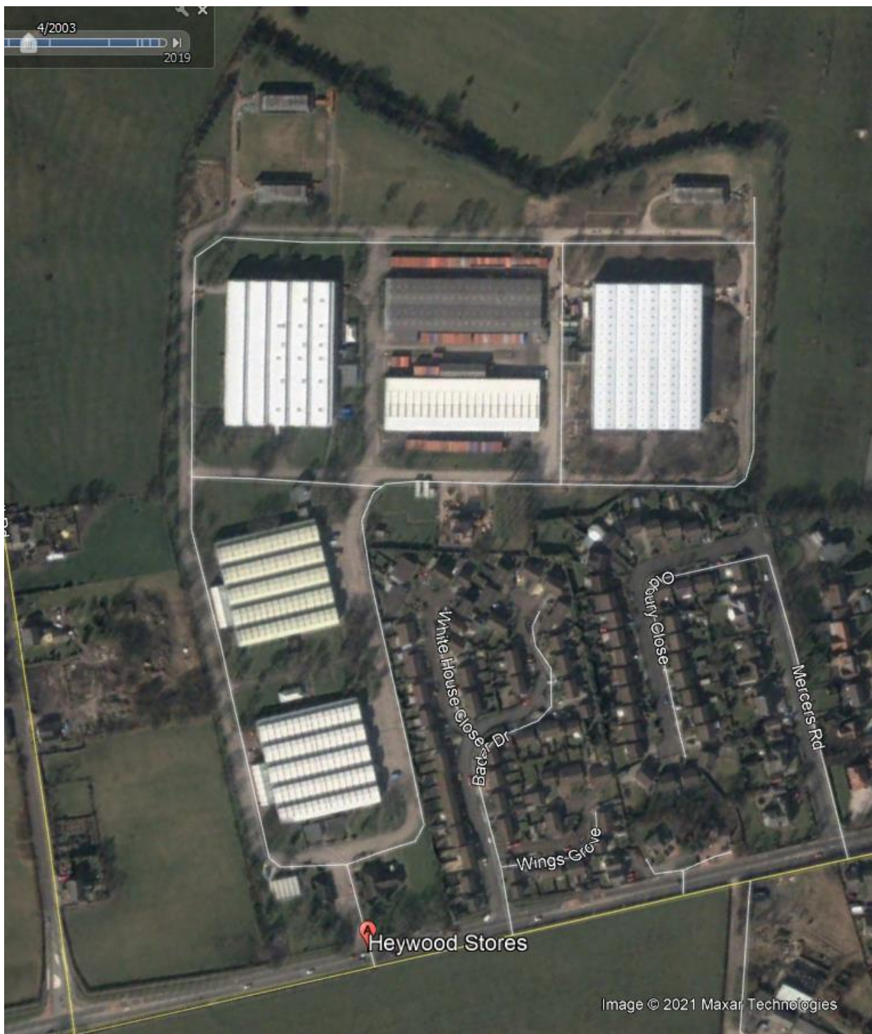
Aerial Photograph April 2003
