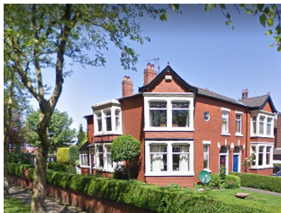
Corner turner at Hopwood Road and Manchester Road Junction *
