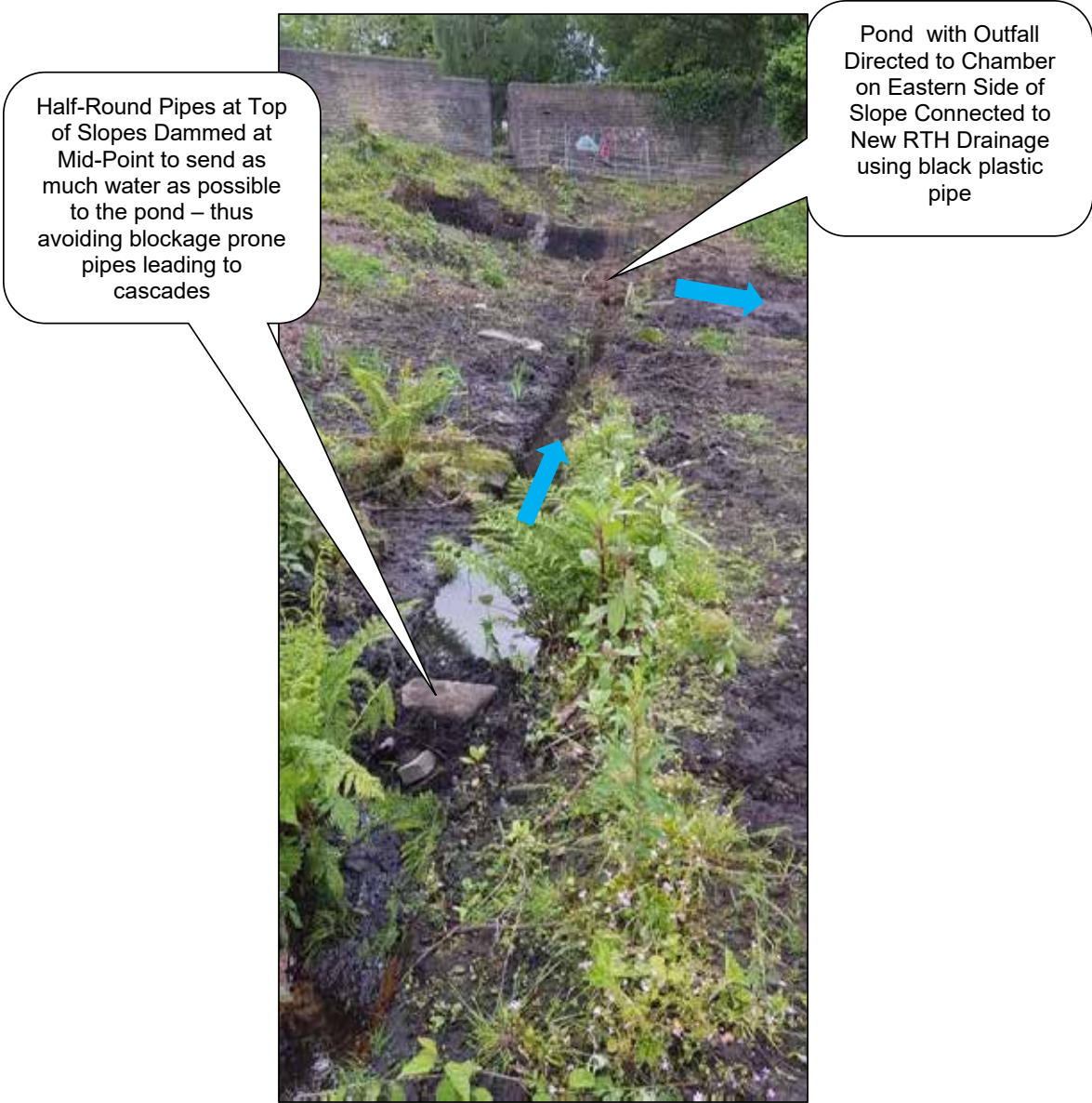
Fig. 8.4 Half-Round Pipes at Top of Slopes Dammed at Mid-Point
