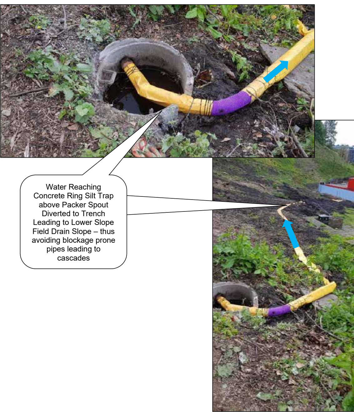
Fig. 8.5 Water Reaching Concrete Ring Silt Trap above Packer Spout Diverted to Trench Leading to Lower Slope Field Drain Slope
