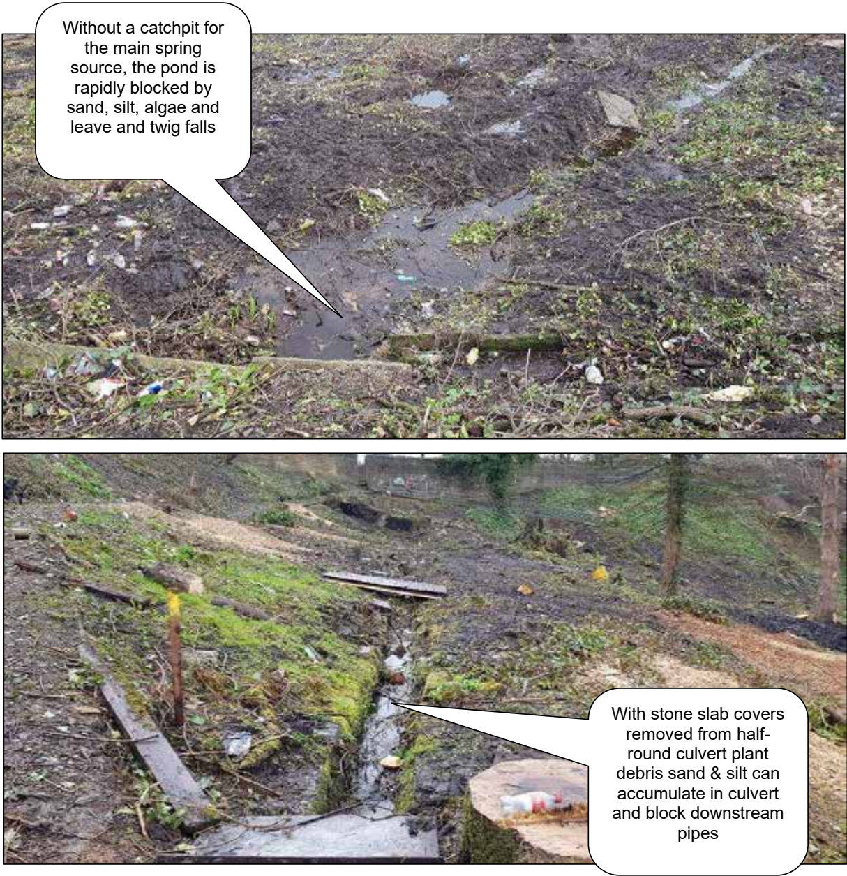
Fig. 6.3 At Main Spring Source for Packer Spout the Spring Catchpit was Removed and Pond Created - Stone Slab Covers Removed from Half-Round Culverts
