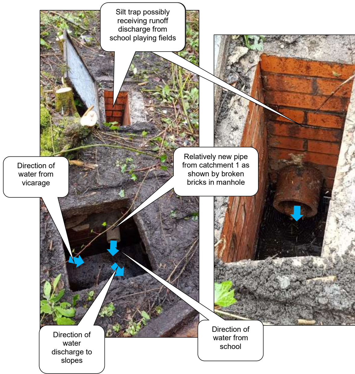
Fig. 11.3 Manhole Next to Garden Gate Receiving Runoff from Direction of Catchment 1 (School Playing Fields)
