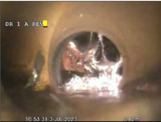
Photo: 5_9a, 00:00:00 4.1m, Junction at 09 o'clock, dia 100 mm
