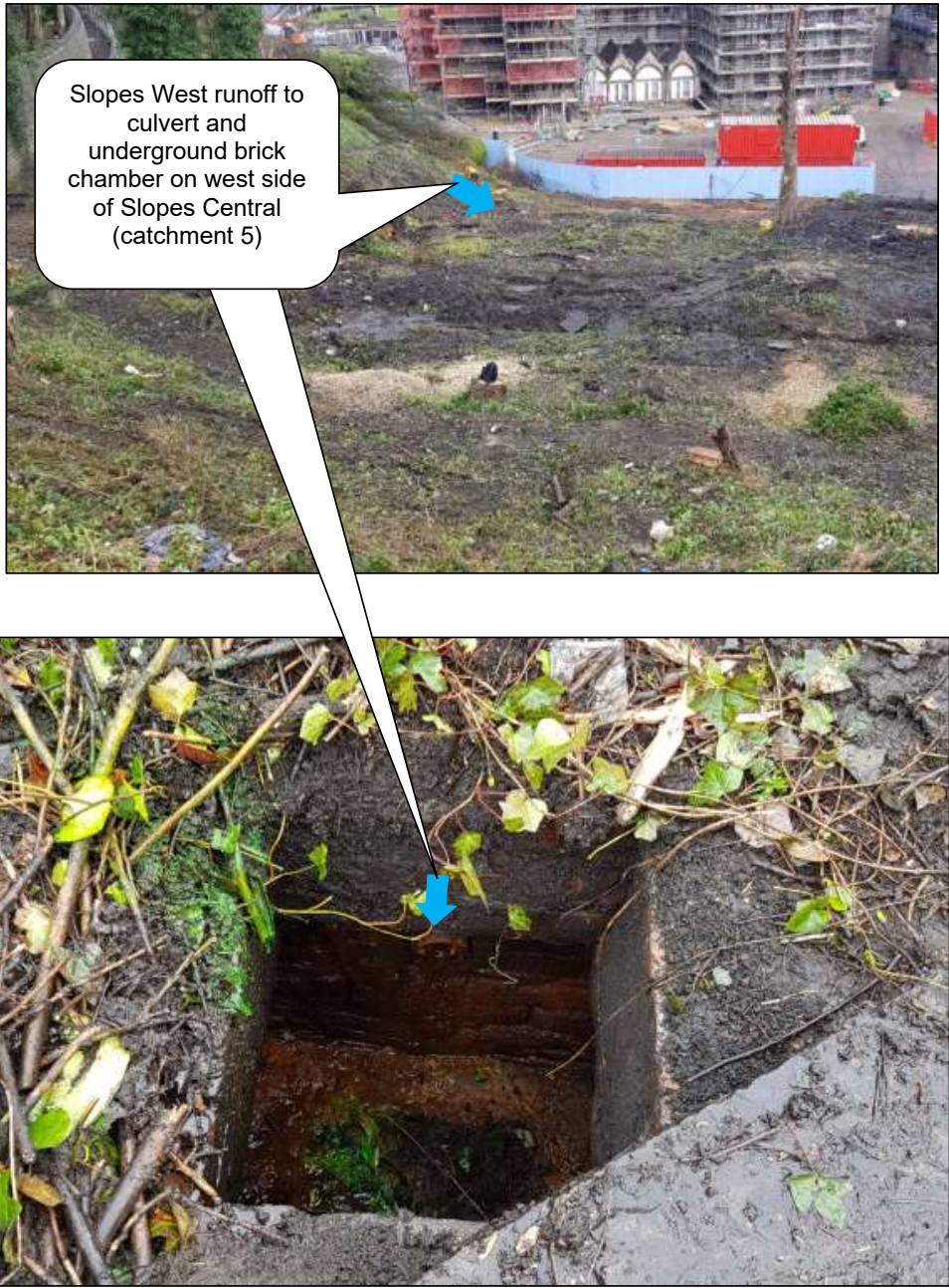
Fig. 14.2 Catchment 4 – Slopes West runoff to culvert and underground brick chamber on west side of Slopes Central (catchment 5)
