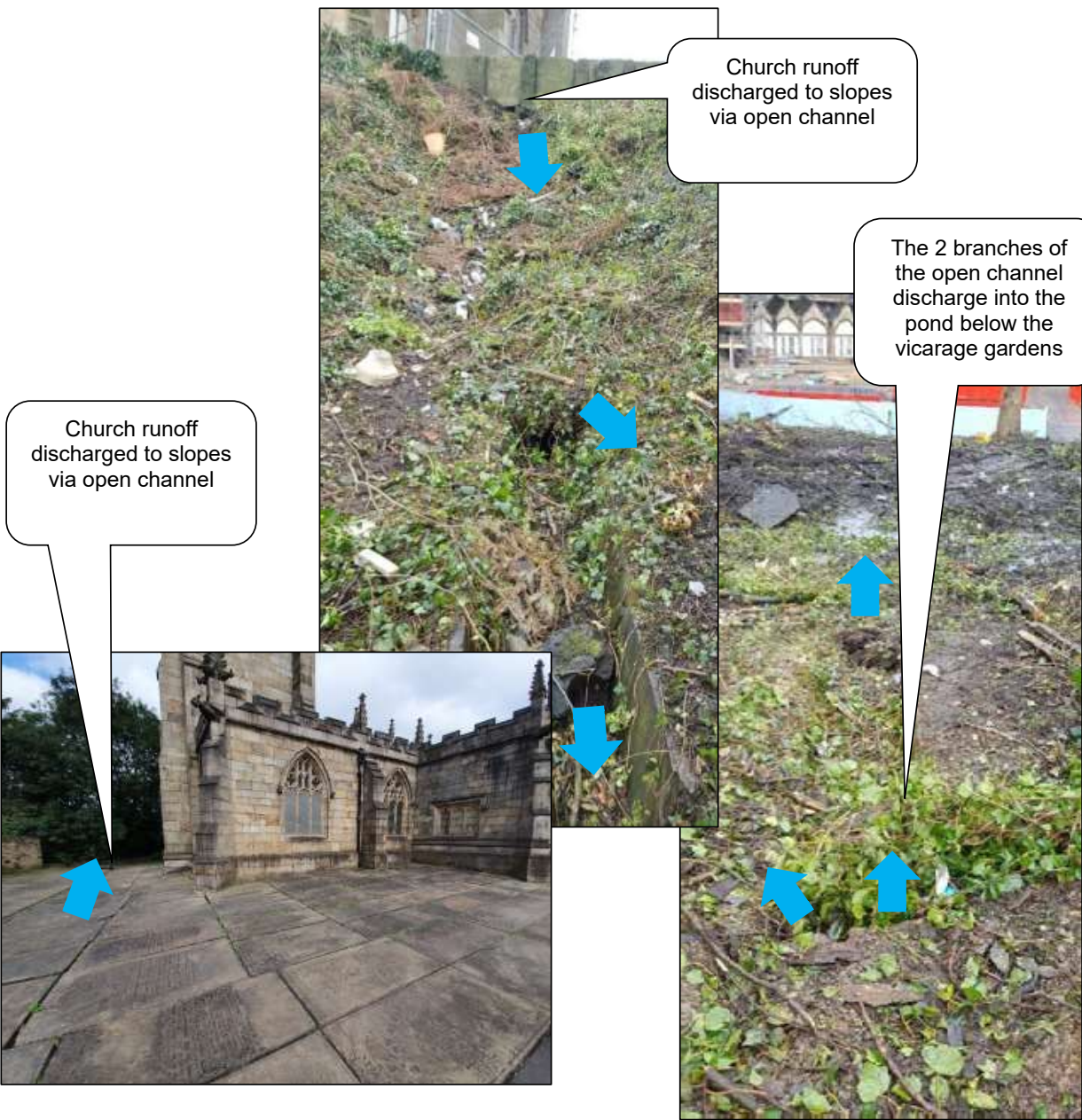
Fig. 13.2 West Side of Church Discharging Runoff to Slopes Via Open Channel to Packer Spout Water Supply – Open Channel Splits into Two Channels Halfway Down Slope
