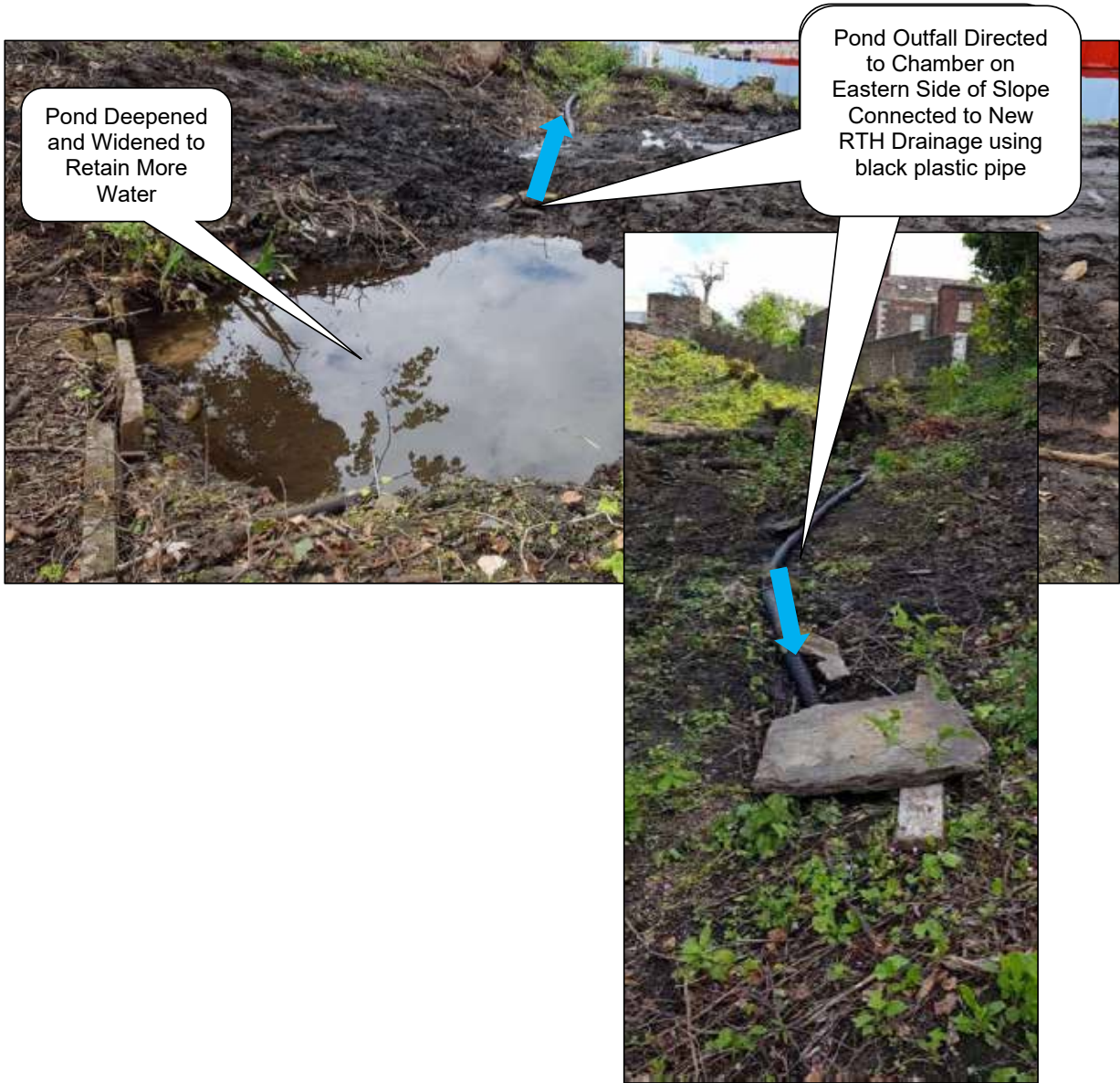
Fig. 8.3 Pond Deepened and Widened to Retain More Water and Pond Outfall Directed to Chamber on Eastern Side of Slope Connected to New RTH Drainage
