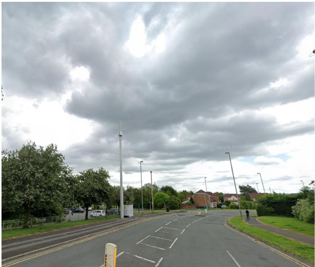
Figure 9 existing streetworks radio base station utilised by another operator at Hazelhurst Drive which cannot be upgraded by VMO2 to provide 5G to the surrounding area
