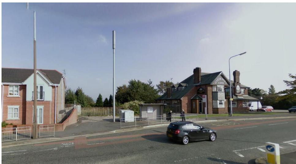
Image 1: Previous 12.5m monopole for Telefonica on Hollin Lane (Source: Googlemaps.com)
