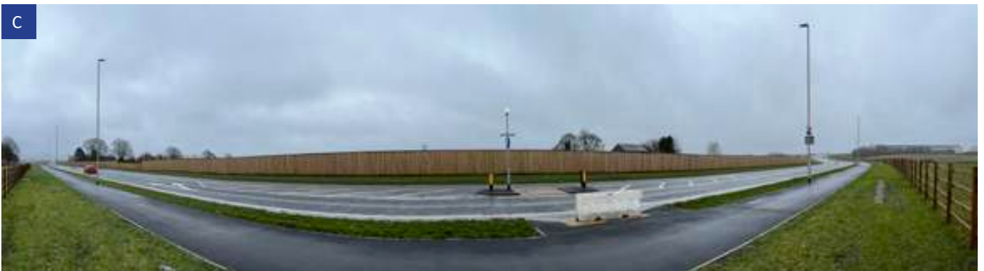
A closed boarded fence borders the southern side of the new link road with distribution warehouses visible in the distance.
