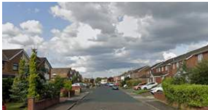
Photo 2. Properties on Salisbury Avenue
