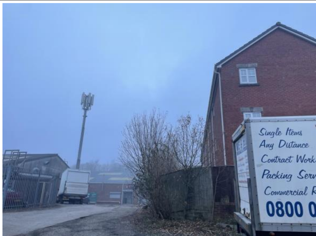
Image 1: Site photograph of existing mast in context of low level industrial buildings and three storey residential townhouses.
