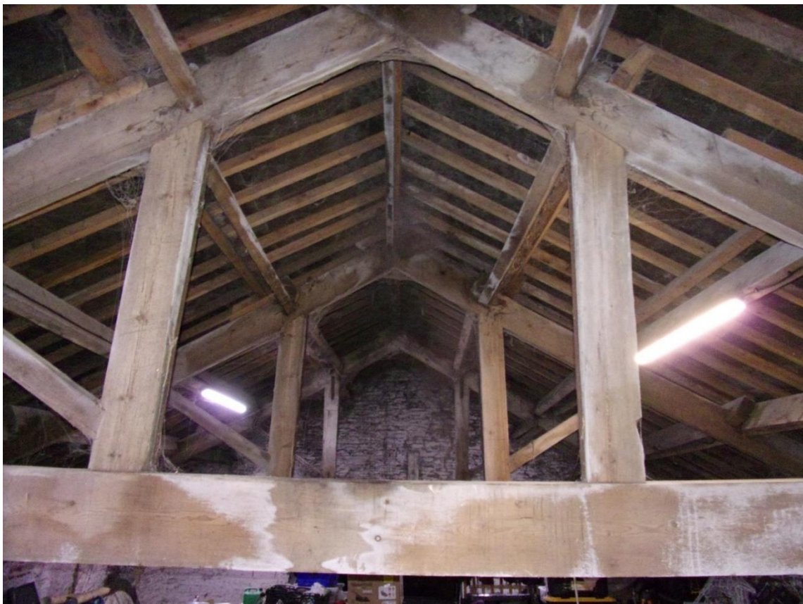
Plate 70 Queen post truss facing east
