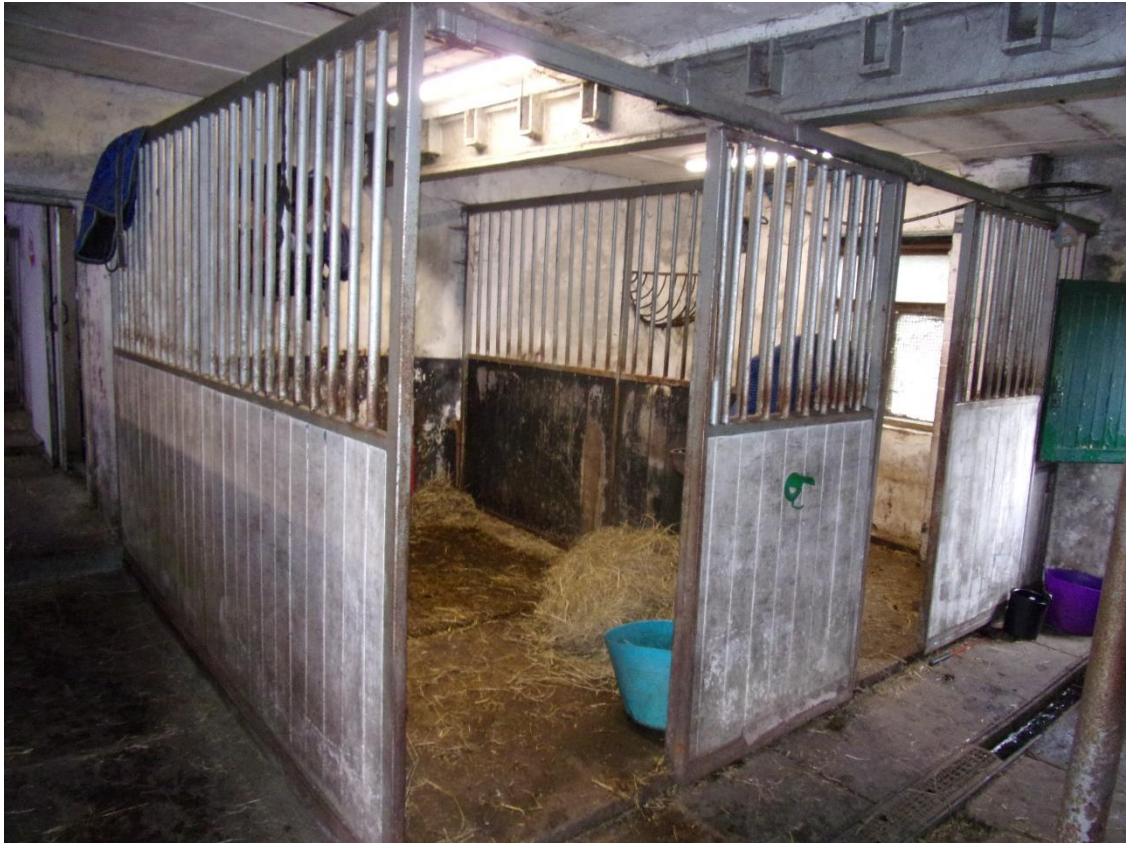
Plate 46 View into Room 6 from the northwest corner
