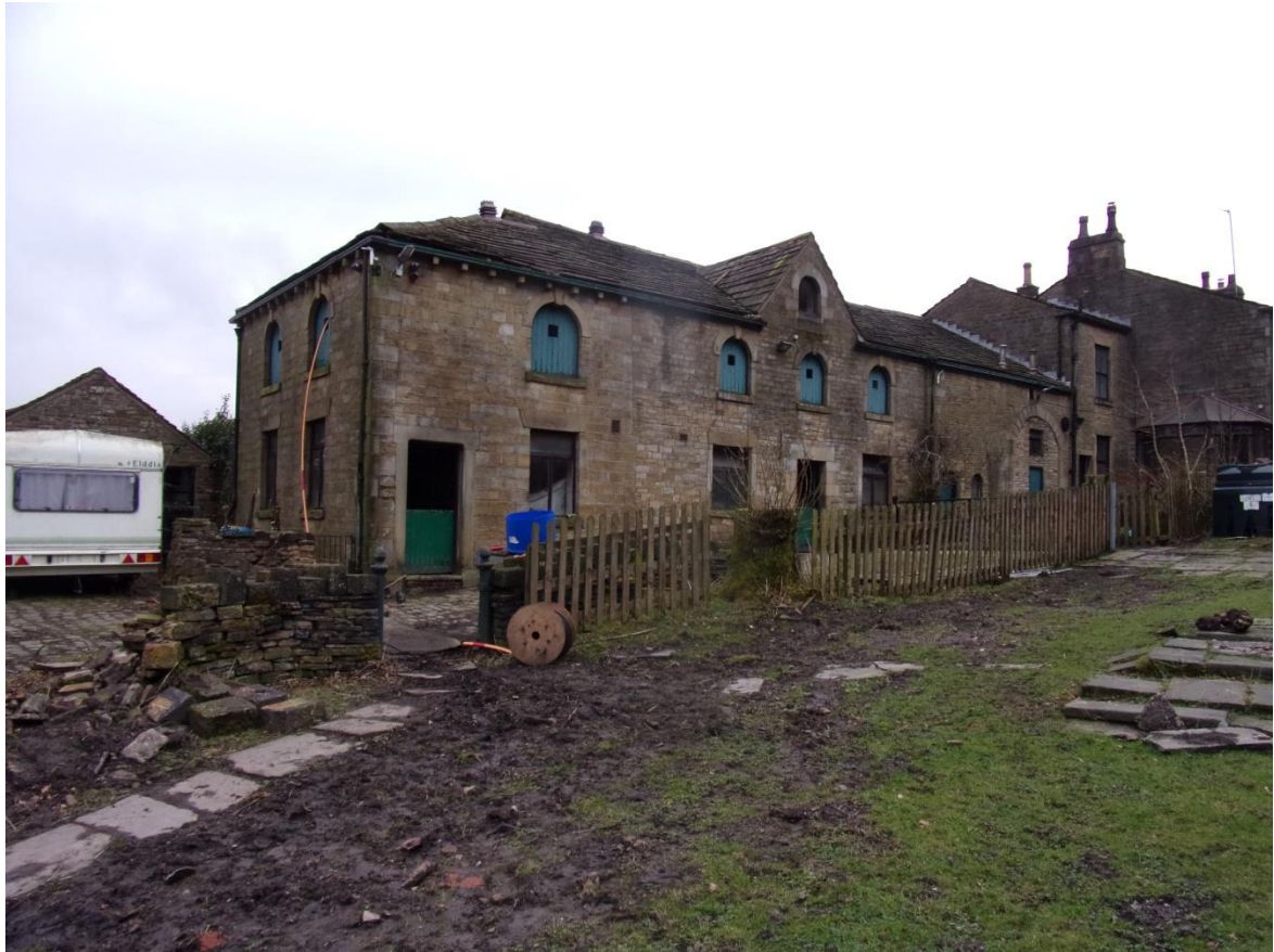
Plate 11 South and east elevations facing northeast
