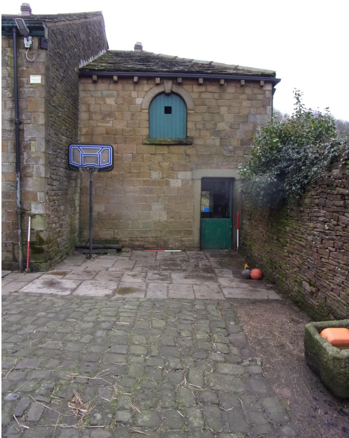
Plate 4 North elevation of the western stable facing south
