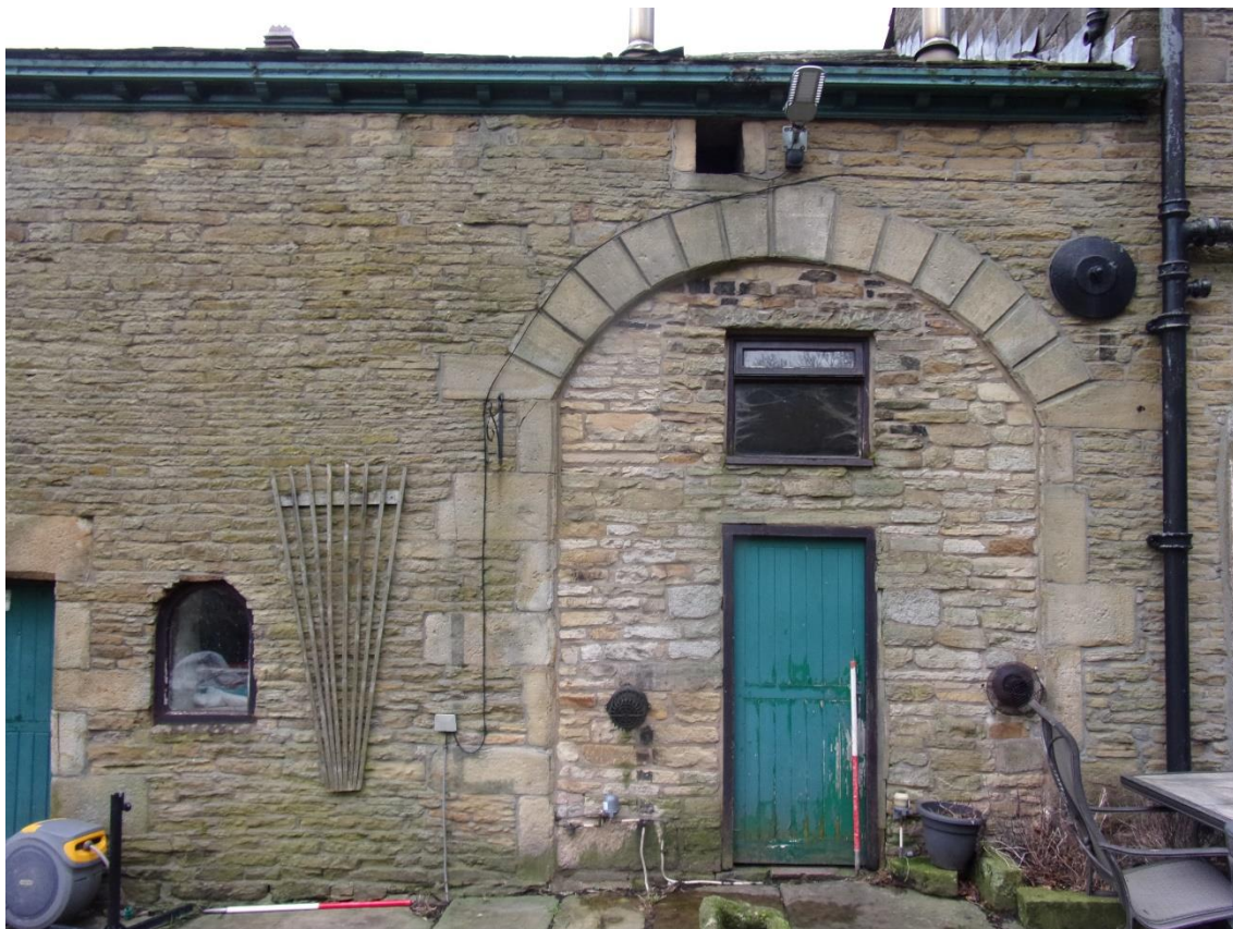
Plate 16 Blocked cart door in the south elevation facing north
