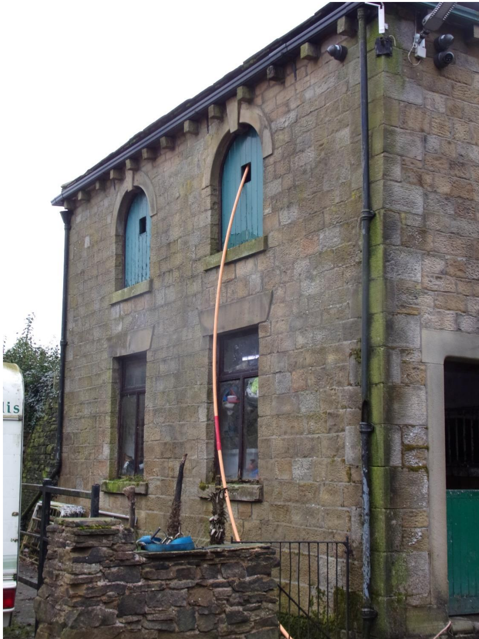
Plate 19 West elevation facing northeast
