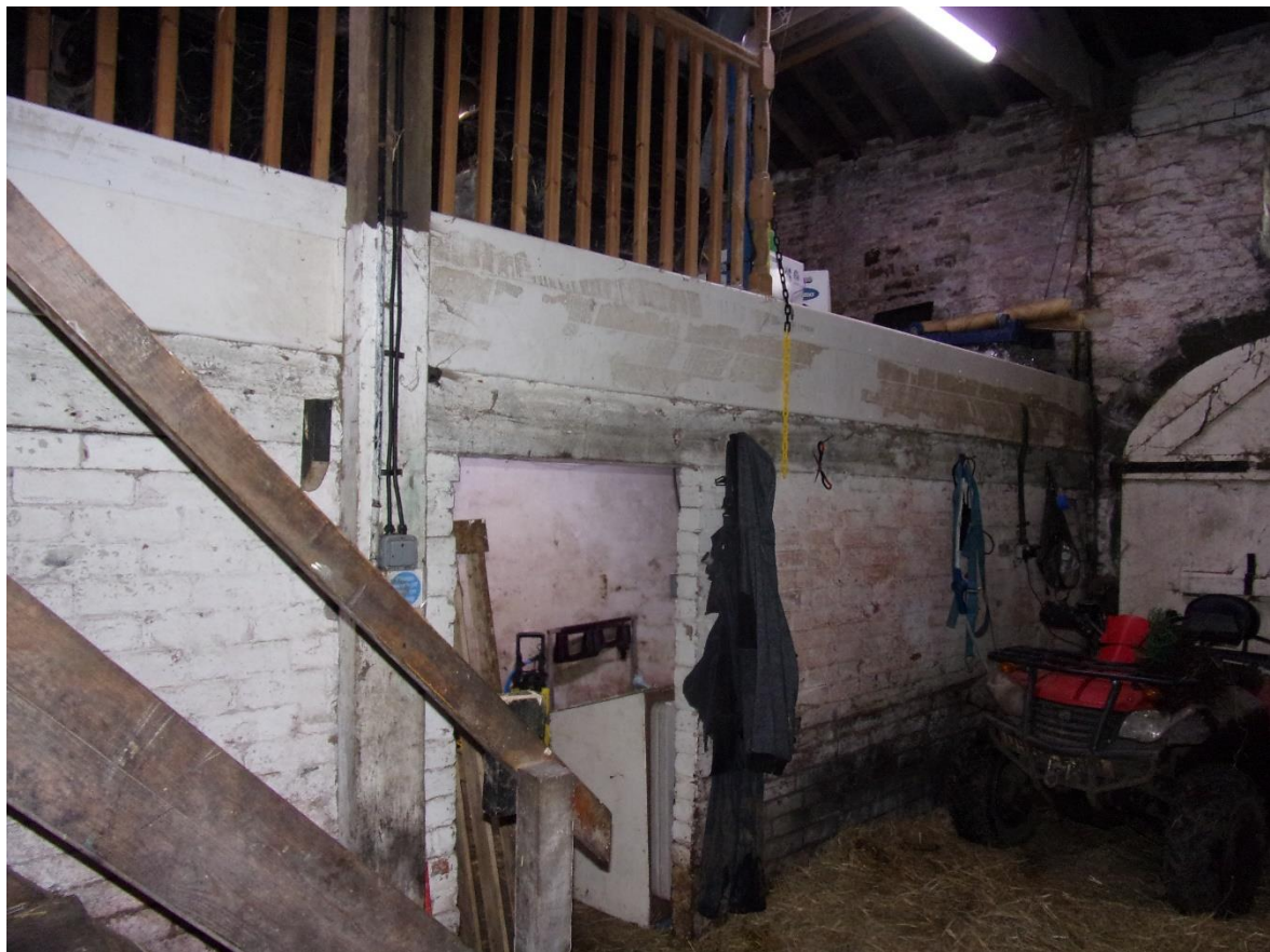
Plate 29 Partition wall in Room 1, facing northwest
