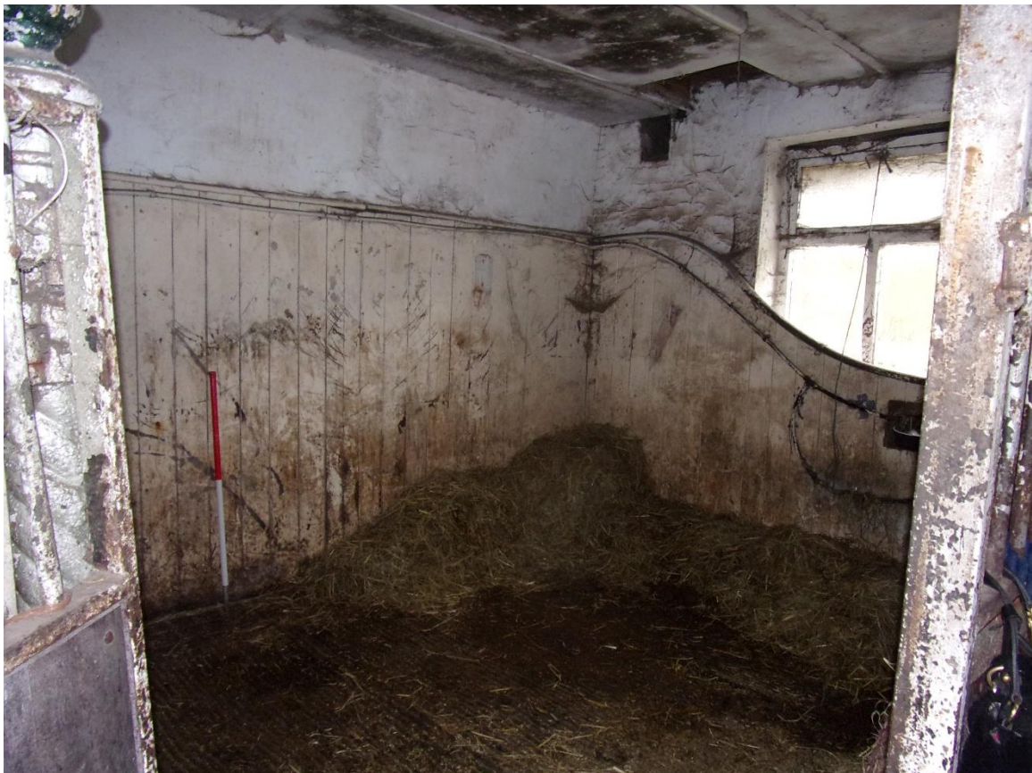
Plate 54 Timber panelling in Room 11, facing southeast
