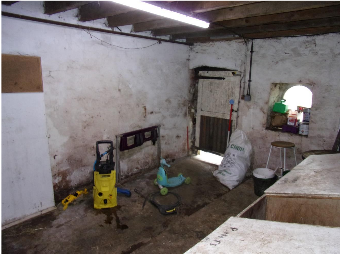
Plate 33 West internal elevation of Room 2, facing northwest
