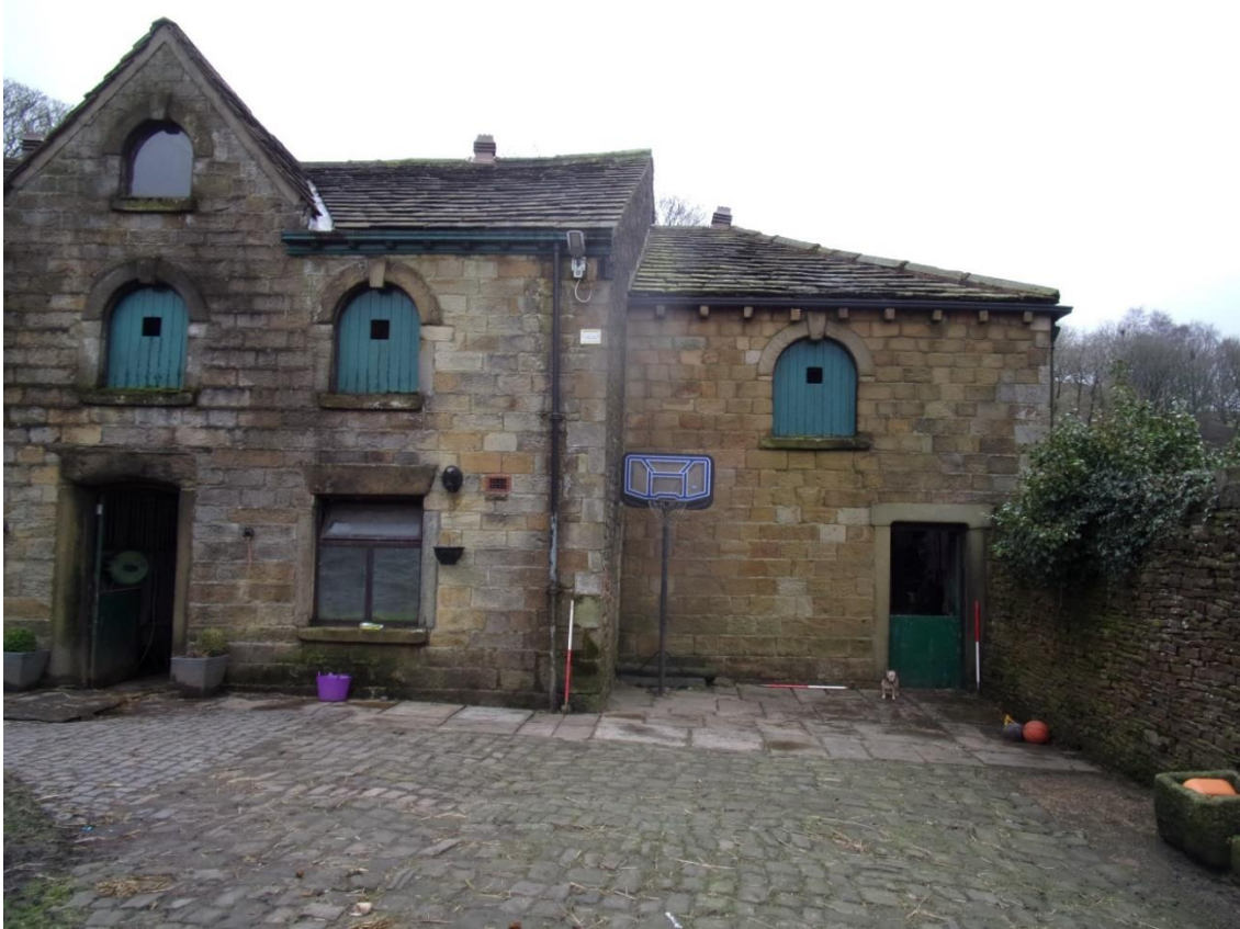
Plate 3 North elevation facing south
