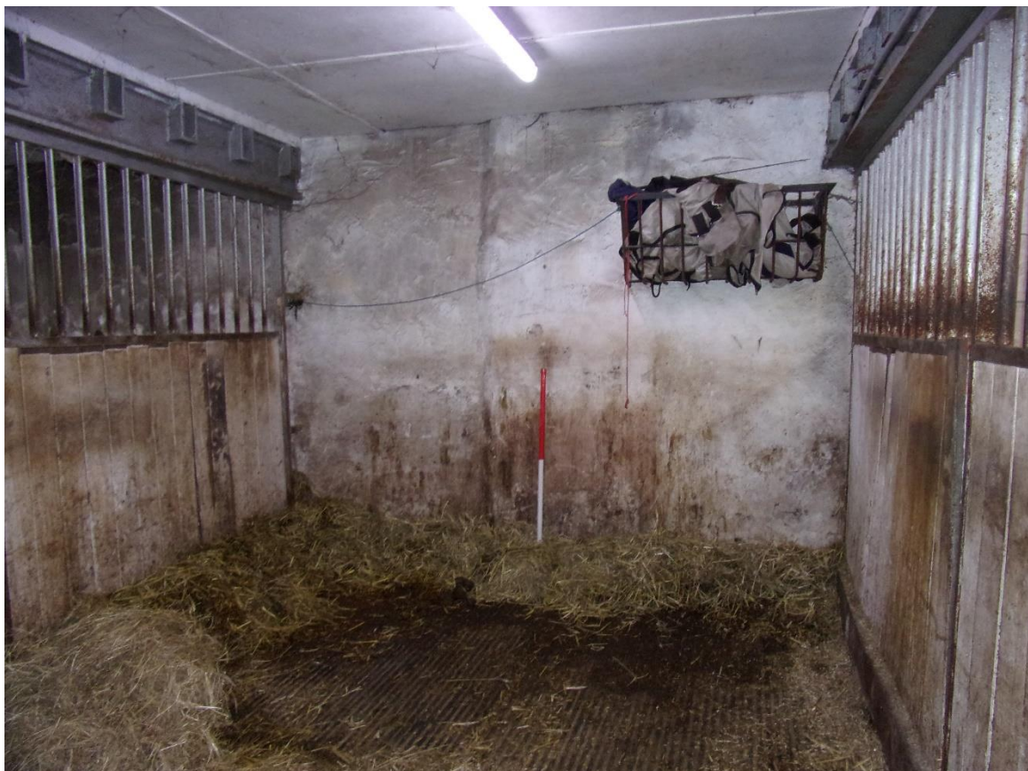
Plate 49 Room 8 facing west
