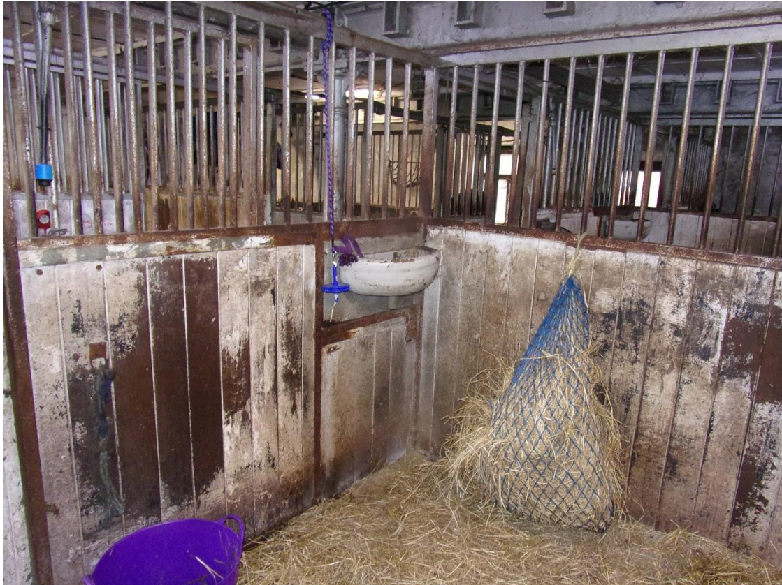
Plate 48 Room 7 facing southeast
