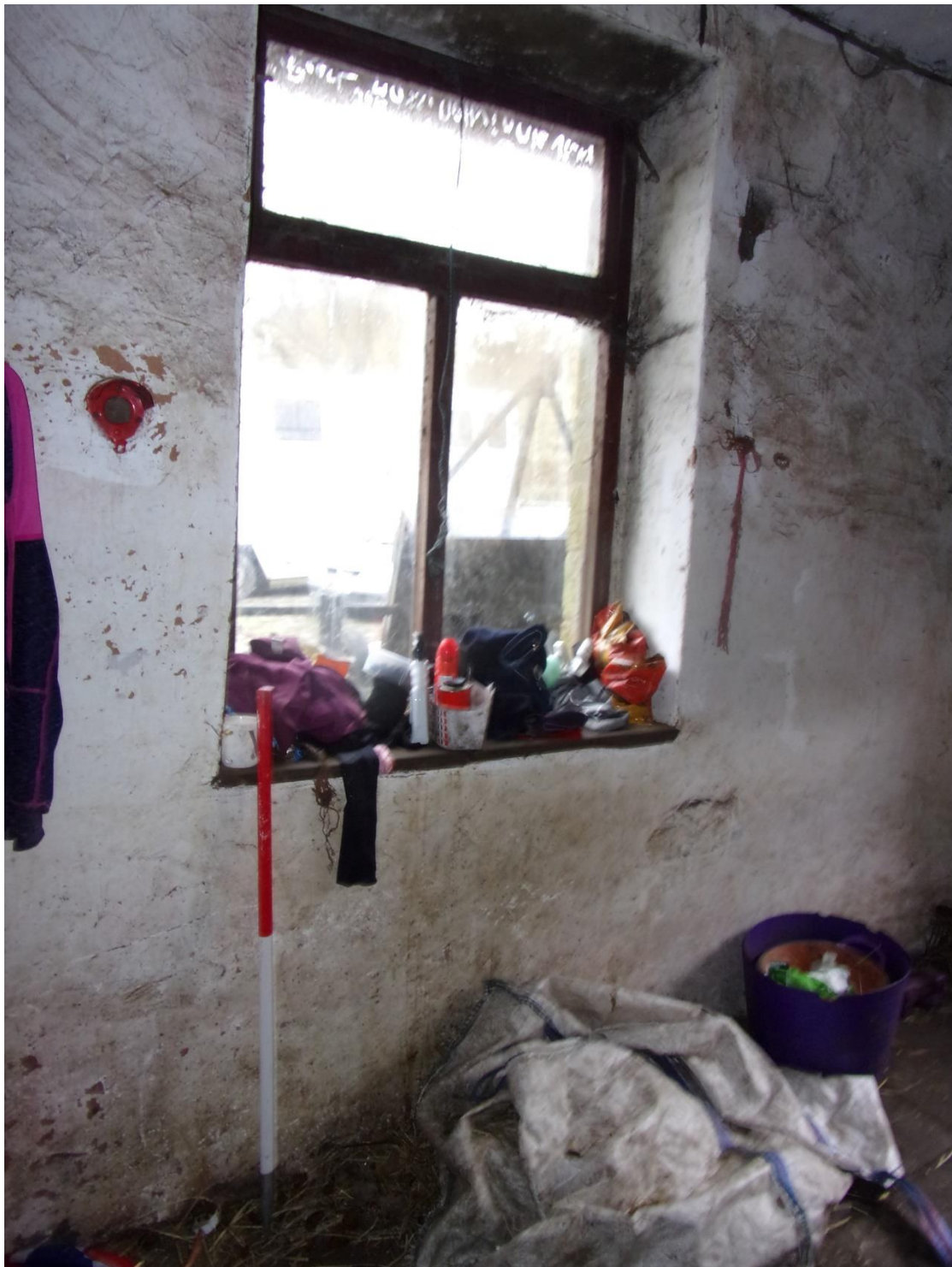
Plate 57 West internal elevation of Room 12, facing northwest
