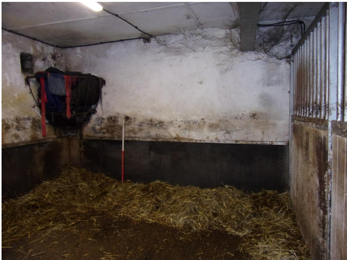
Plate 38 Room 4 facing east
