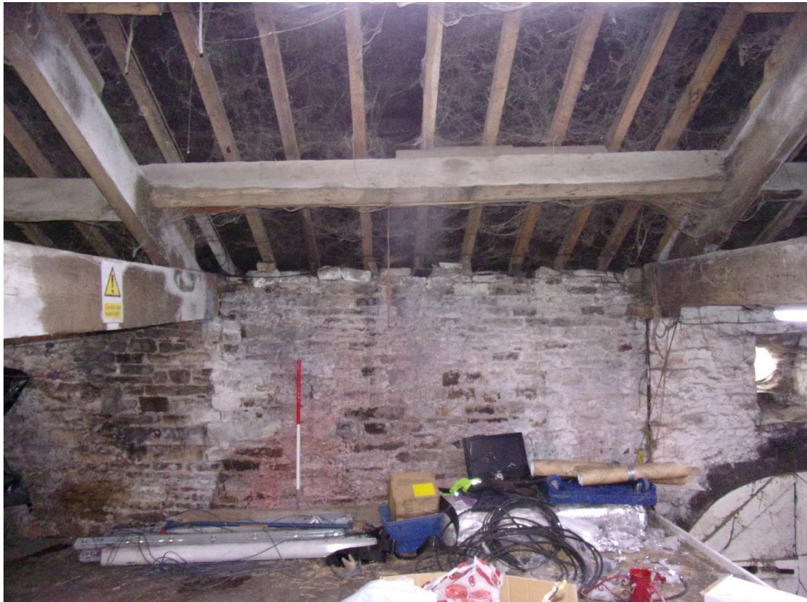
Plate 61 North elevation of Room 13 facing north
