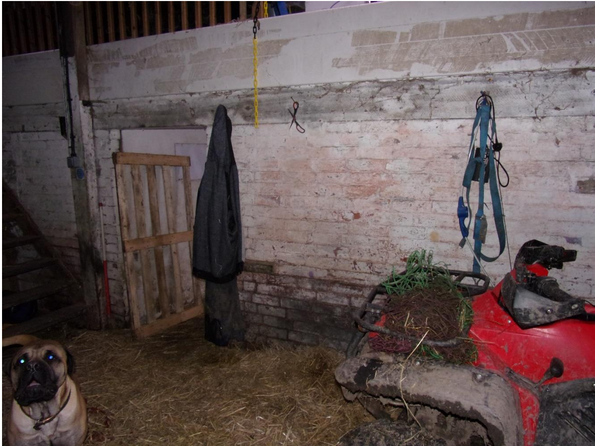
Plate 28 Partition wall in Room 1, facing southwest
