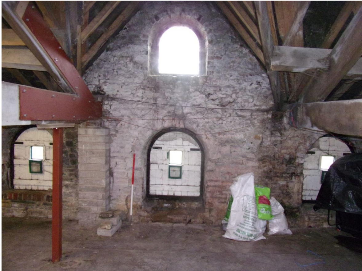
Plate 59 North internal elevation showing round headed arched windows
