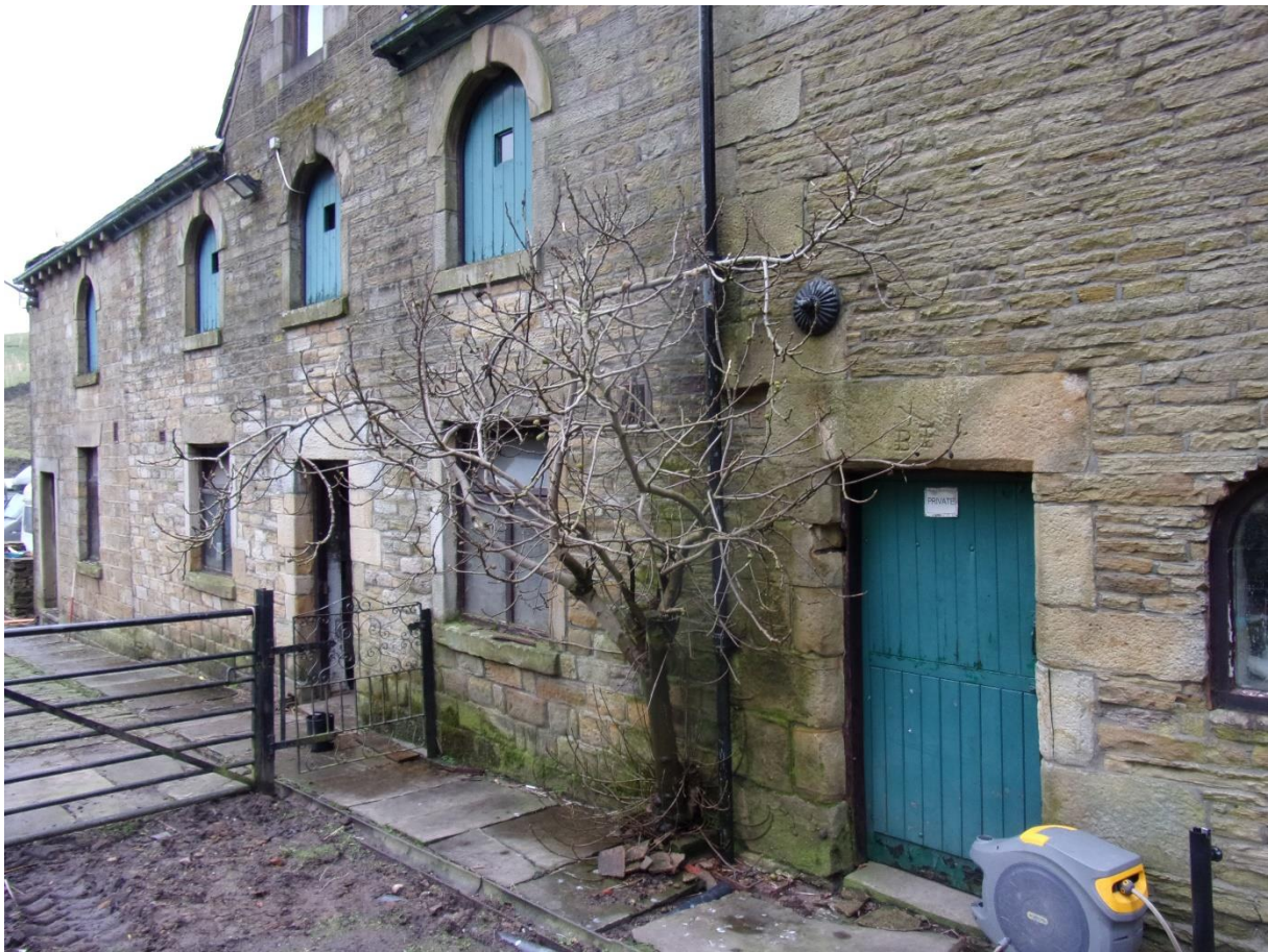
Plate 17 Stone quoins between the barn and the stable, facing northwest
