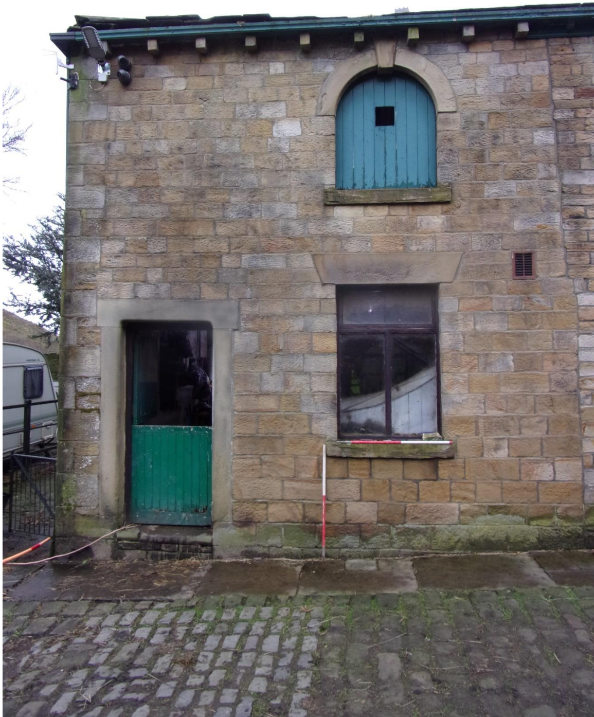
Plate 12 South elevation of the west stable, facing north. Clear join in the stonework can be observed.
