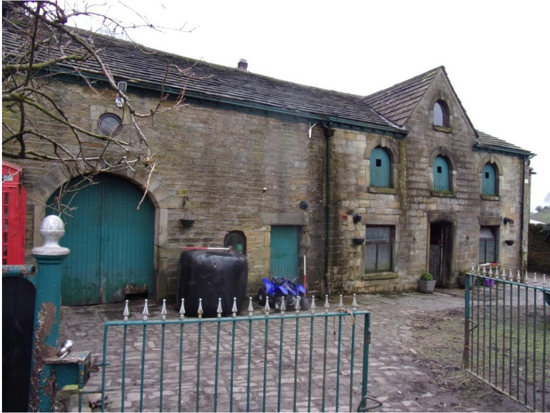
Plate 1 North elevation facing southeast
