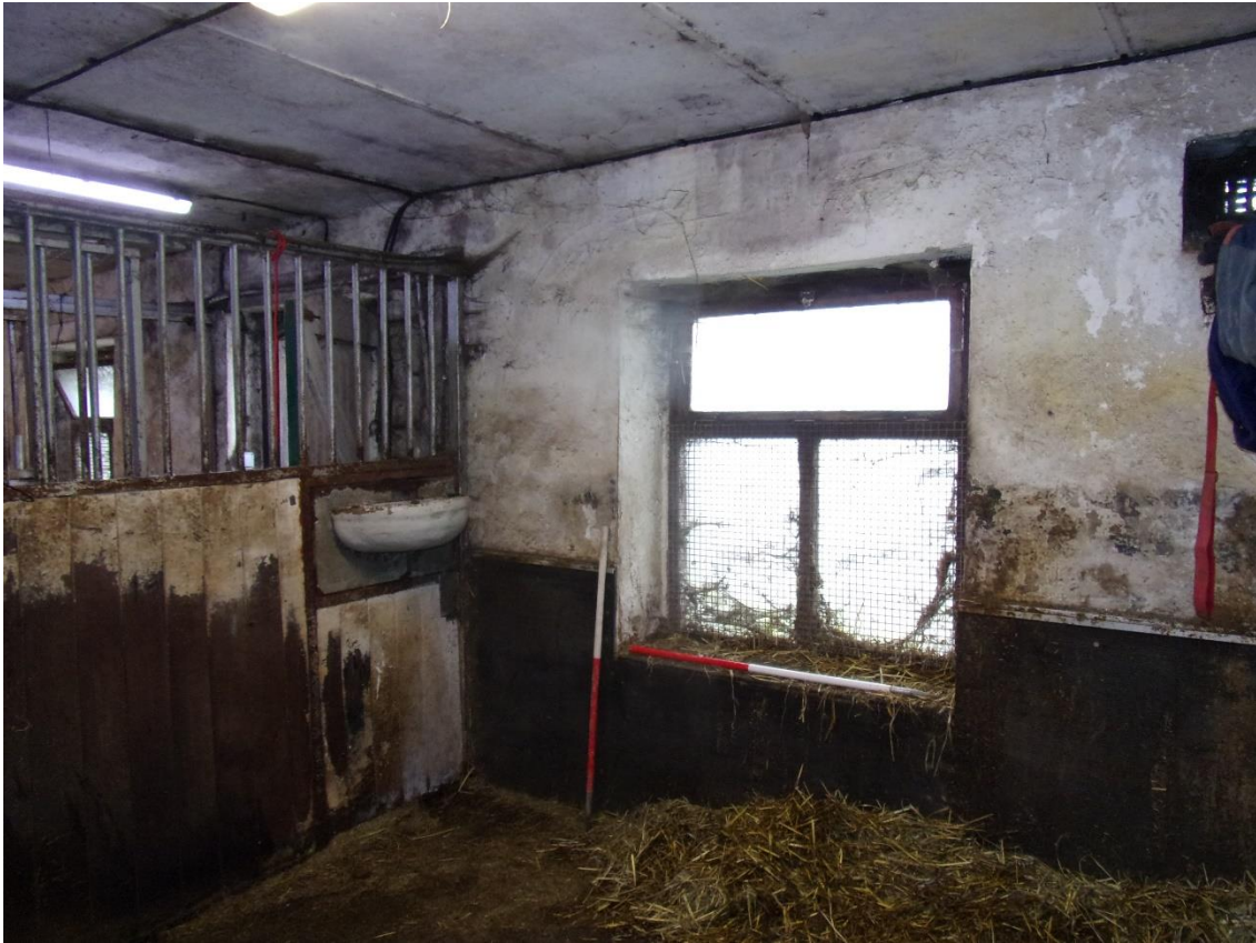
Plate 37 Room 4 facing northwest
