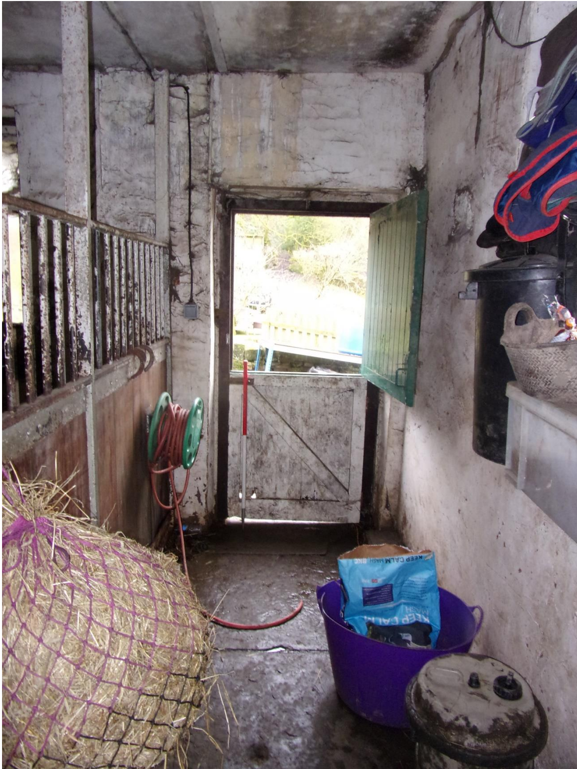
Plate 56 South elevation of Room 12, facing south
