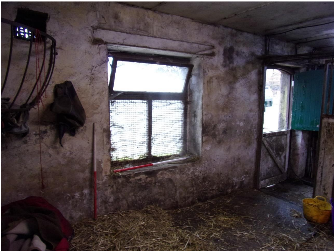
Plate 47 Room 7 facing northeast
