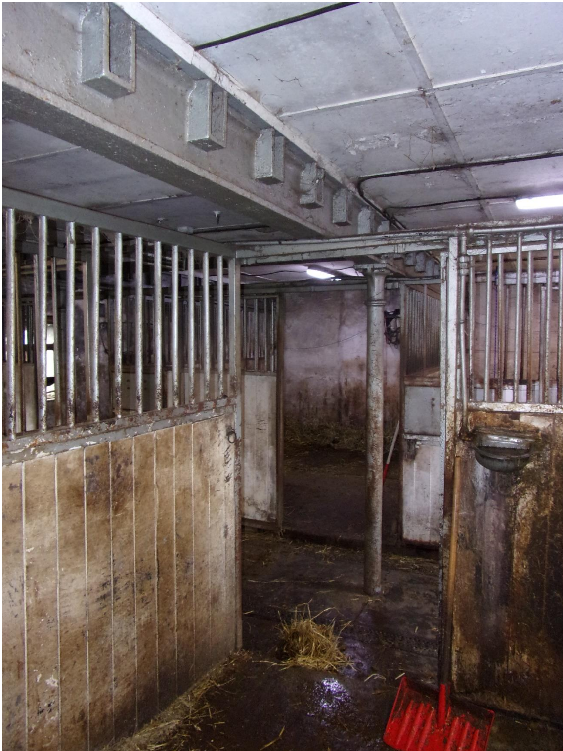
Plate 41 Room 5 facing west
