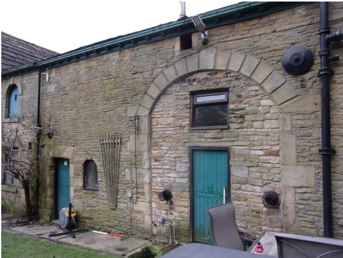
Plate 15 Blocked wagon door in the south elevation, facing northwest
