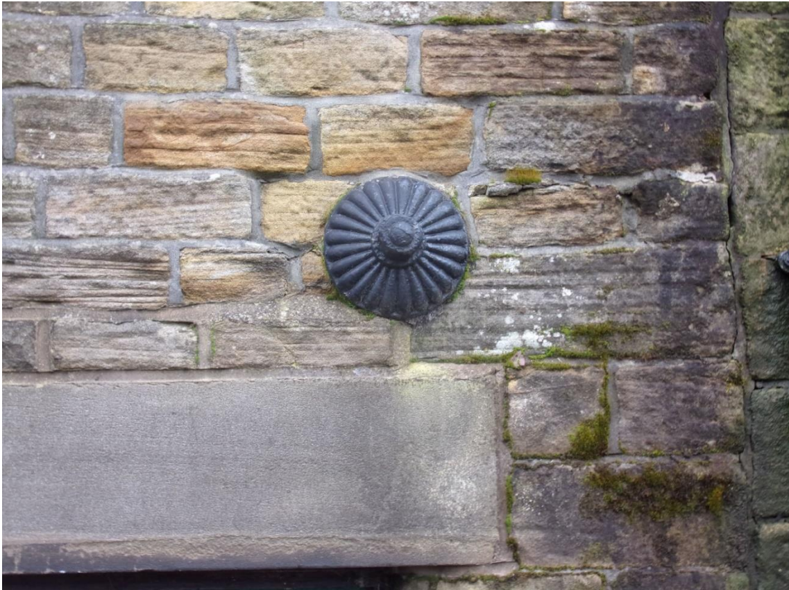
Plate 9 Cast iron wallplate above the doorway in the north elevation
