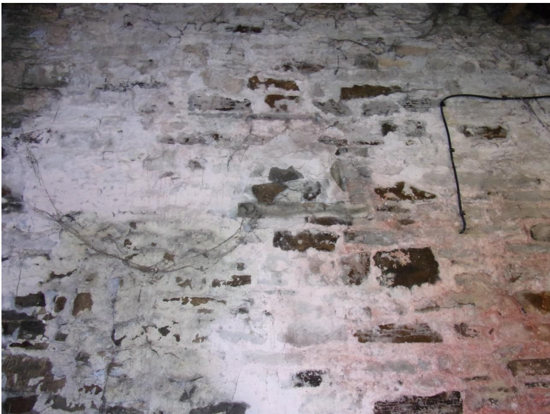
Plate 74 Possible blocked aperture in the west elevation of Room 13, facing west
