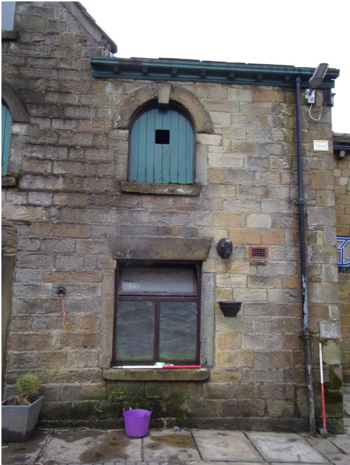
Plate 6 North elevation facing south
