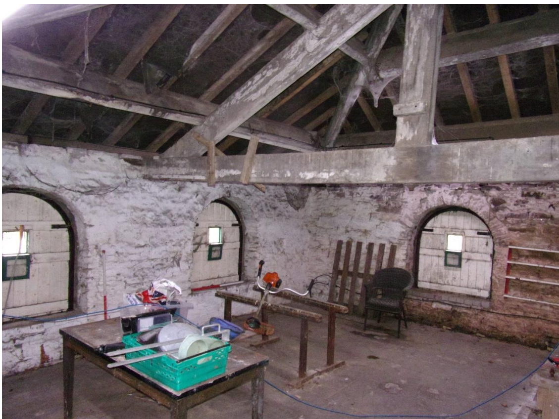
Plate 78 Room 14 facing southwest
