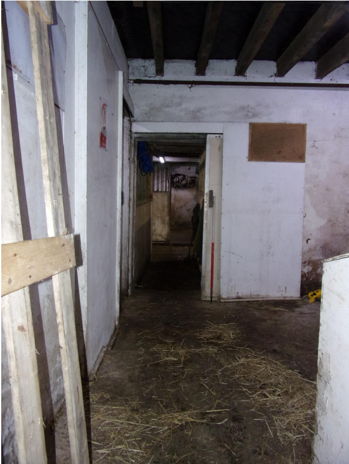
Plate 35 Room 2 facing west
