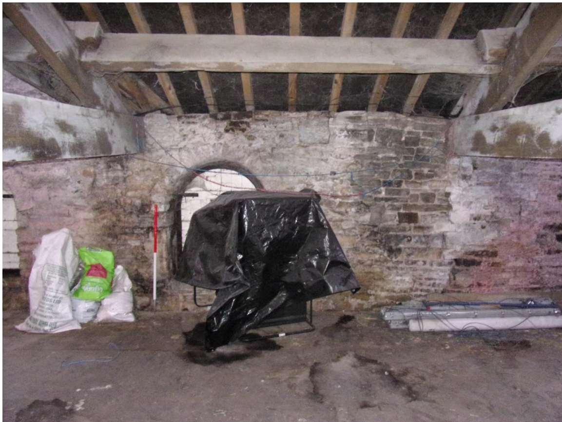
Plate 62 North elevation of Room 13, facing north
