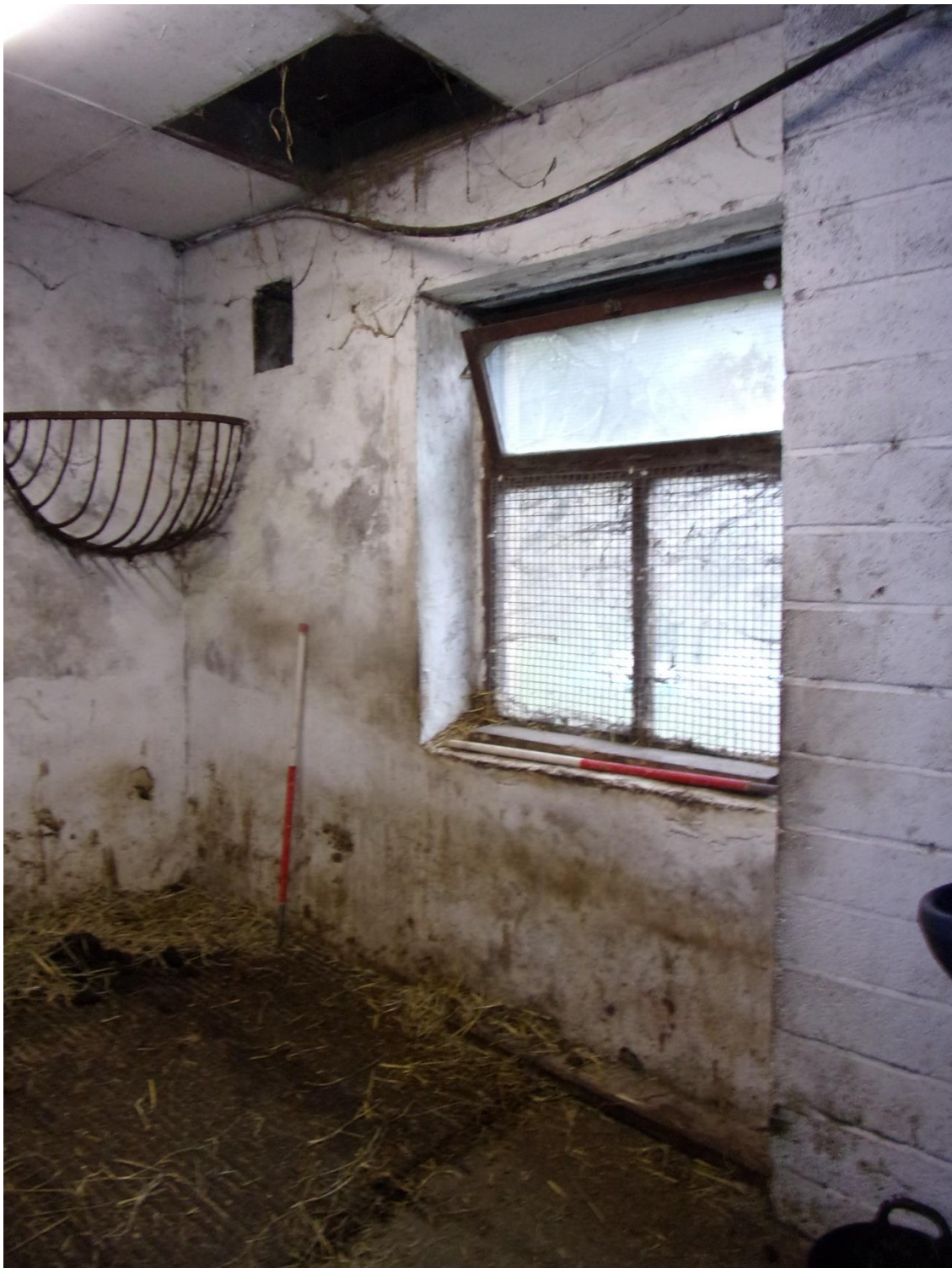
Plate 51 Room 9 facing southeast
