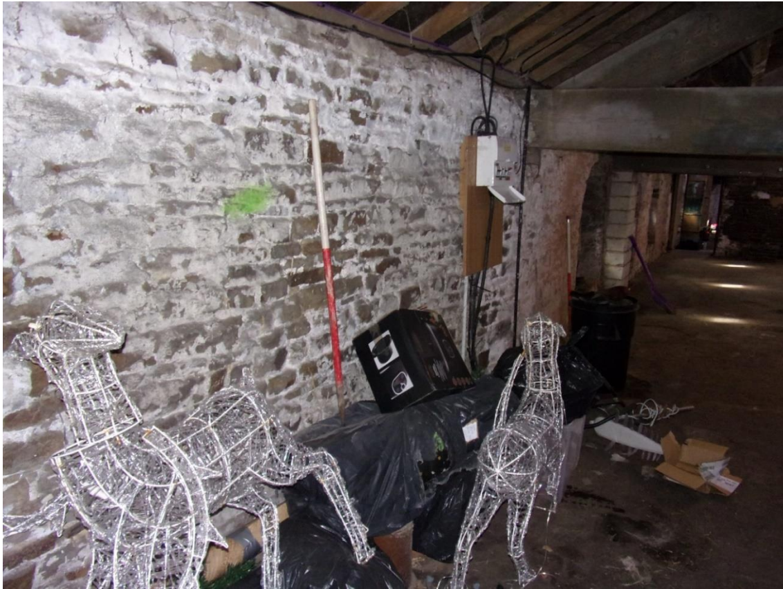
Plate 64 South internal elevation facing southwest
