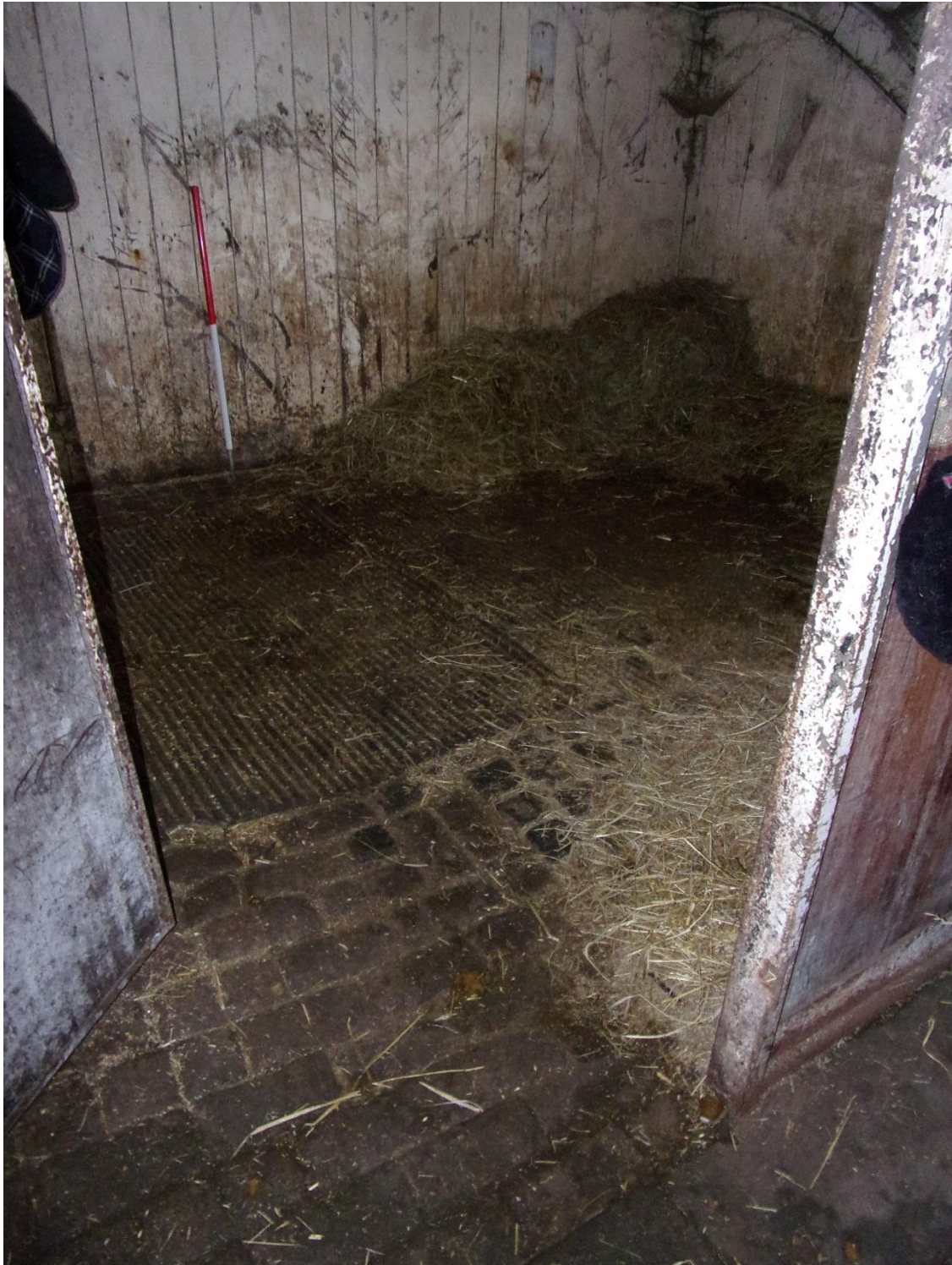
Plate 55 Floor in Room 11, facing southeast
