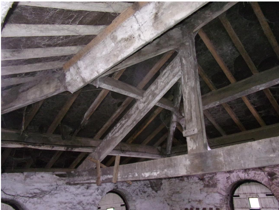
Plate 80 Roof structure of the west stables
