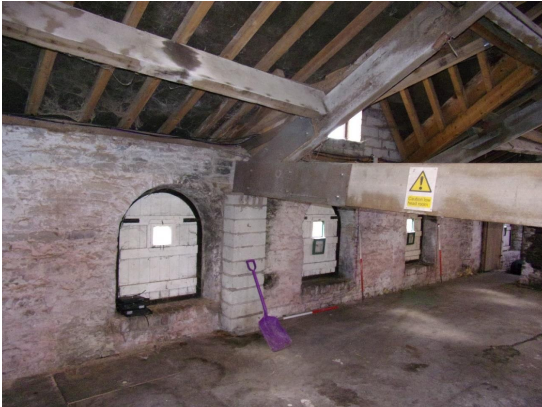
Plate 66 South internal elevation of Room 13 facing southwest
