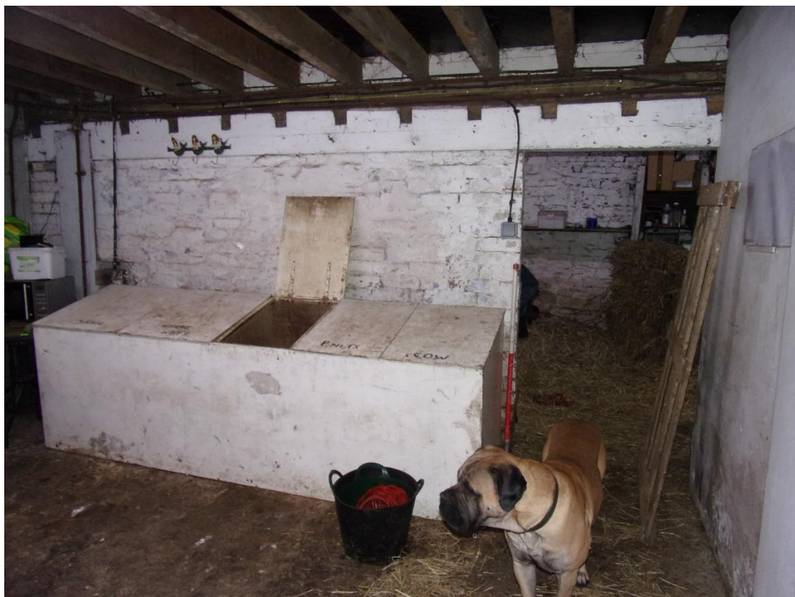
Plate 32 East internal elevation of Room 2, facing northeast
