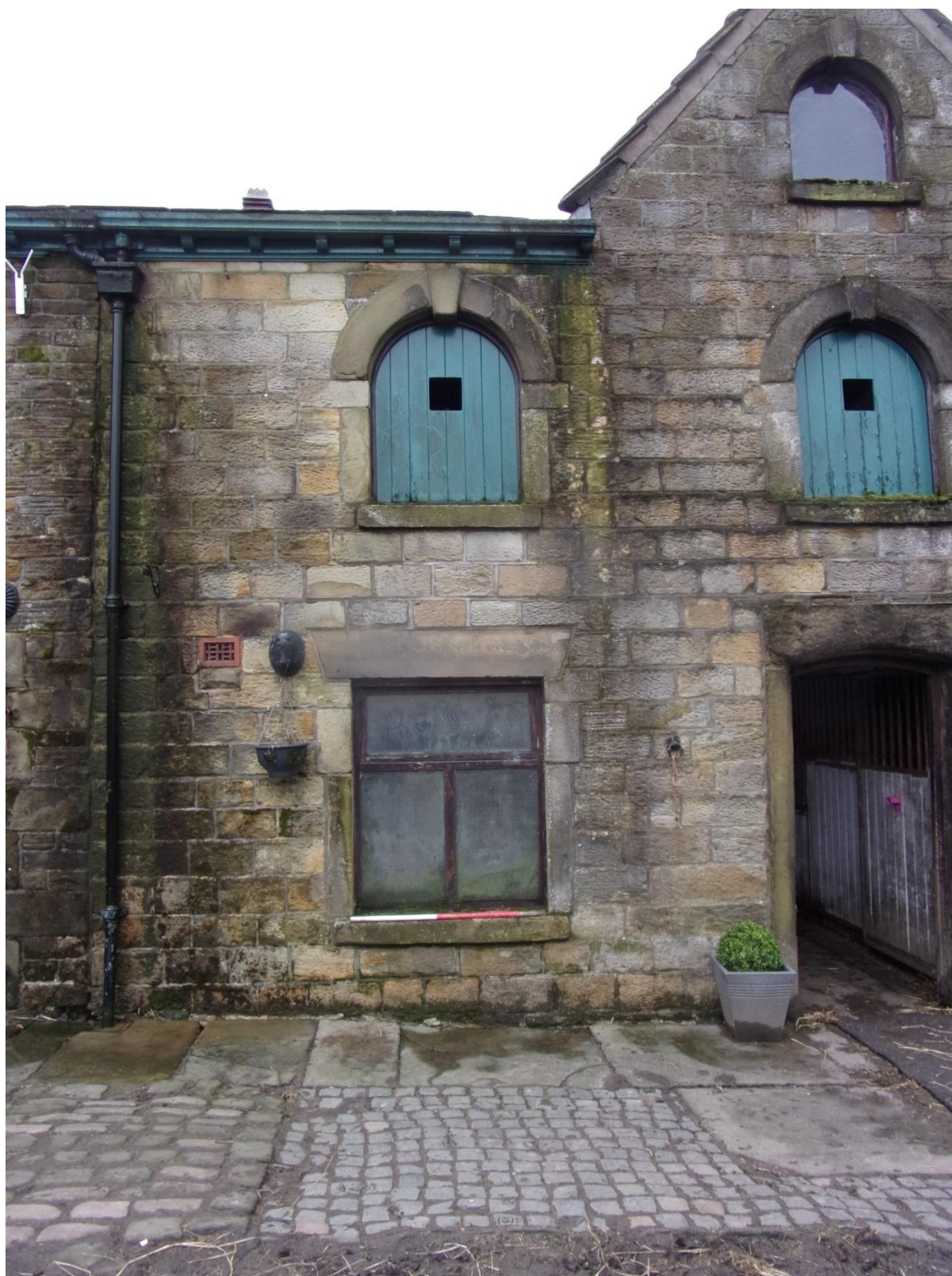
Plate 7 Remodelled central part of the north elevation, facing south
