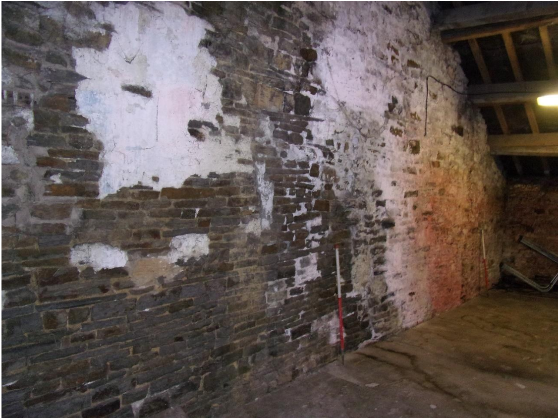
Plate 73 Partition wall between Rooms 13 and 14, facing northwest
