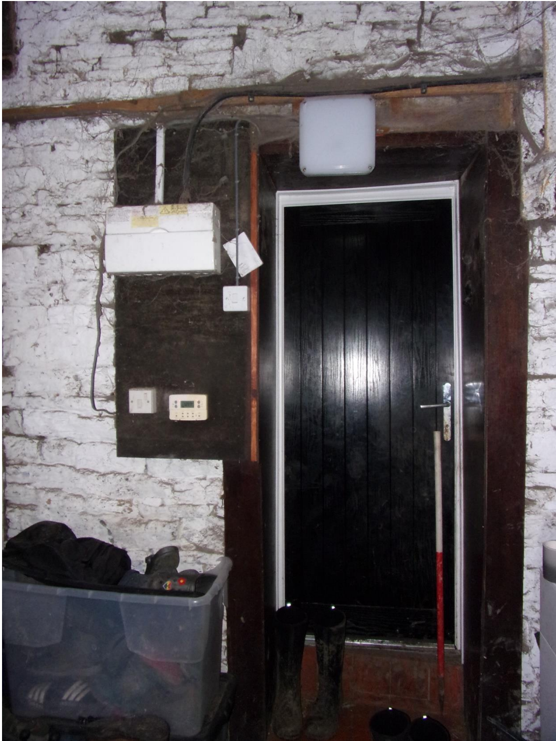
Plate 27 Modern doorway to the farmhouse in the east elevation
