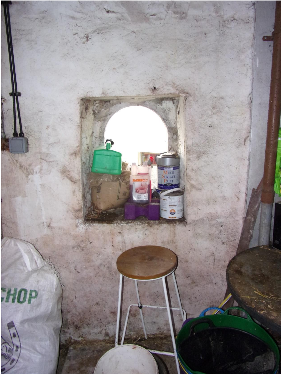
Plate 34 Window in the north elevation of Room 2
