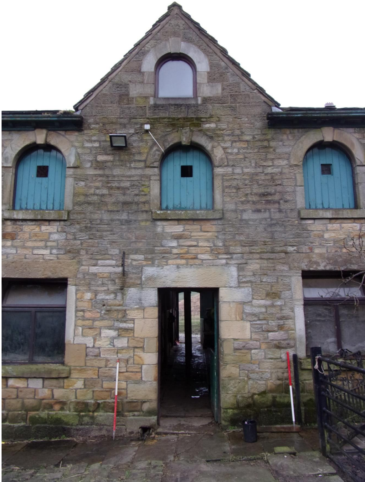
Plate 14 Central remodelled part of the south elevation facing north. The gable is a later, probably 1980s addition.
