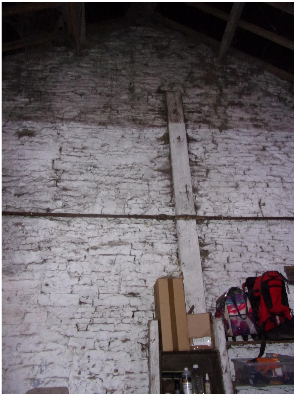
Plate 25 East internal elevation of Room 1
