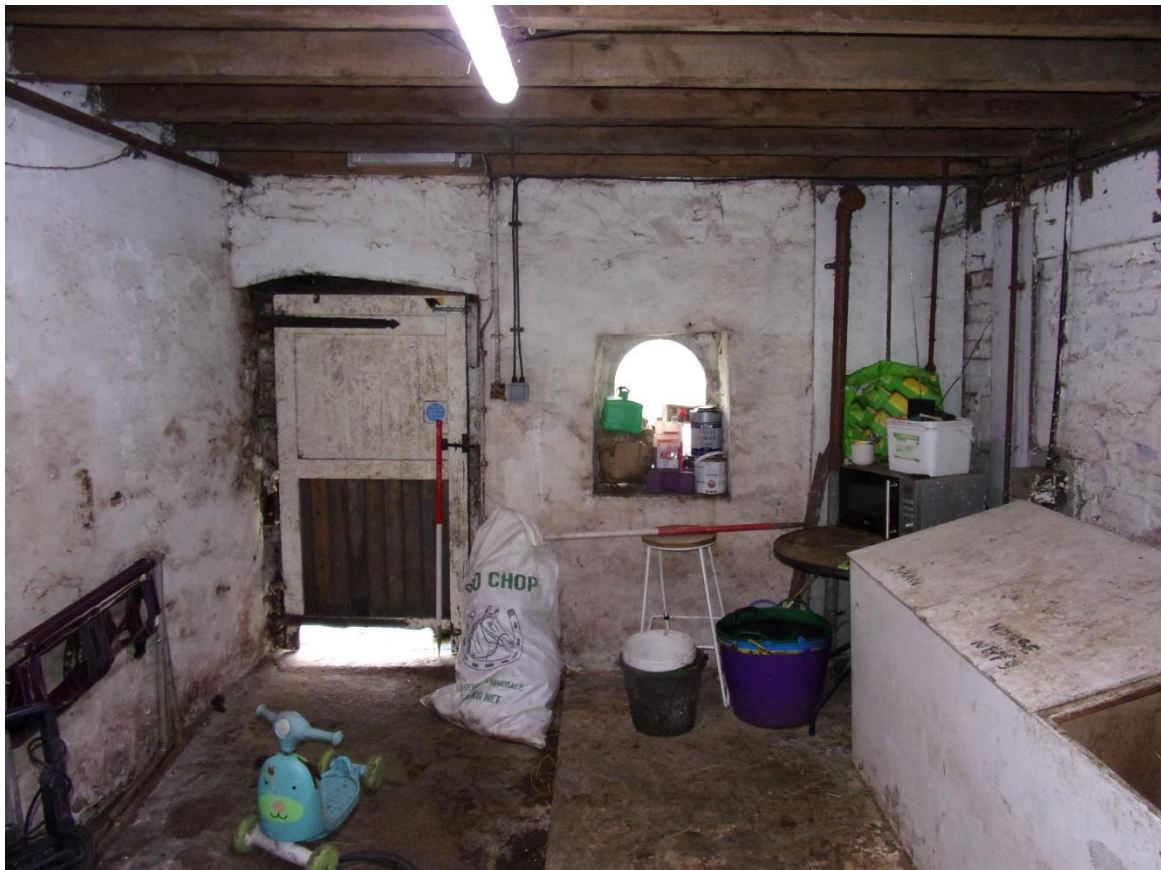
Plate 31 North internal elevation of Room 2, facing north
