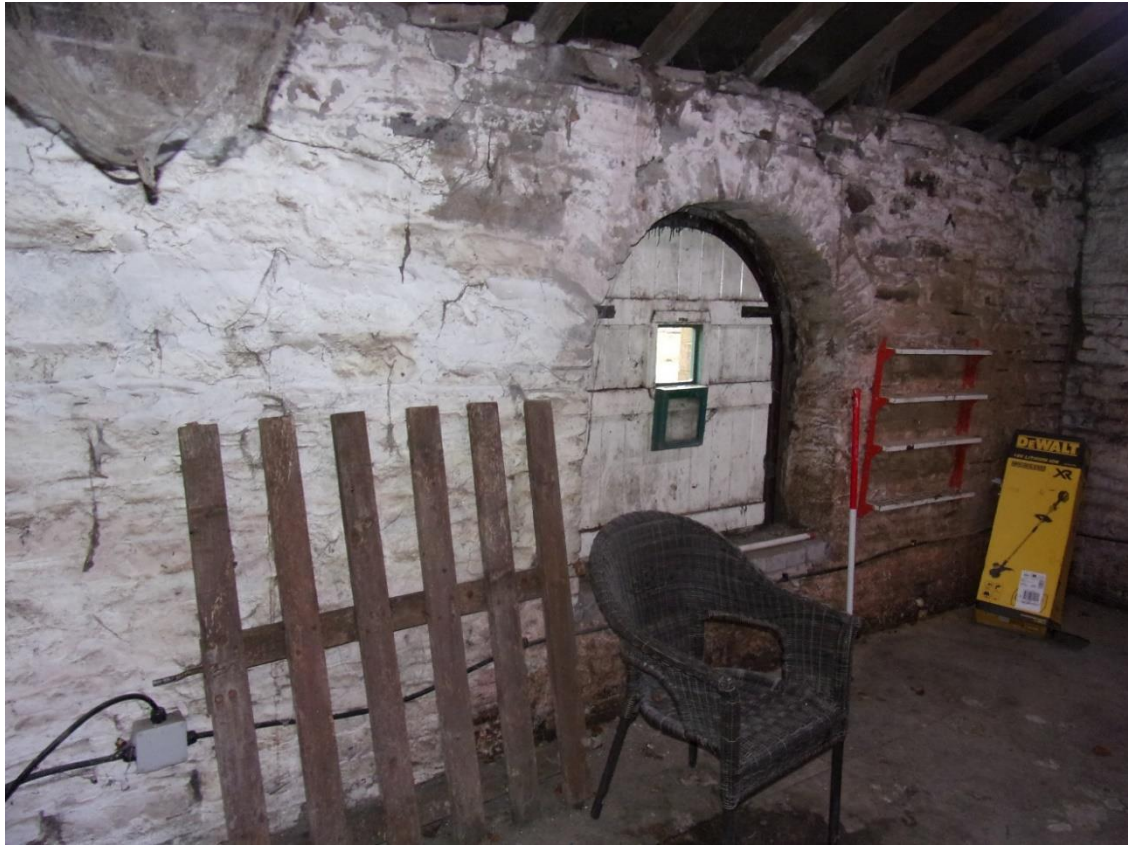
Plate 79 North elevation of Room 14, facing northeast
