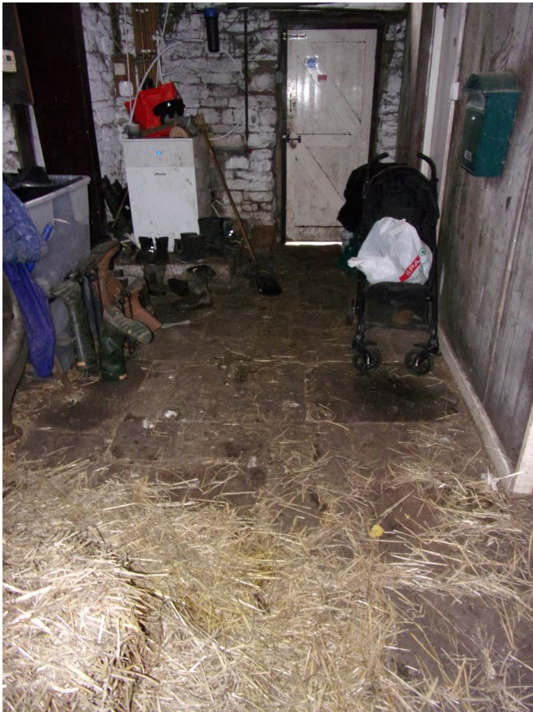
Plate 24 South internal elevation of Room 1
