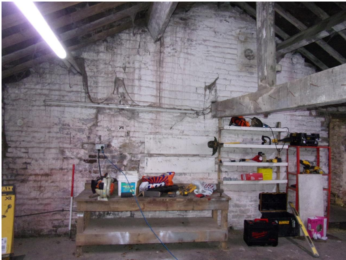
Plate 75 East elevation in Room 14, facing southeast
