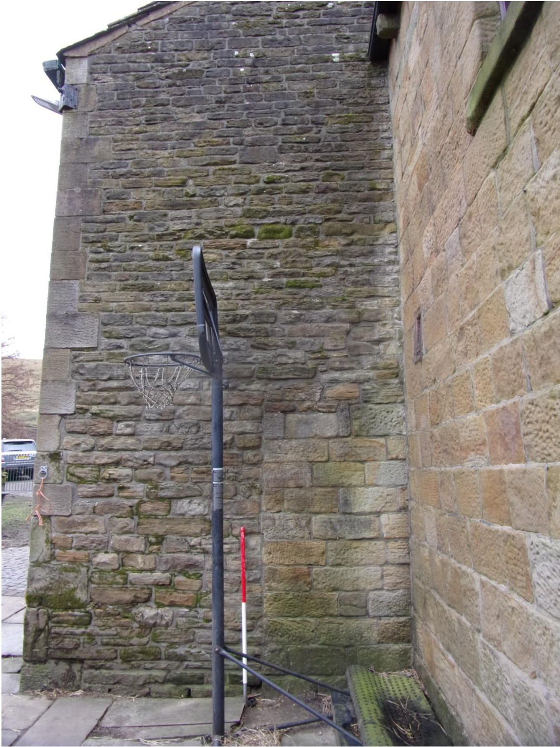
Plate 5 Blocked aperture in the east elevation of the barn
