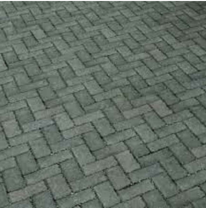
M3 Driveway / Access Road Surface
