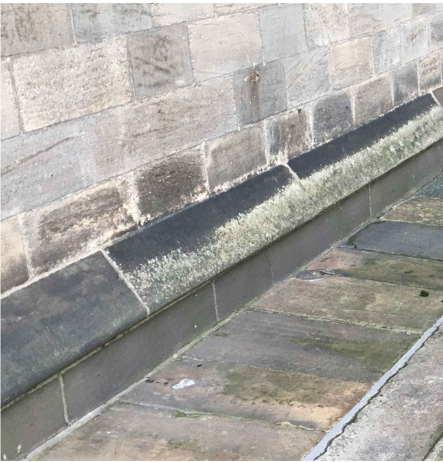
Original plinth replicated
