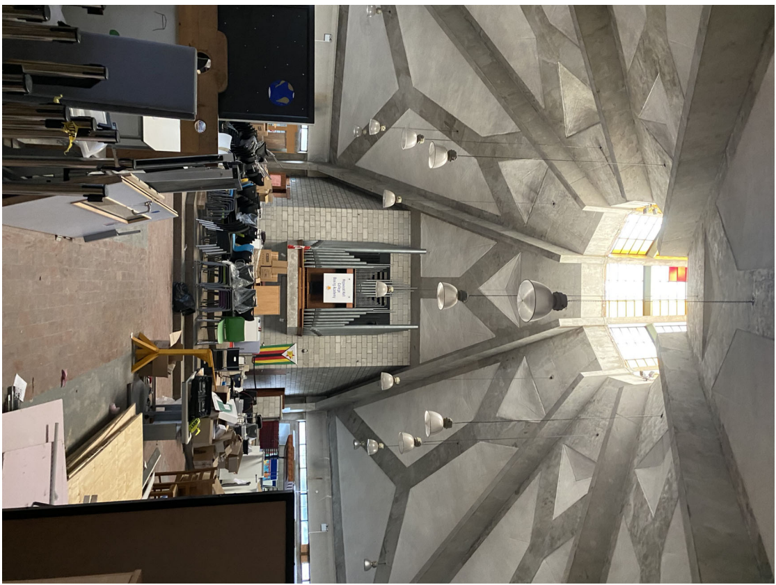
Interior Views showing asbestos soffits and high level wall panels
